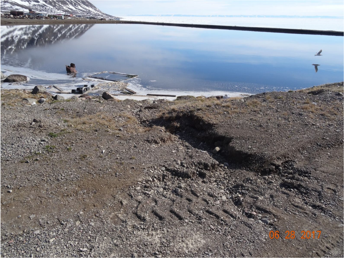
Figure 2: SDF infiltration and erosion
