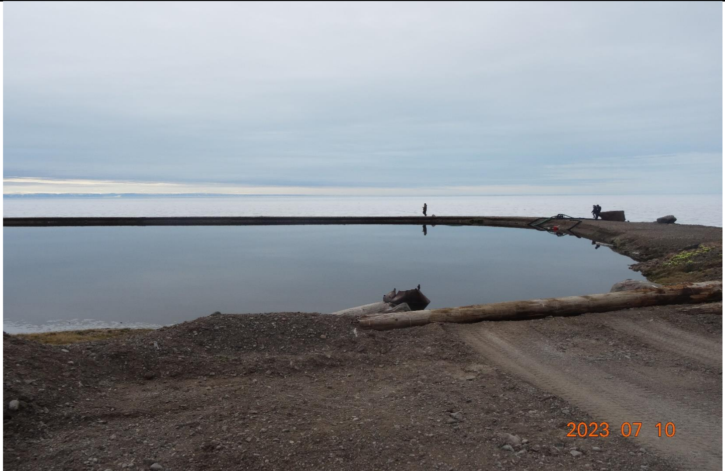
Description: The sewage lagoon Freeboard less than 1 metre
