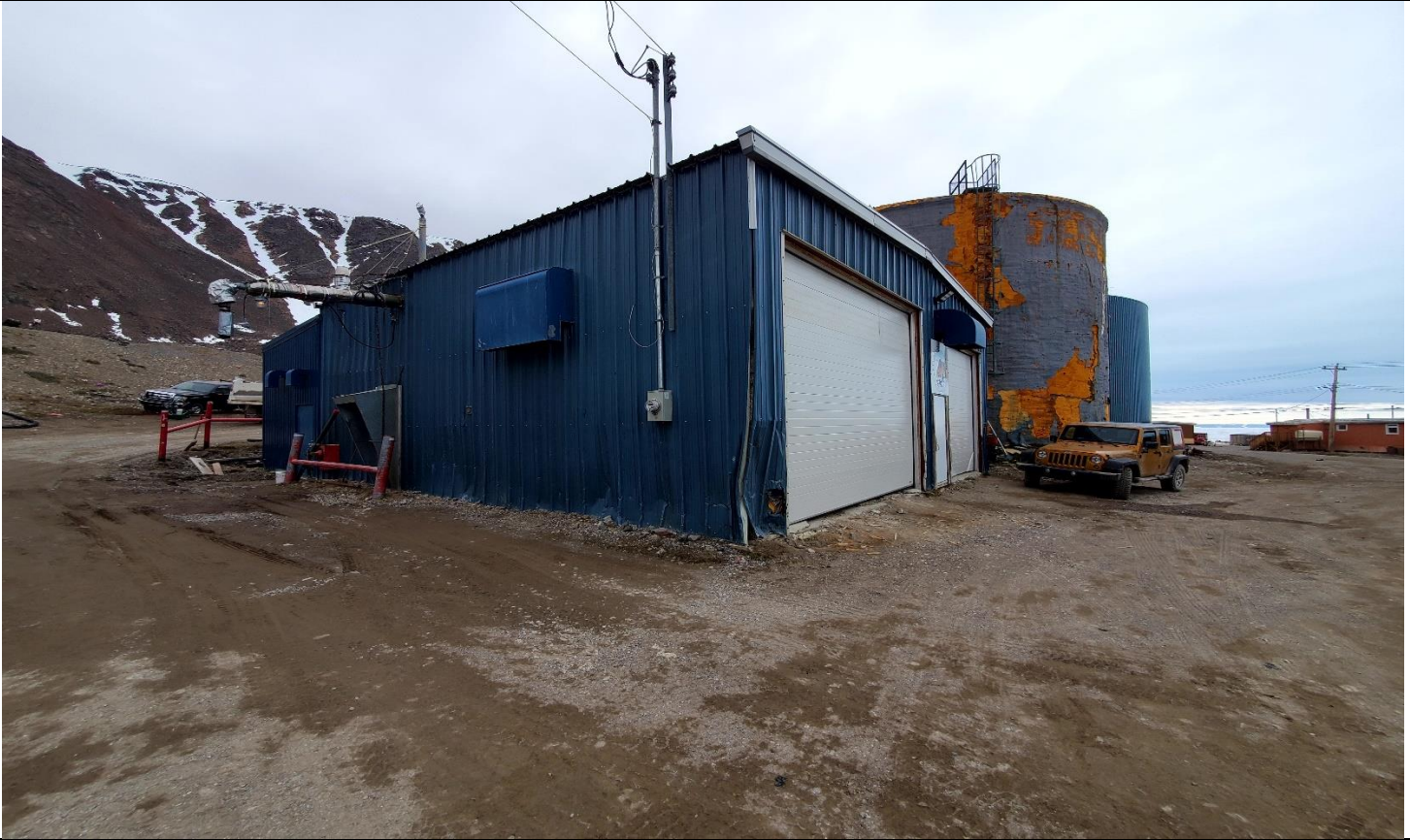
Description: 3x Water Storage Tanks. 1 of 3 Water Storage Tanks damaged, and decommissioned. Truck refill station.
