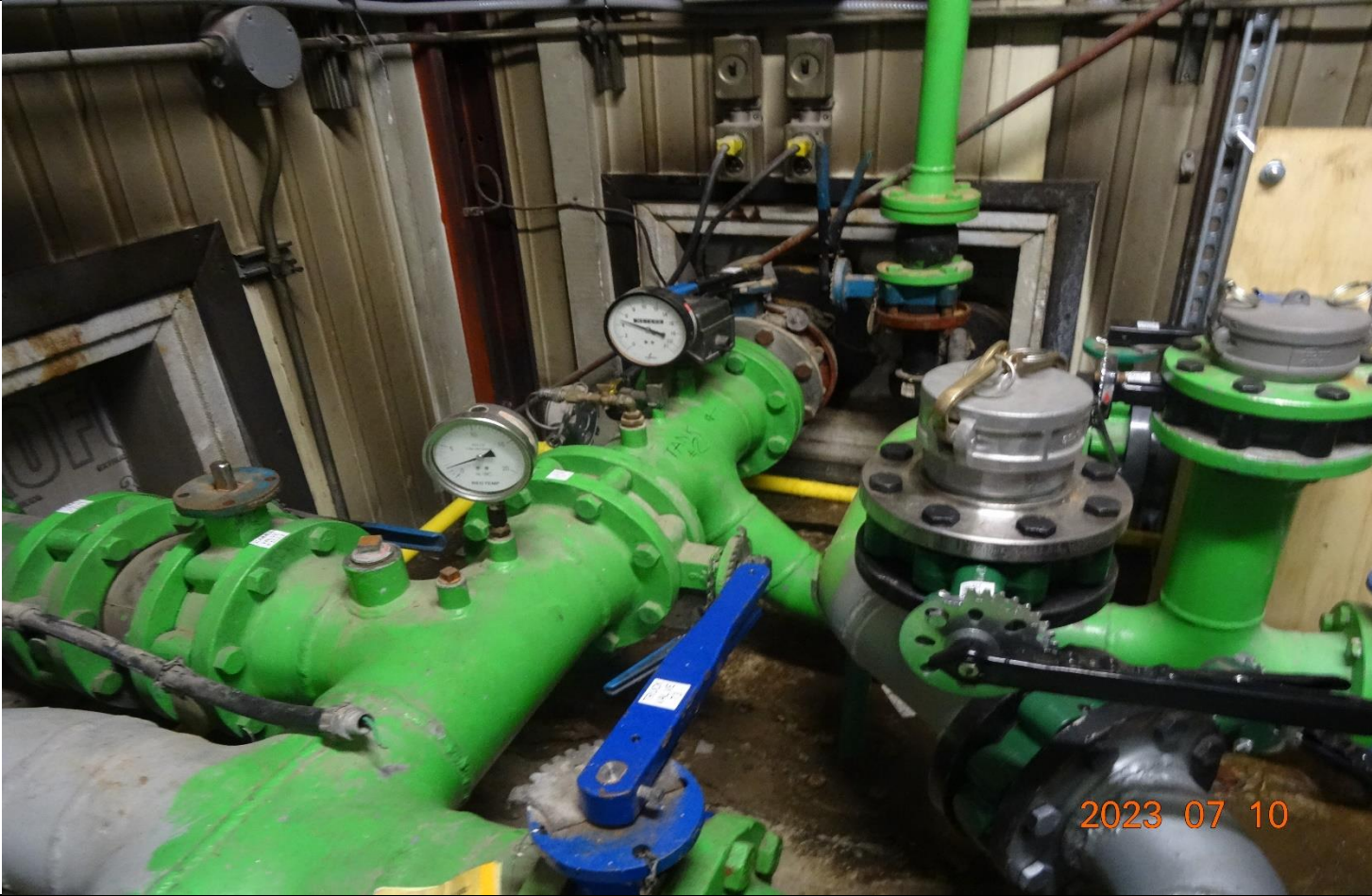
Description: Internal piping to distribute water to the 3 different water storage tanks. Water comes in from the reservoir on the left, and is distributed to the two working water storage tanks.
