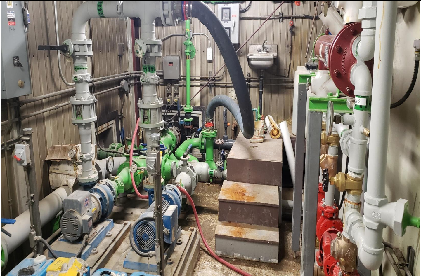
Description: Internal piping to distribute water to the 3 different water storage tanks.
