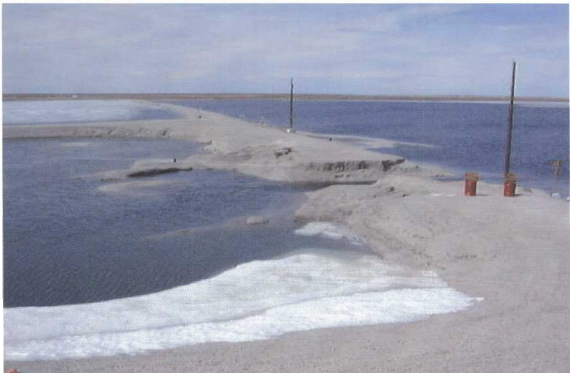
figure 3. Breached berm along the northern face of the 'inner' lake; 2001/07/12.
