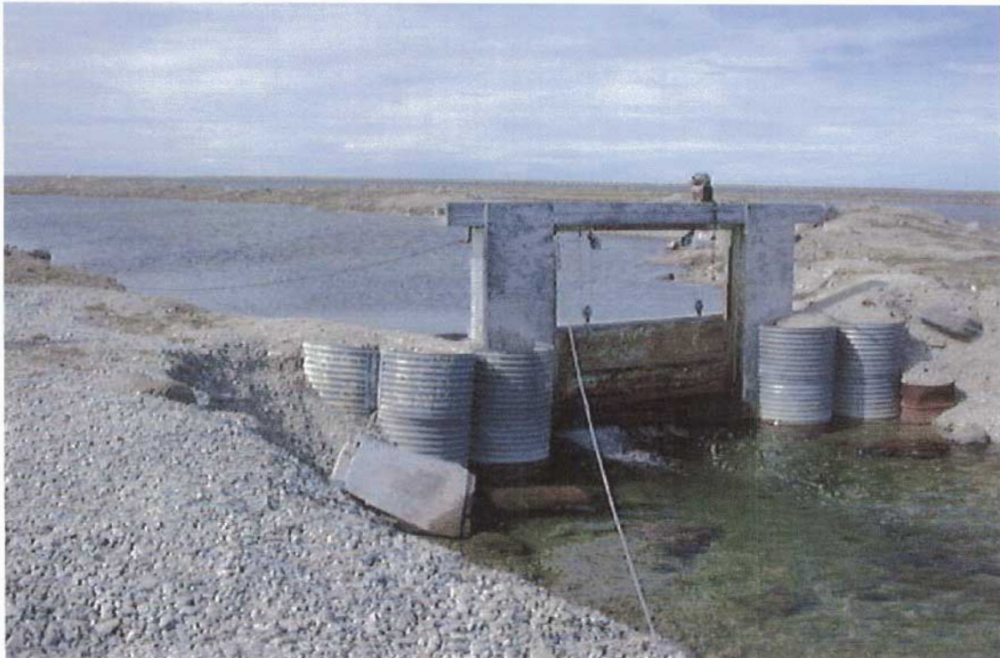
figure 1. Decant station at outlet of Water Lake; 2001/07/12.
