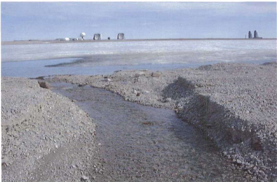
figure 2. Breached berm along western face of the 'outer' lake; 2001/07/12.
