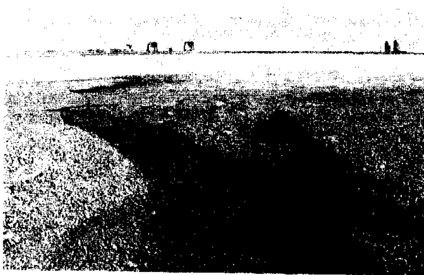
figure 2. Breached berm along western face of the 'ouner' lake; 2001/07/12.
