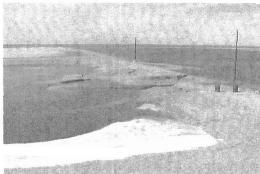
figure 3. Breachd berm along the northern face of the 'inner' lake; 2001/07/12.
