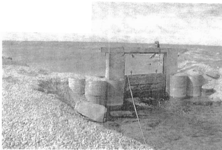
figure 1. Decant station at outlet of Water Lake; 2001/07/12
