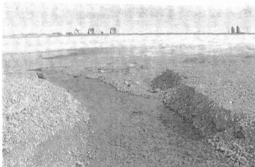
figure 2. Breachd berm along western face of the 'outer' lake; 2001/07/12.
