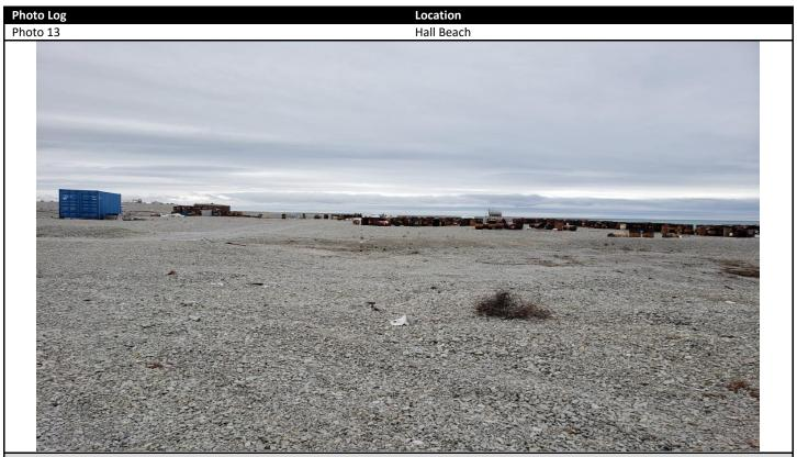
Description: Hazardous Waste Section of the Solid Waste Facility. Non-engineered walls prevent water from entering and mixing with Hazardous waste.
