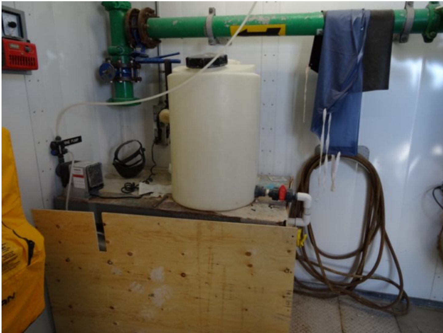
Figure 5 Chlorination mixing and pumping station in Pump House
