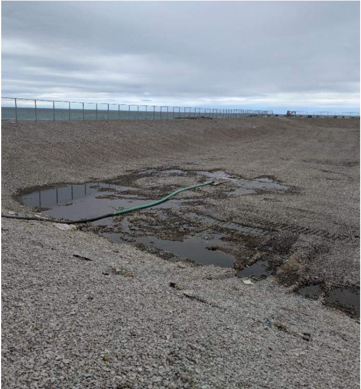
Photograph #3: Water pooling into the northeast corner of the south cell.
