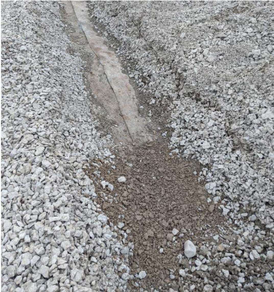
Photograph #2: Seams were covered in sand prior to being covered with the aggregates.
