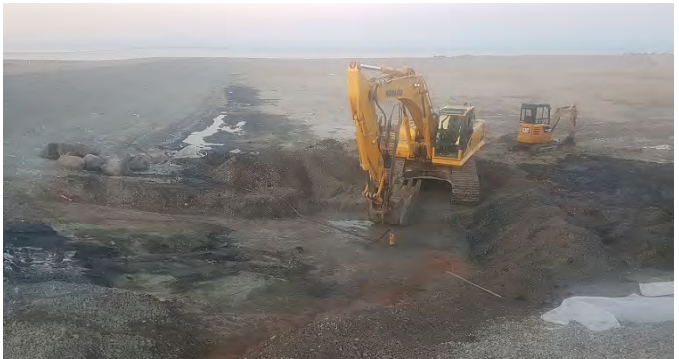
Photo 4: Water pumped from the bottom of the exposed area. Bentonite placed on the GCL seam and closed.
