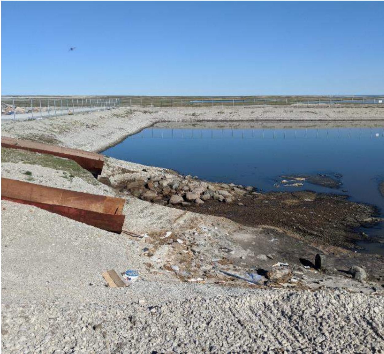
Photograph #4: The north cell's water level has dropped significantly. This picture was taken July 24 th , 13 days after Photograph #3. The water level has dropped by about a meter.
