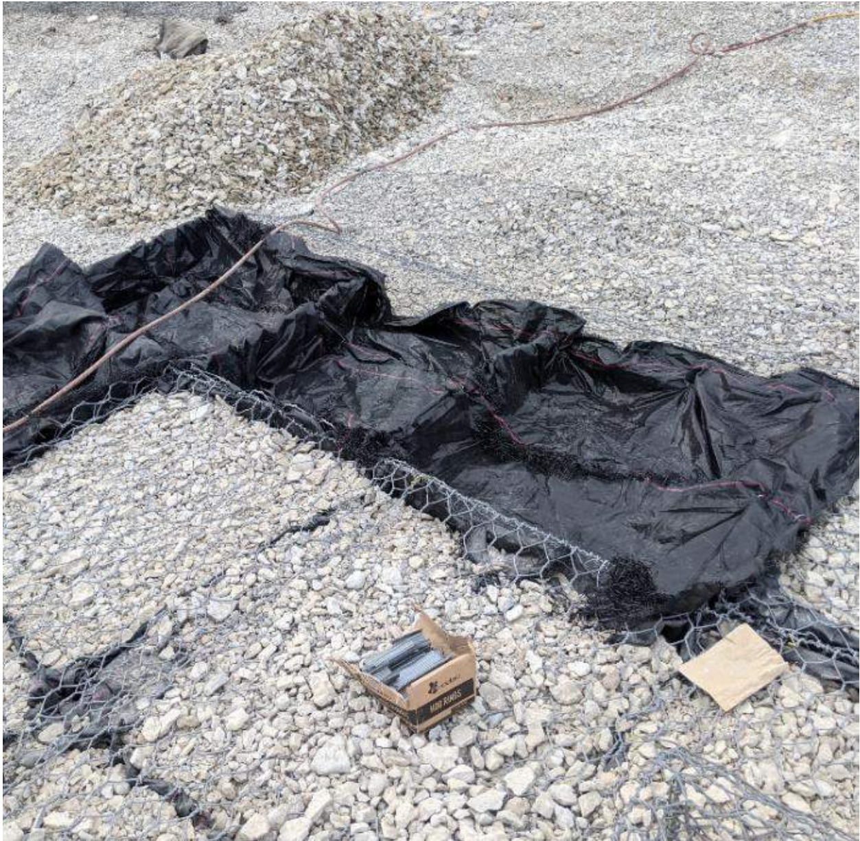
Photograph #1: Lined cages ready to be filled.
