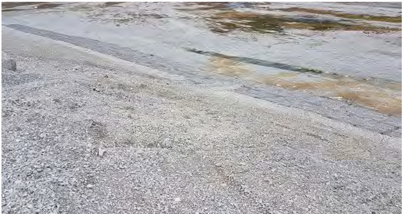
Photo 2: View of the eastern berm of Cell 1, where seepage has occurred.
