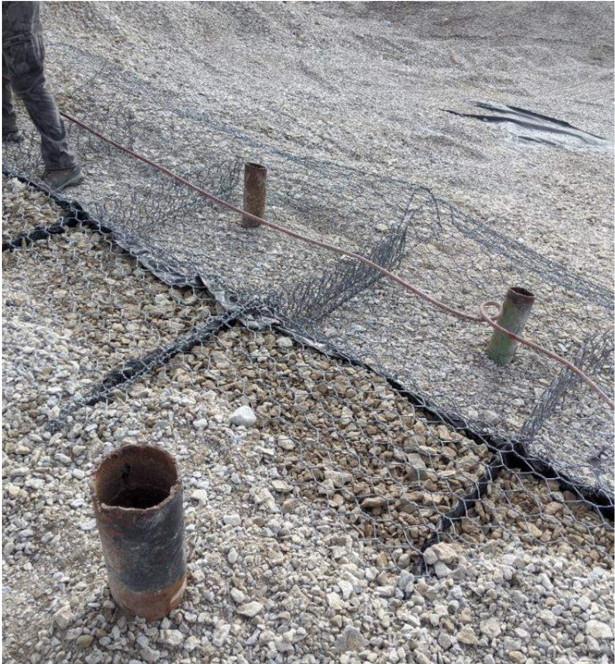
Photograph #1: Gabion cages installation at north discharge station.
