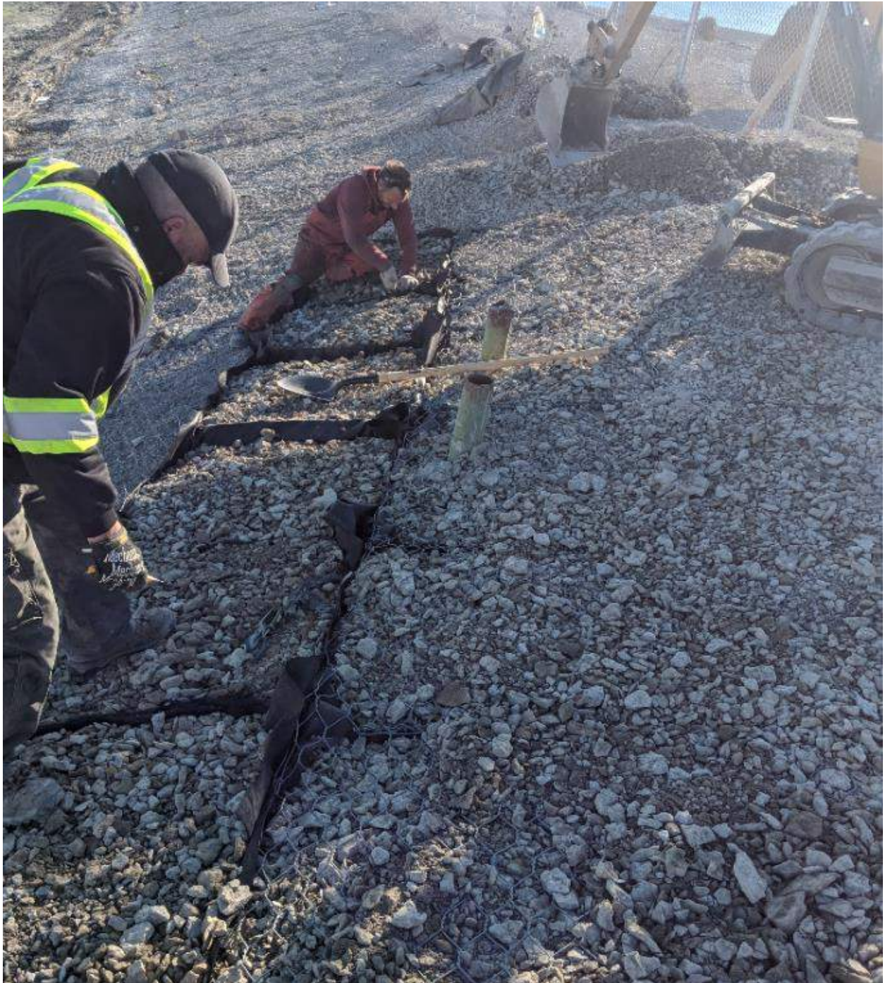
Photograph #1: The gabion cages, once filled, were wired shut as well as wired to the previous row of cages to form a complete mat.
