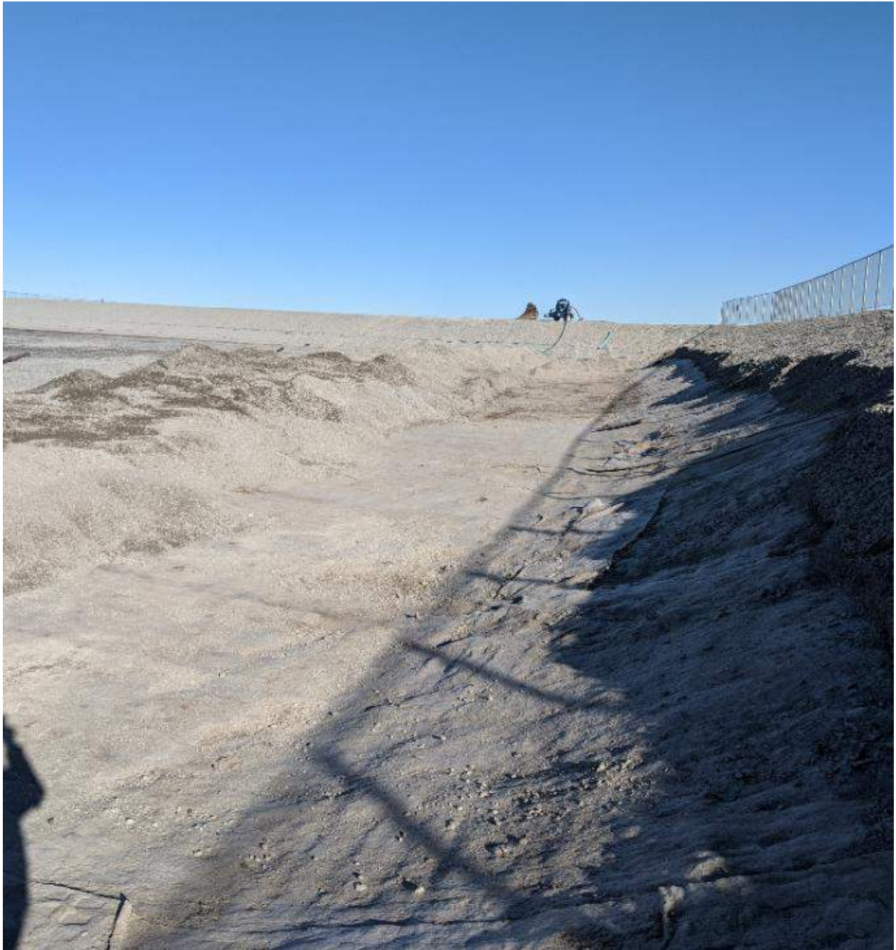
Photograph #1: The result. Existing liner exposed along the bottom of the lagoon. Some wrinkles and rolls present, which will be smoothed out prior to placing the new liner down.
