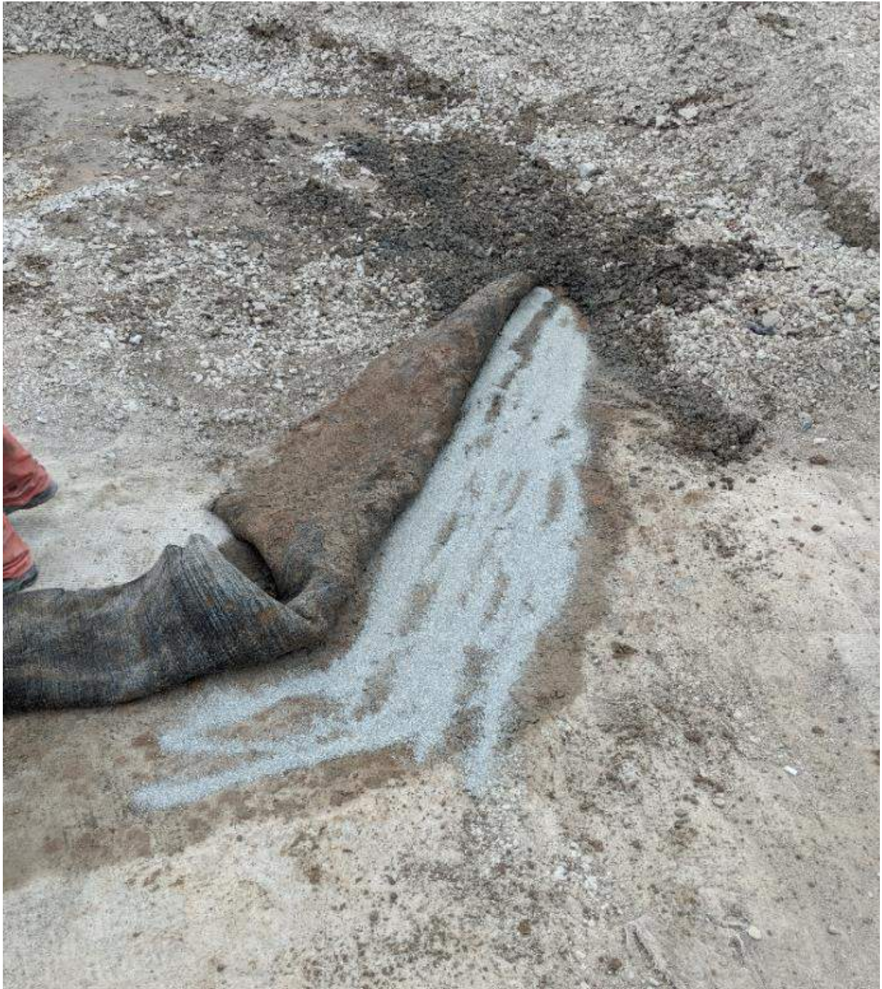
Photograph #1: Seams in existing liner were cleaned out and sealed with additional bentonite.
