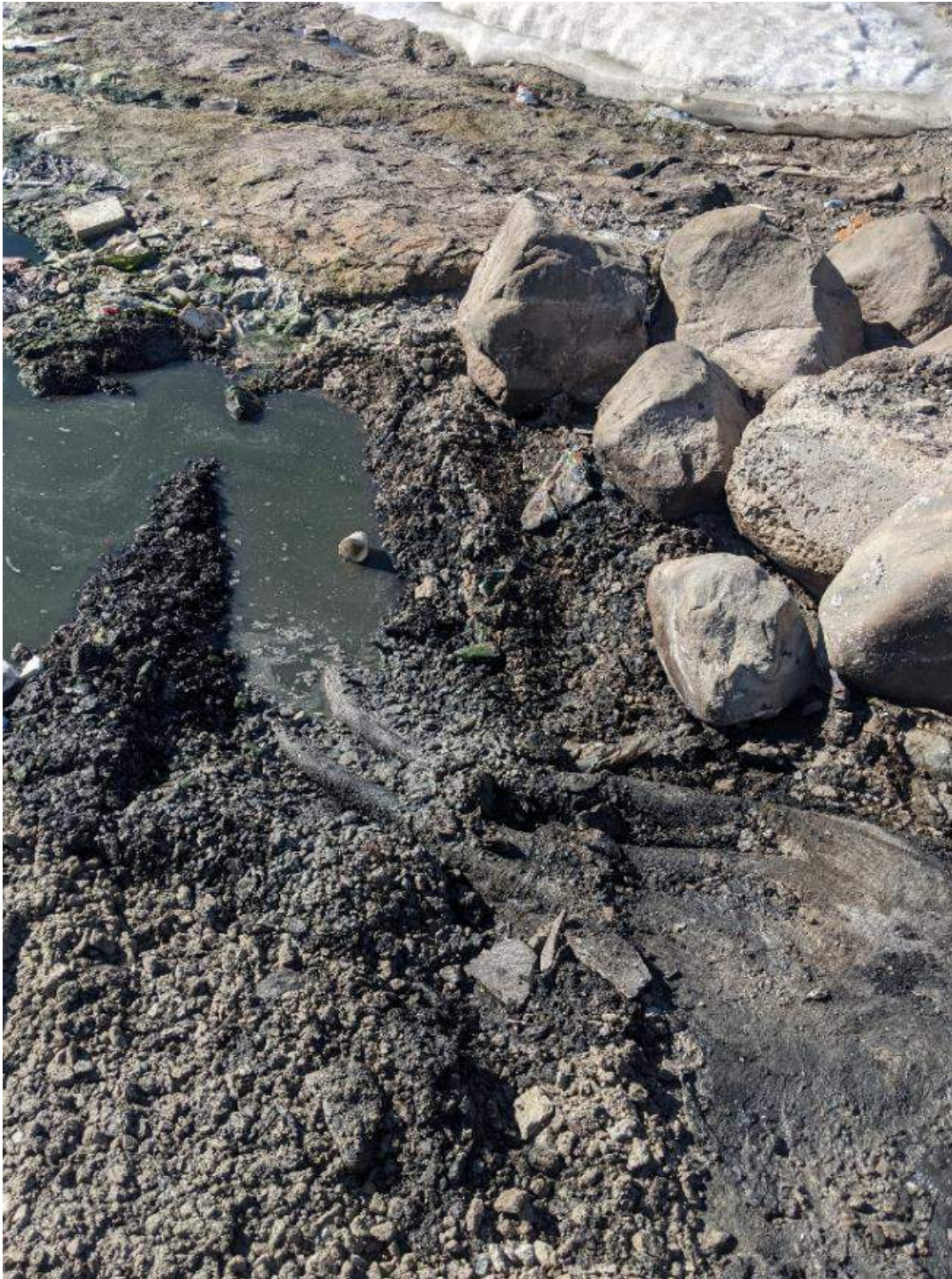
Photograph #2: Several of the large rocks were resting directly on the liner. Once the rocks were removed, the liner can clearly be seen to be folded over and damaged. A clearer picture will be obtained once the fines are removed, which will occur once the water within the lagoon is drained (seen here at left).
