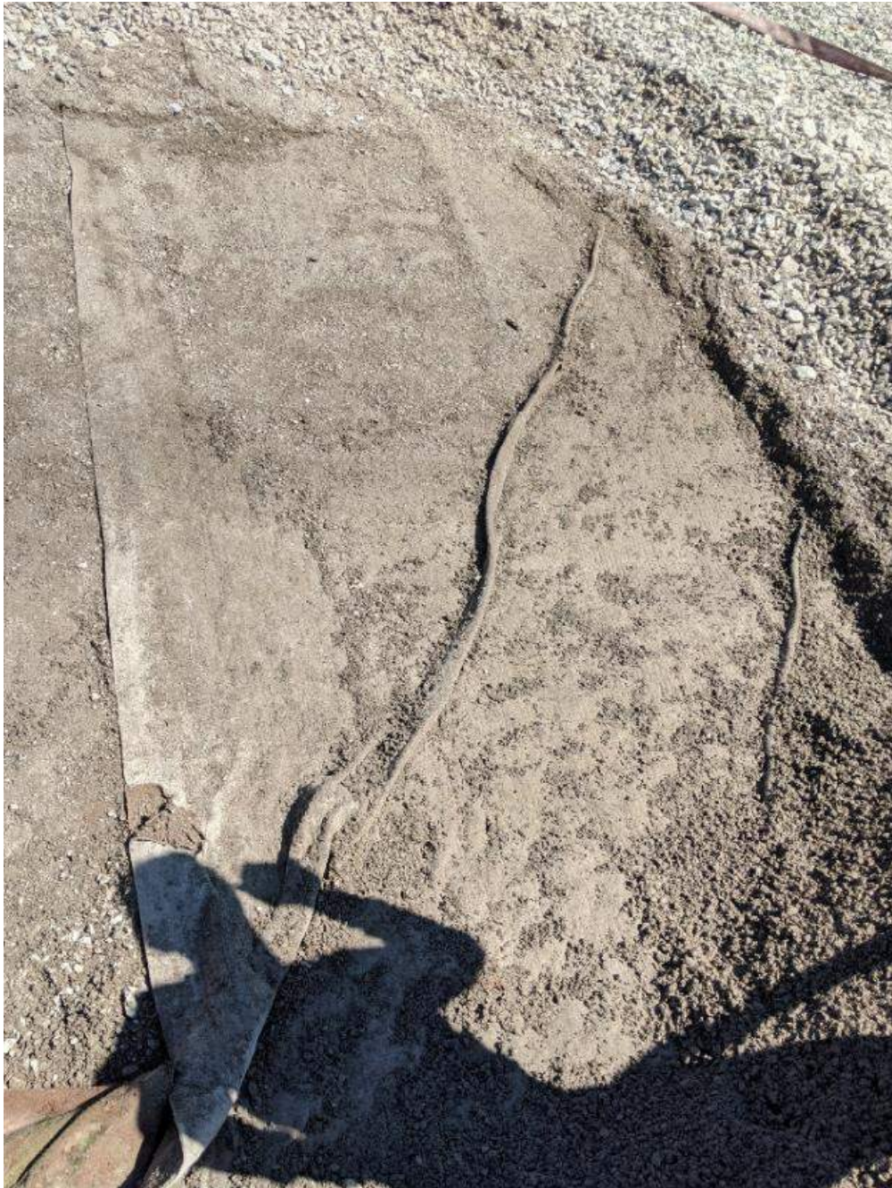
Photograph #1: Wrinkling found on a liner panel, leaving the lower left side open for water to flow under the liner.
