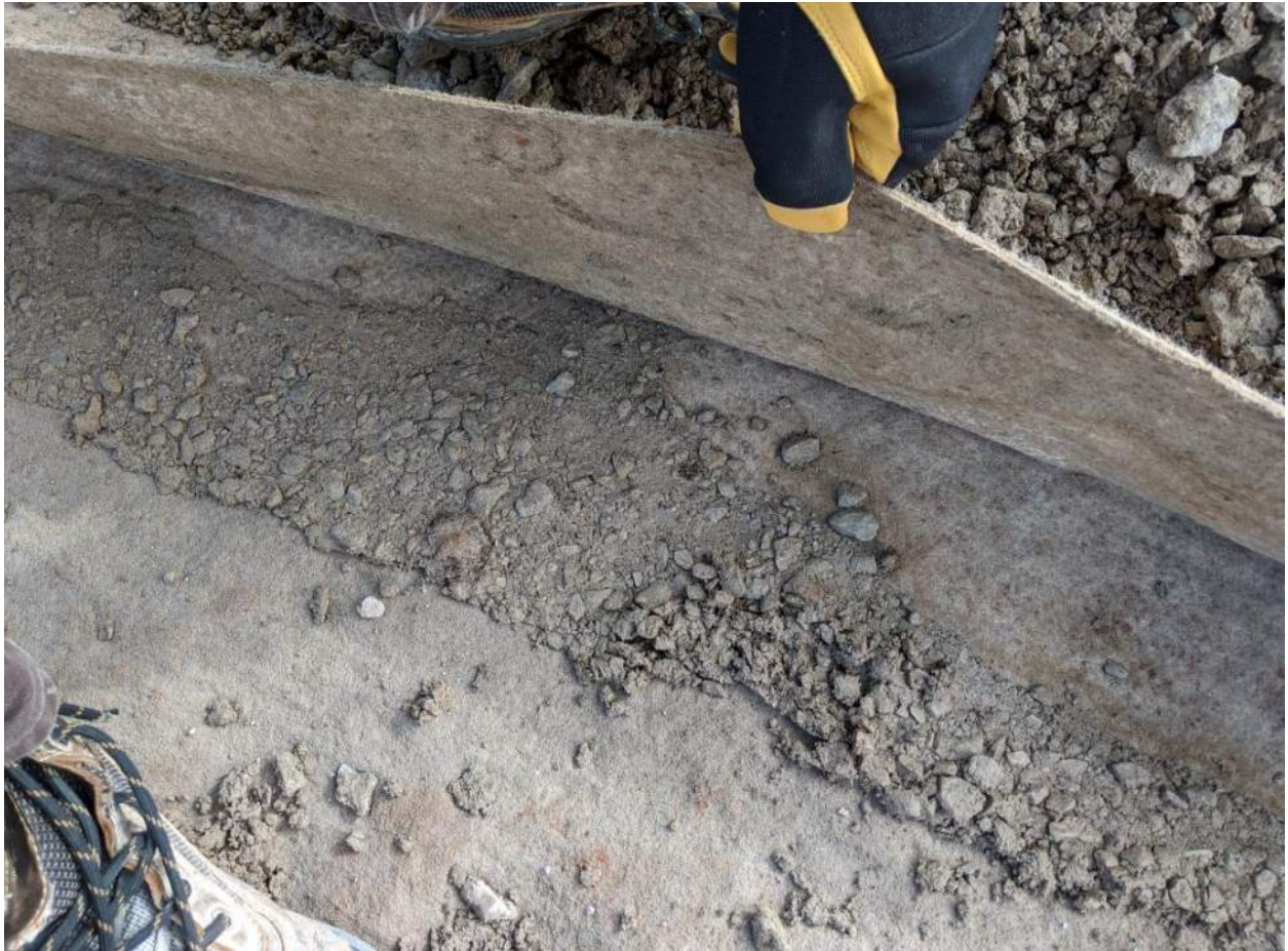
Photograph #2: Gravel compressed between the liner layers, even deep into the joint.
