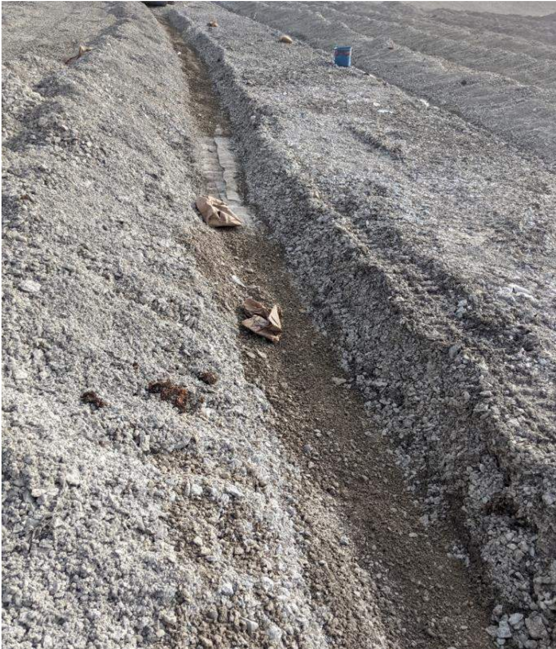
Photograph #1: Bentonite has been applied and the seam buried with fine aggregates. The areas around the north-south seams are being left open to allow for easy location and exposure of these seams once the east-west seams have been restored.
