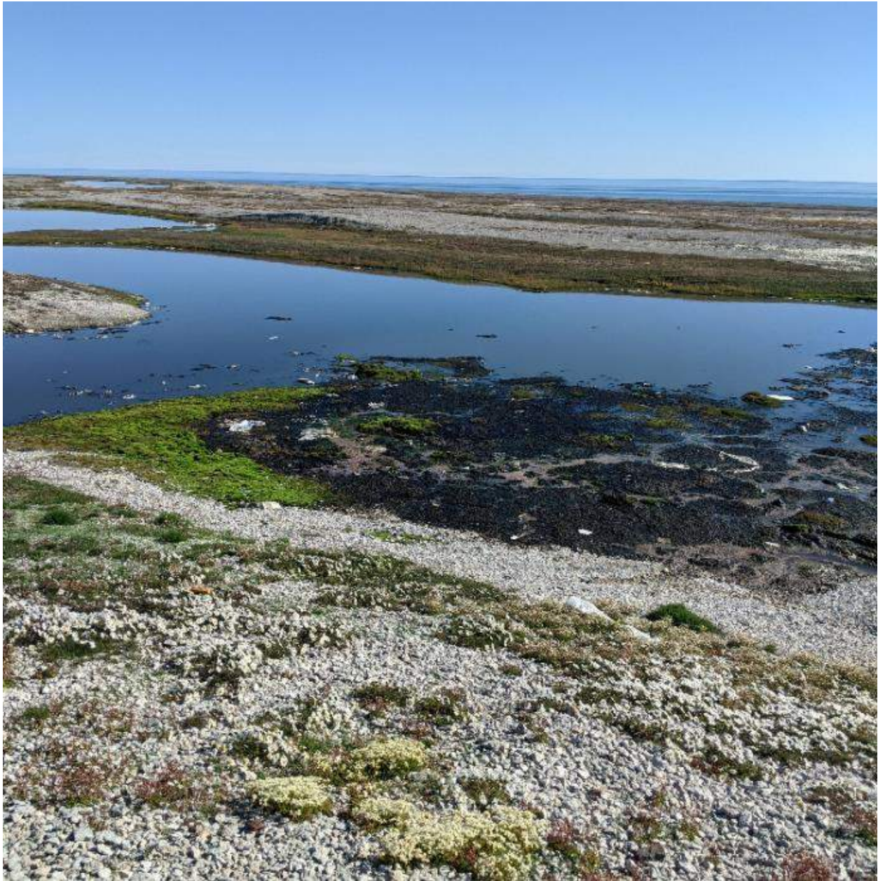
Photograph #5: There is an accumulatio of black matter outside the north cell's northeast corner. The water level in the area is also at or higher than the level where the water was coming out of the ground in this area. It is difficult to tell whether there is still water coming from the ground, and in what quantity.
