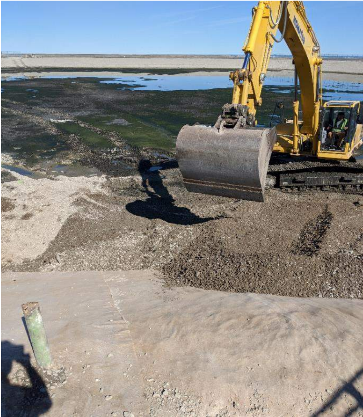
Photograph #3: Liner was covered with granular material.
