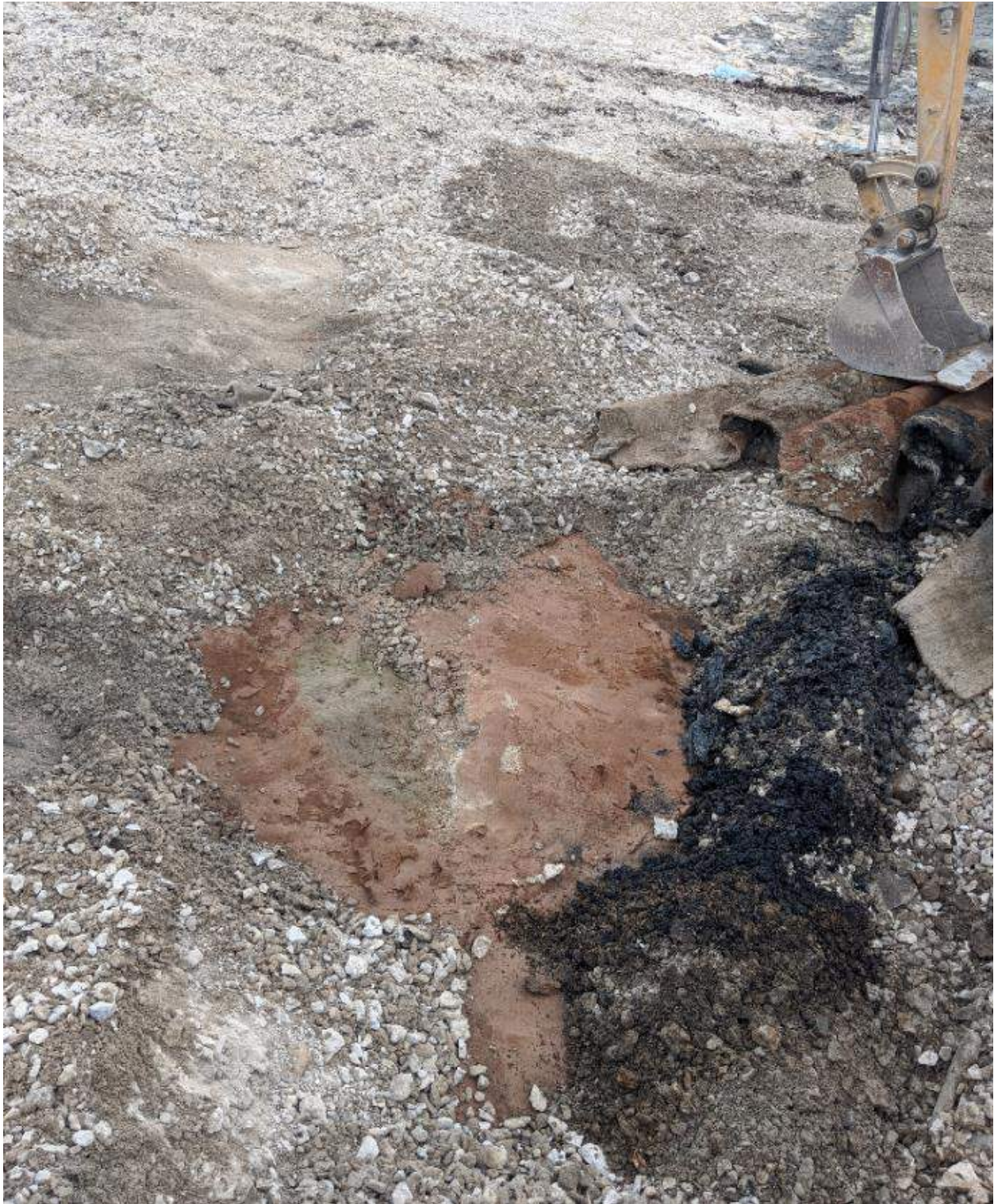
Photograph #5: Patch on embankment at north discharge station was removed. Patch was not sealed onto underlying liner.
