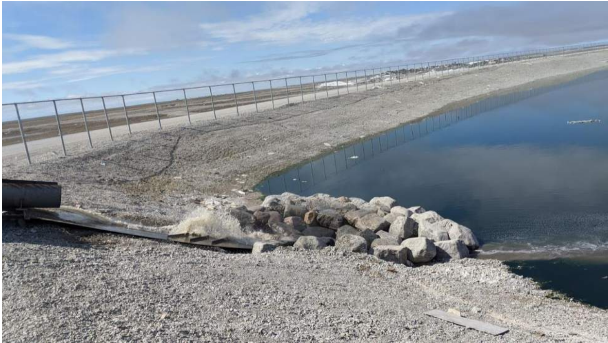
Photograph #3: South discharge station, discharge in progress. Note concentrated plume of sewage entering lagoon through rocks.
