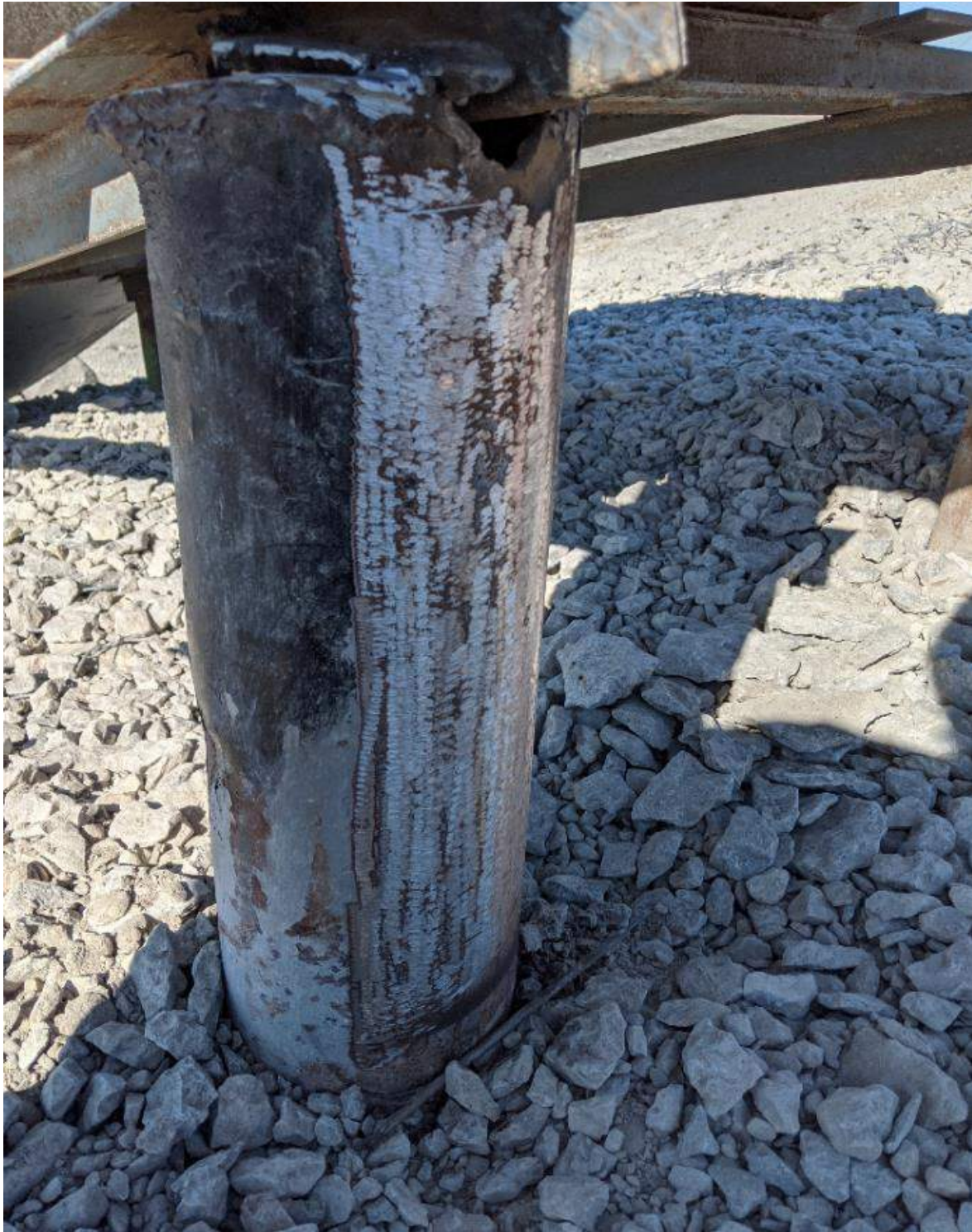
Photograph #3: The front o the piles was lightly grinded to remove paint and rust in preparation for the weld.
