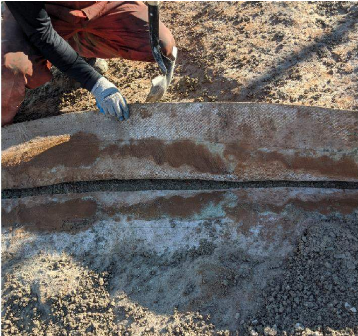
Photograph #1: Existing liner seam, showing bentonite staining within lap joint.
