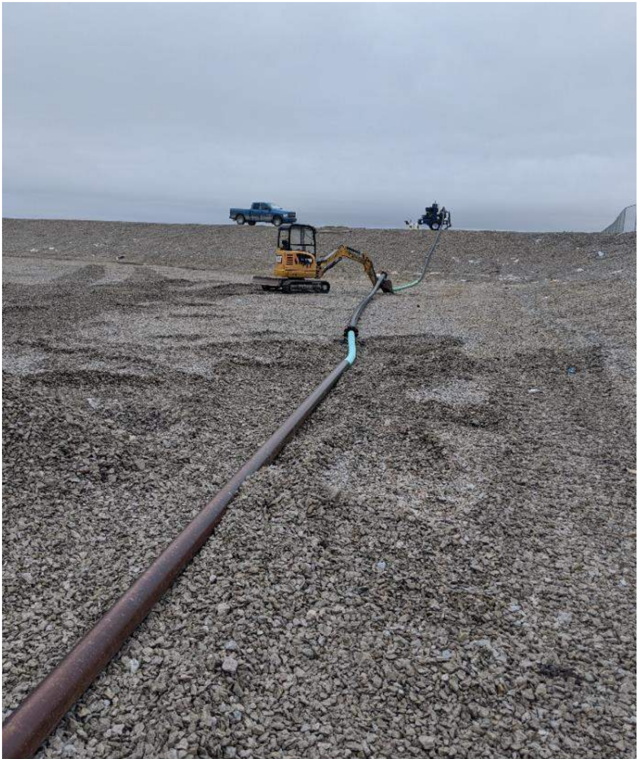
Photograph #1: Pump, with series of hoses leading to the area to be flooded.
