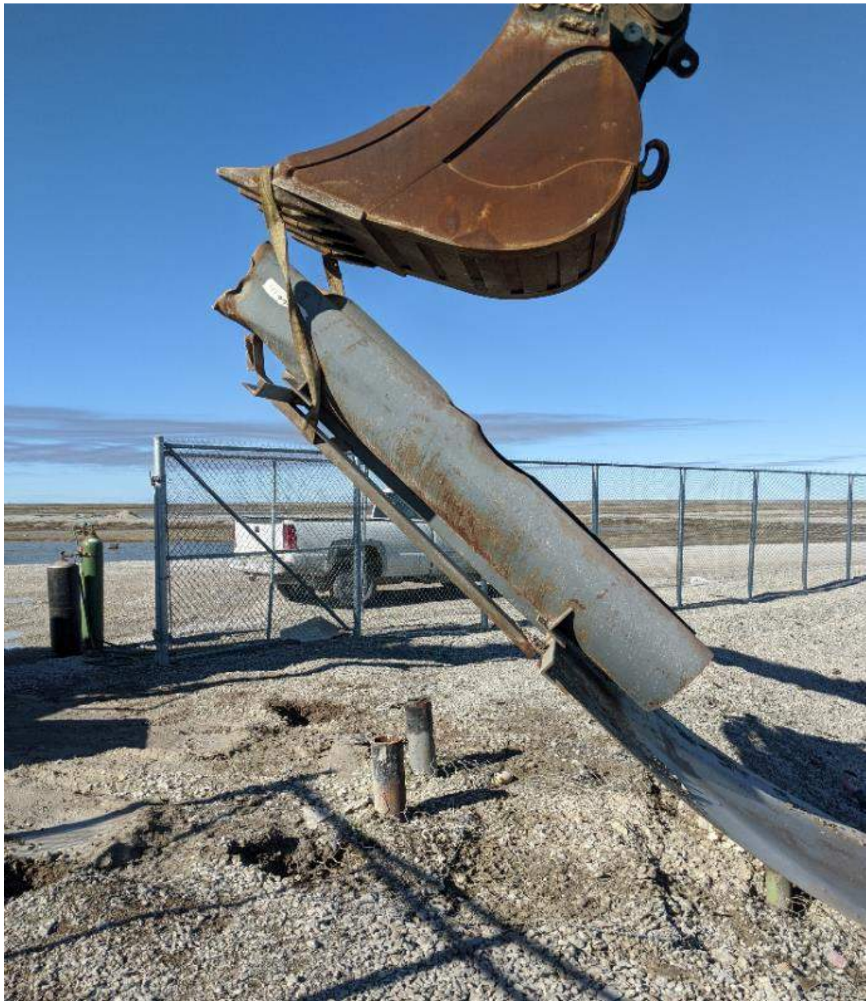
Photograph #3: After being cut off its piles, chute was removed with excavator.
