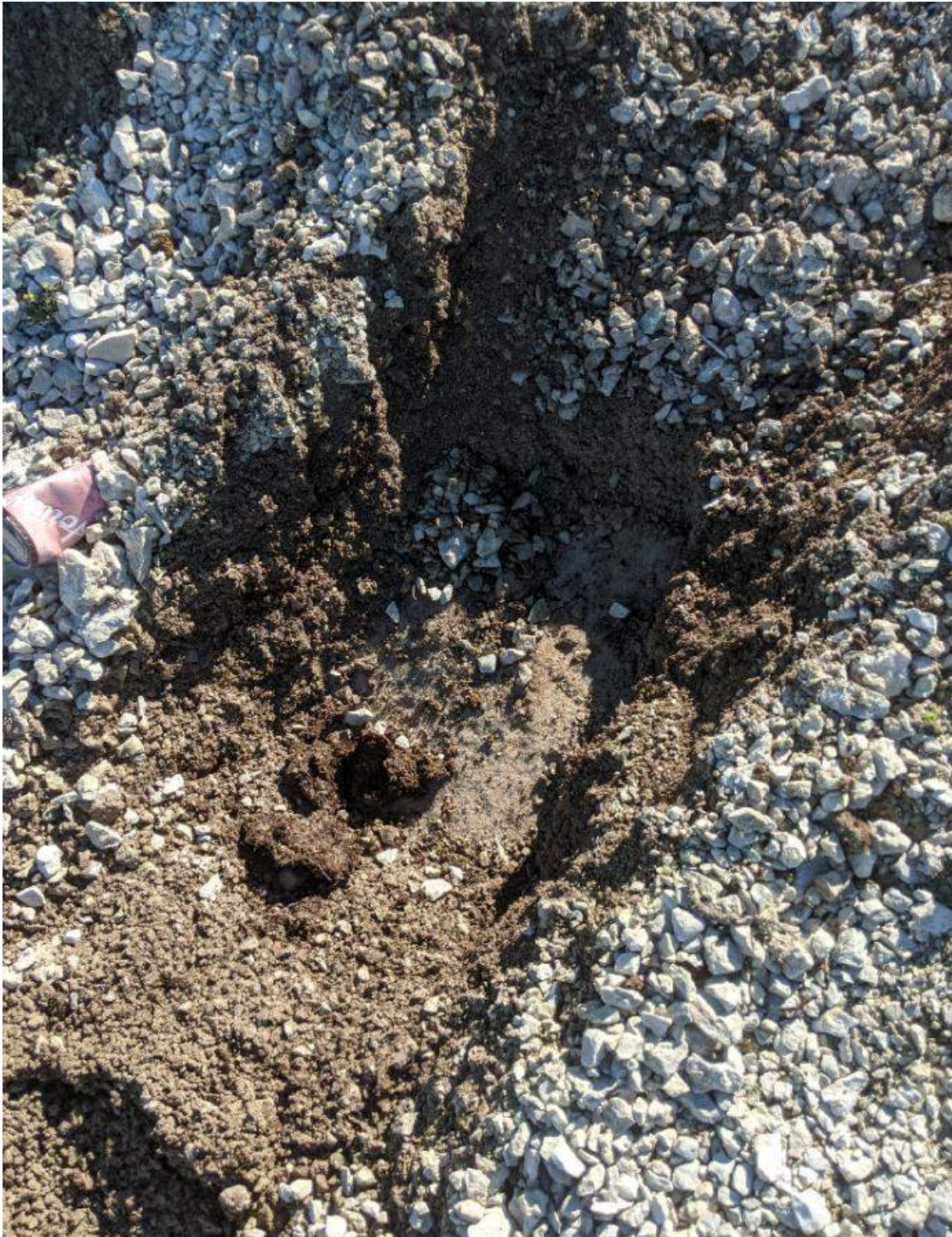
Photograph #4: Liner was exposed by hand to gauge depth. There appears to be approx. 0.4m of material left over liner, as a general average.
