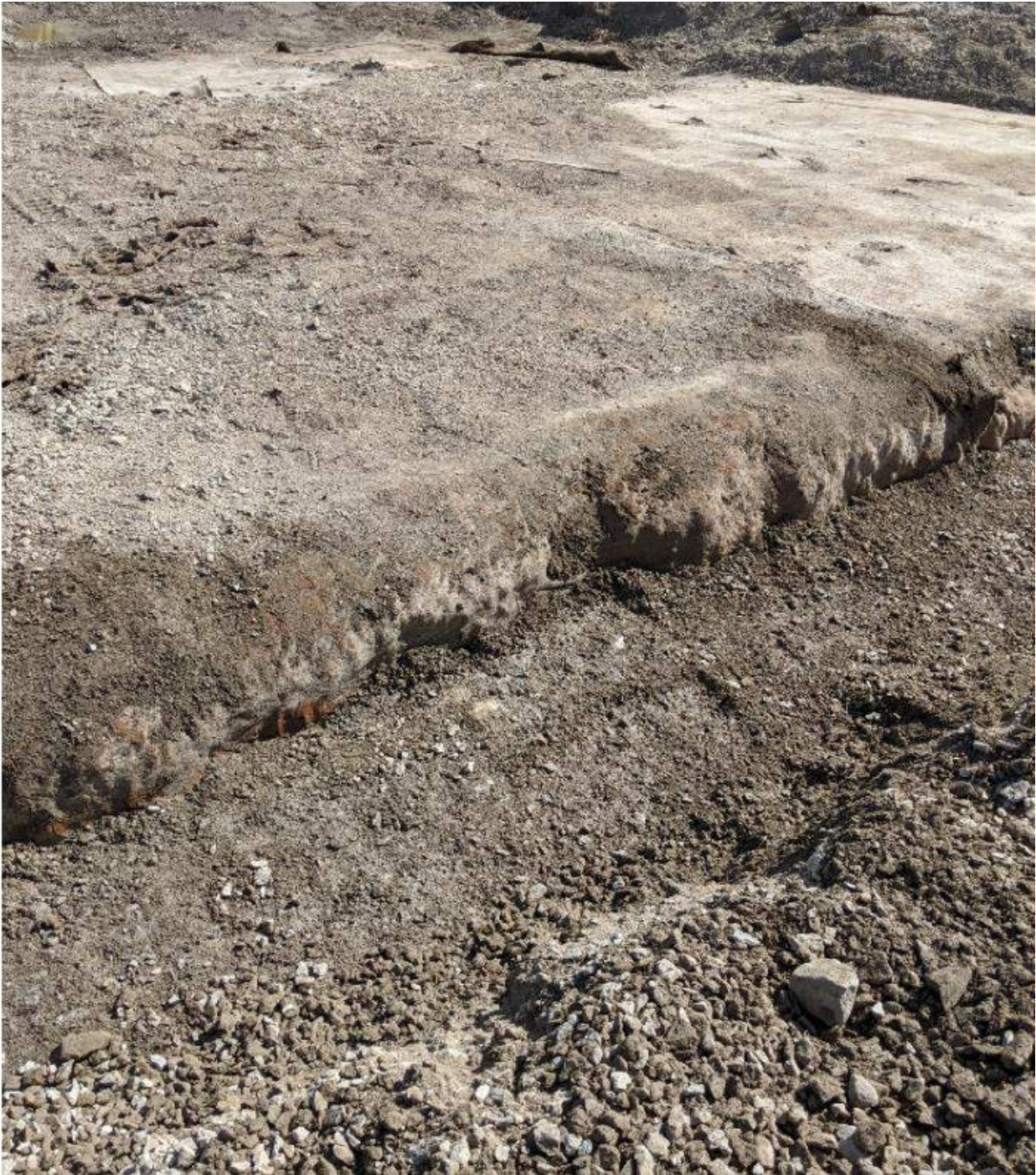
Photograph #4: The anchor trench for the new liner, located immediately behind the existing liner's anchor point, was dug.
