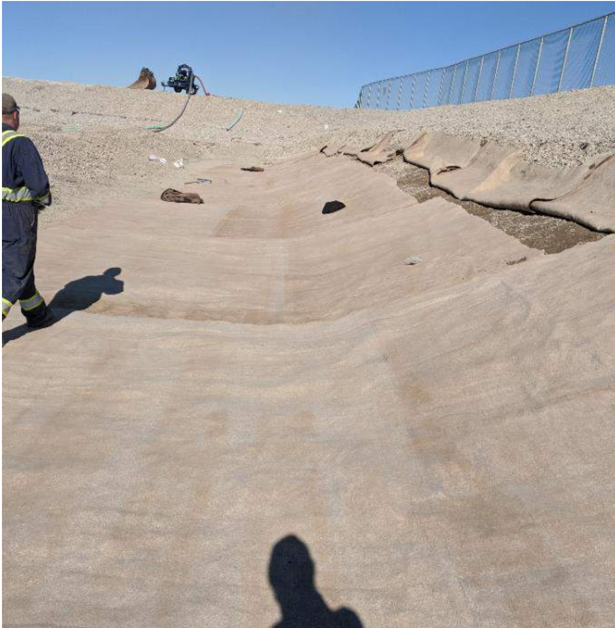
Photograph #4: New liner installed. The top flap of the existing liner will be rolled down once the seams are properly sealed with bentonite.
