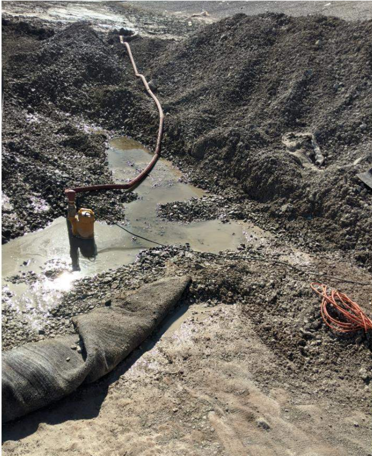
Photograph #2: A pump was used to drain the water at the bottom of the embankment, but had difficulty keeping up. The soil to the right of the picture still needs to be removed in order to prepare a clean dry joint for the new liner.
