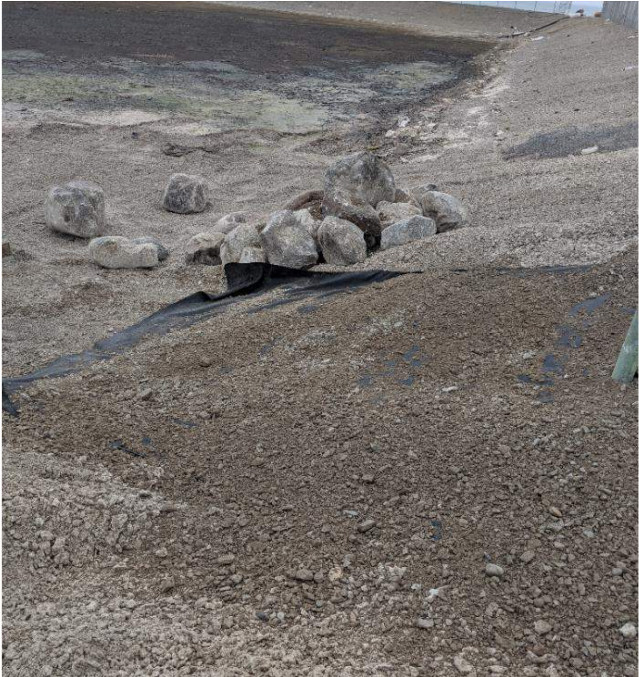
Photograph #1: Geotextile installed at south discharge station.
