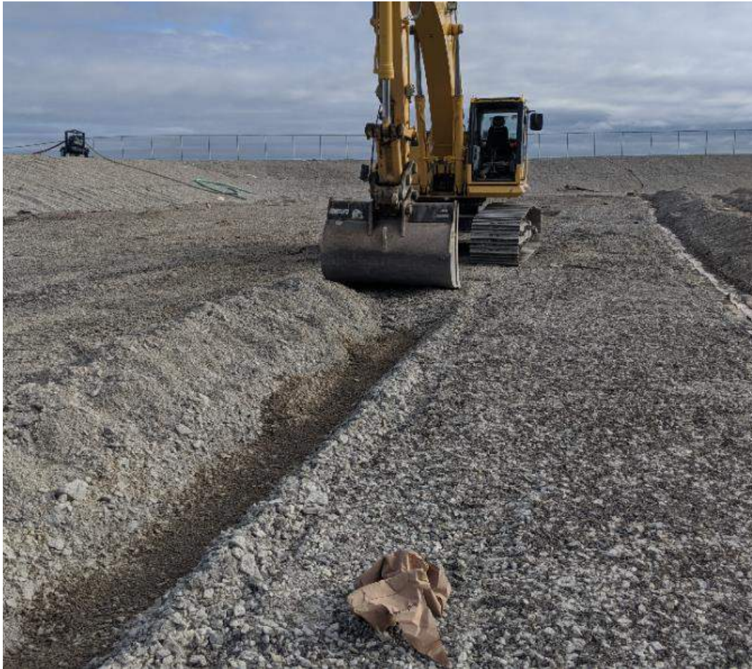
Photograph #3: Covering of the fine aggregates with the aggregates removed during the exposure process, shortly after placement of the bentonite and fines.
