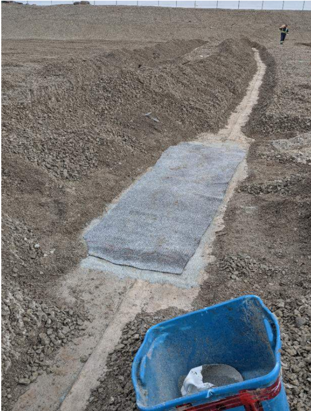
Photograph #2: Installed patch.
