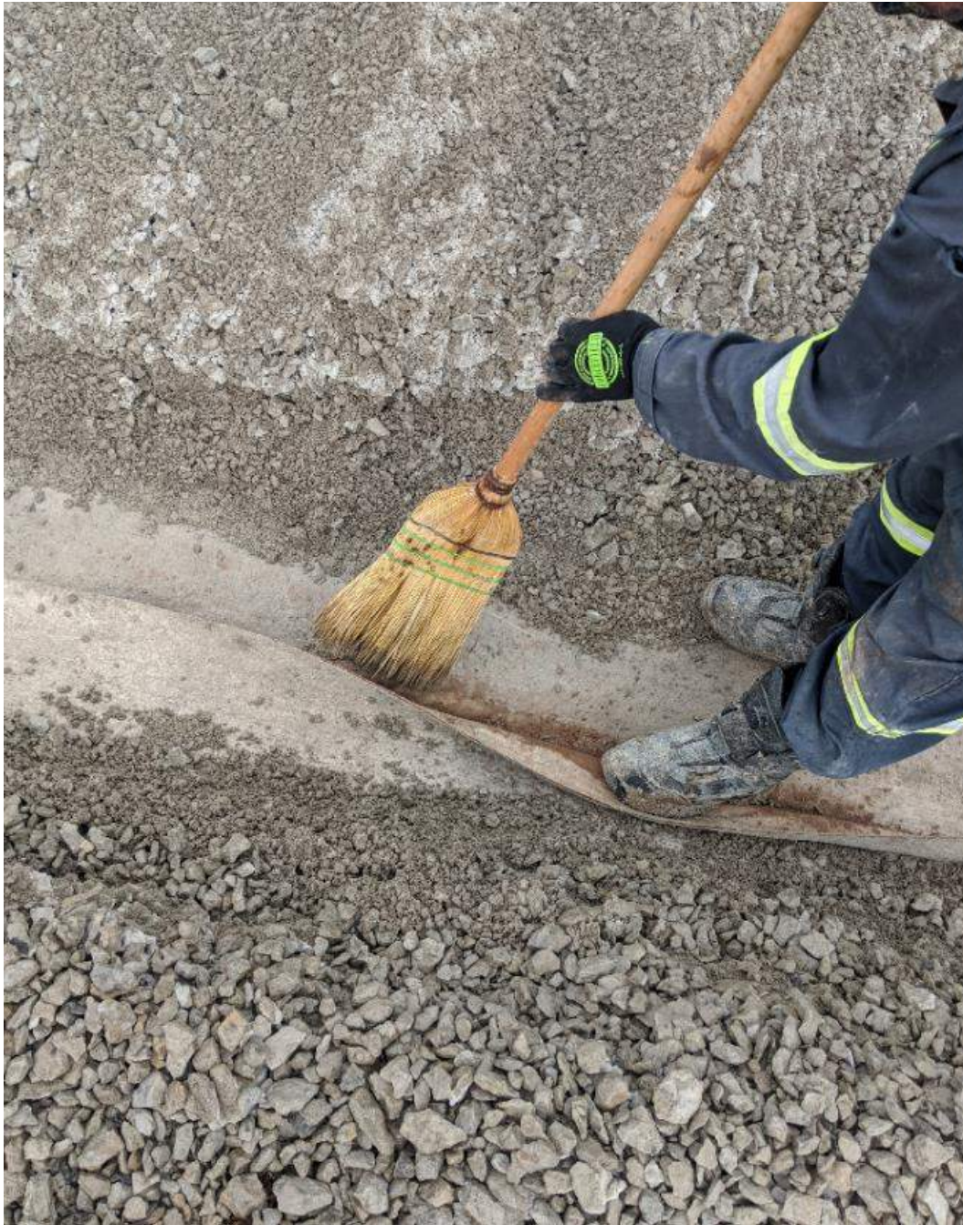
Photograph #3: Joints are broom cleaned prior to the placement of new bentonite.
