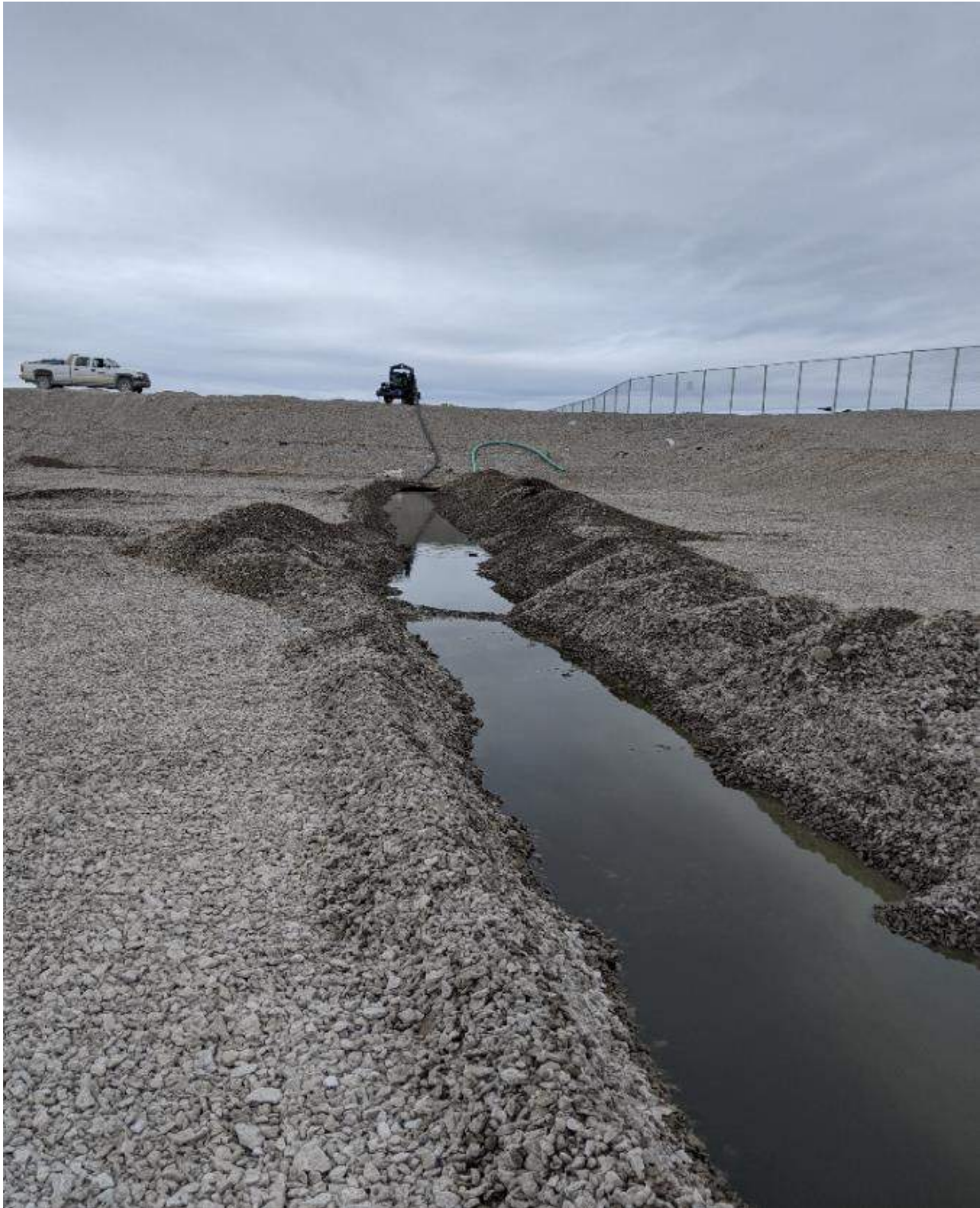
Photograph #2: Single channel dug to delimit the extent of the pool created yesterday. By digging until dry material was encountered, the area to be searched for leaks can be restricted to within the wet area.
