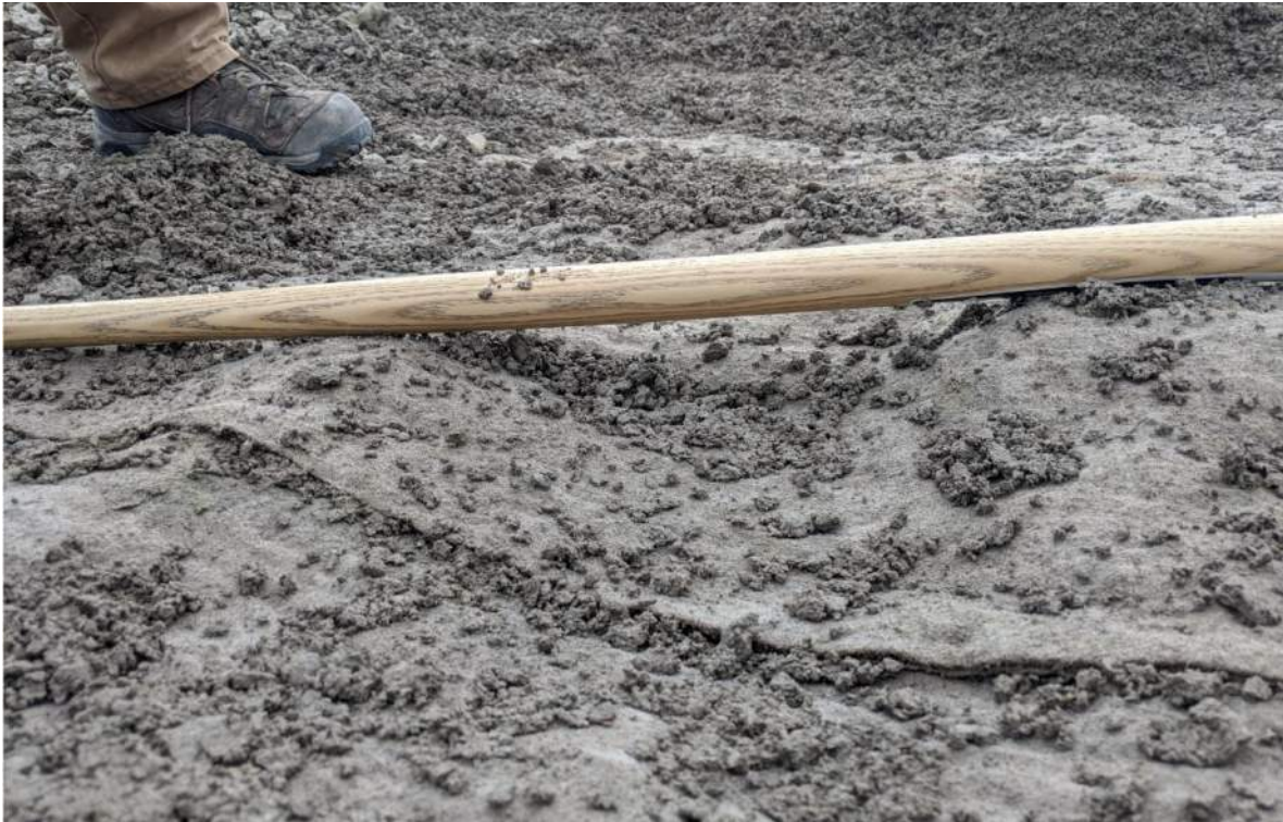
Photograph #3: The liner at the bottom of the lagoon is not even. Significant local depressions are commonplace.
