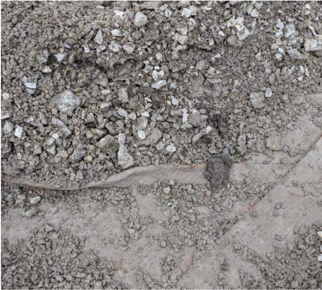
Photograph #4: Major roll next to a liner seam. The roll will be cut out and patched later on during the seam re-sealing process, prior to backfilling.
