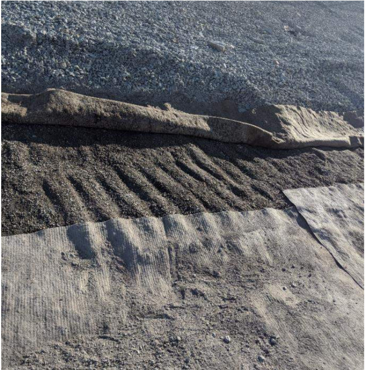
Photograph #1: The existing liner was cut and the top part rolled back to expose the soil underneath. In some parts, the soil showed patterns of having been driven over with a vehicle with cleated tracks.
