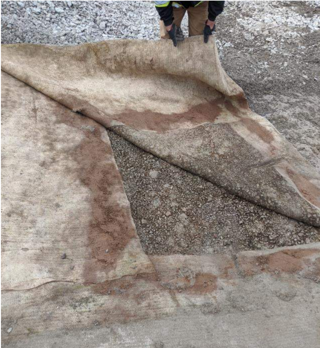
Photograph #2: Corner of a liner panel, at the bottom of the east embankment. The lower panel shows proper overlap, but the top liner seems short. The bentonite strip running horizontally on the embankment (vertically in this picture) is also quite low on the hill, considering the large overlap of the horizontal joint. This joint should also be lapped in the other direction, similar to roof shingling, as opposed to the configuration found here. The configuration found here tends to accumulate aggregates into the joint from the top (cleaned away in this picture).
