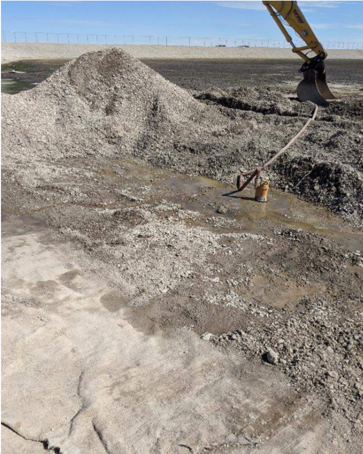
Photograph #3: The bottom of the embankment at the north discharge station is starting to dry. It will be allowed to dry further in order to ensure a proper seal of the new liner to the existing, as well as to help mitigate the issue of water bubbles under the liner.
