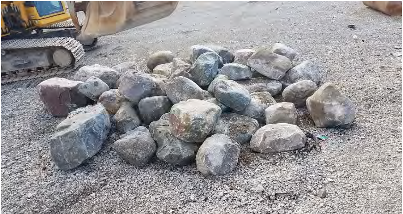
Photo 1: Larger rock that the contractor was able to collect for the south discharge repair.
