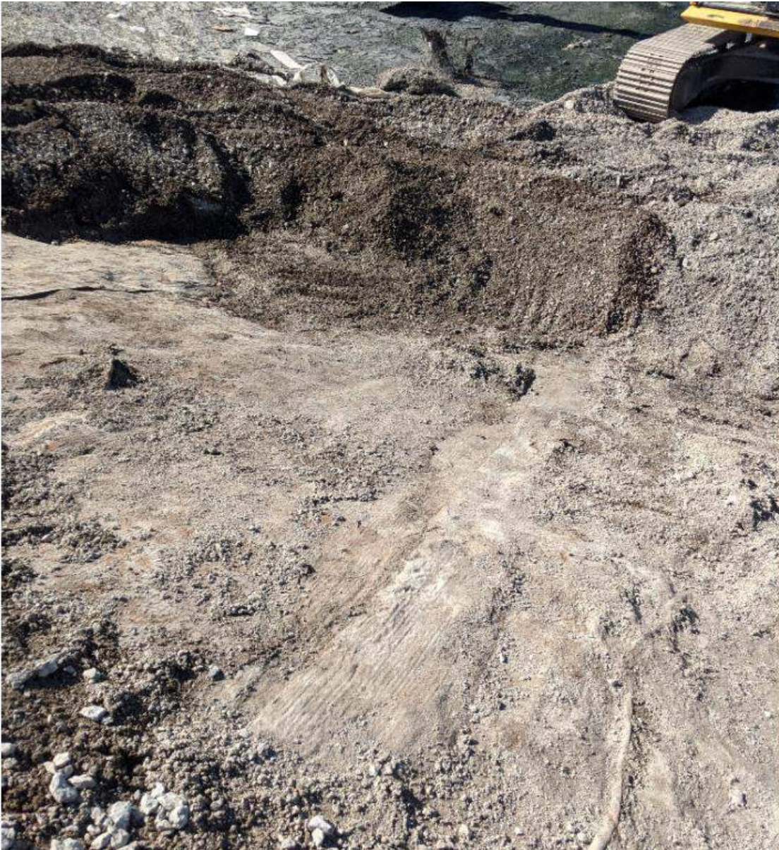
Photograph #2: Exposed liner, seen from top. Liner is largely intact. Minor damage due to process of exposing. A second liner will be applied over this one, thereby patching the holes.
