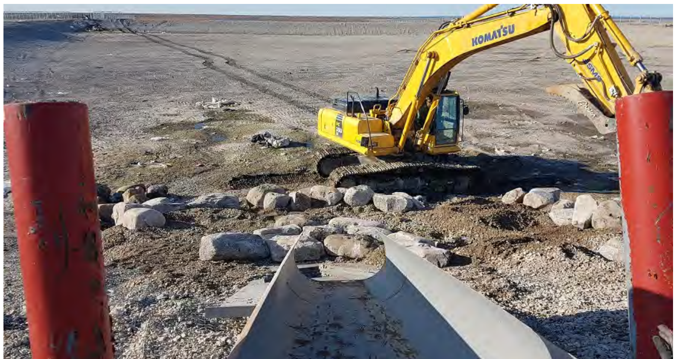
Photo 2: Progress of the south discharge repair. Placed granular material to raise grades, followed by larger stone to reduce erosion.
