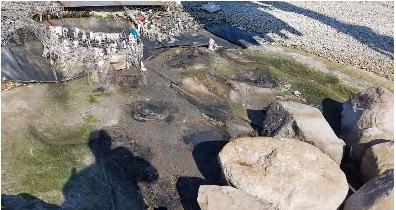
Photo 1: Large stone removed to reveal holes in GCL. Gabion baskets have had all stone eroded out.
