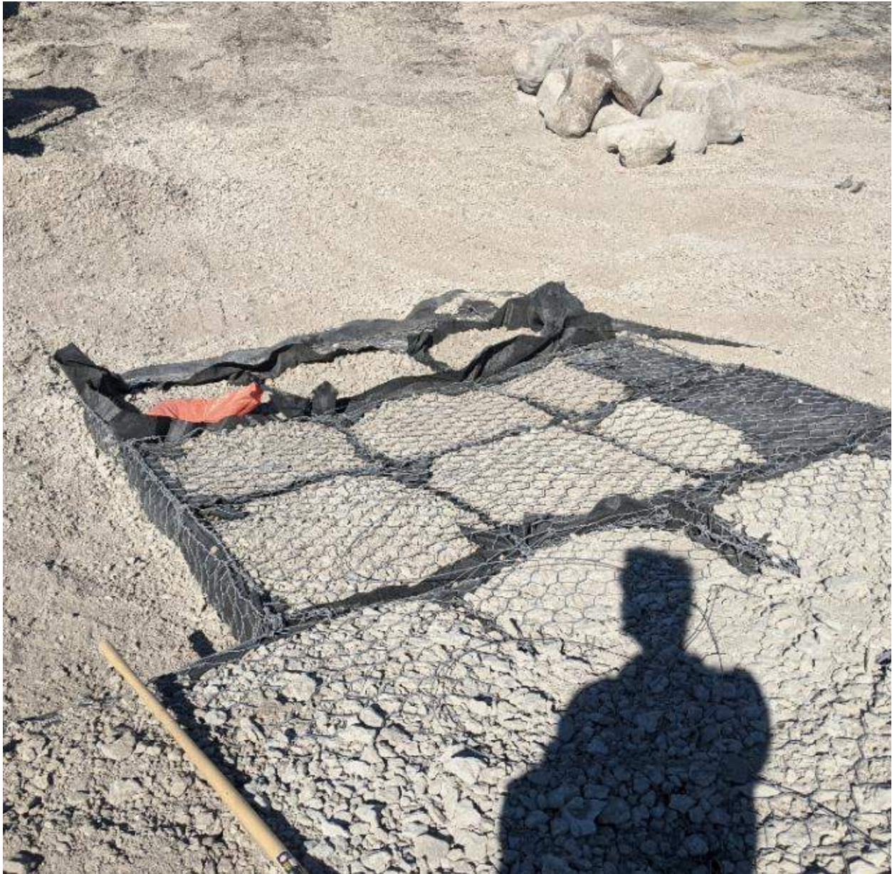
Photograph #3: This photo taken on July 14 demonstrates the geotextile used to prevent the granular material from falling out of the cages.
