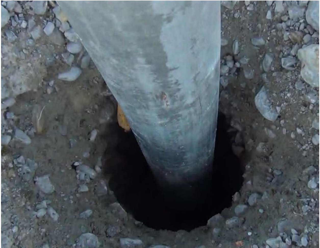
Photograph #4: Significant settlement around fence post, northeast corner of north cell.
