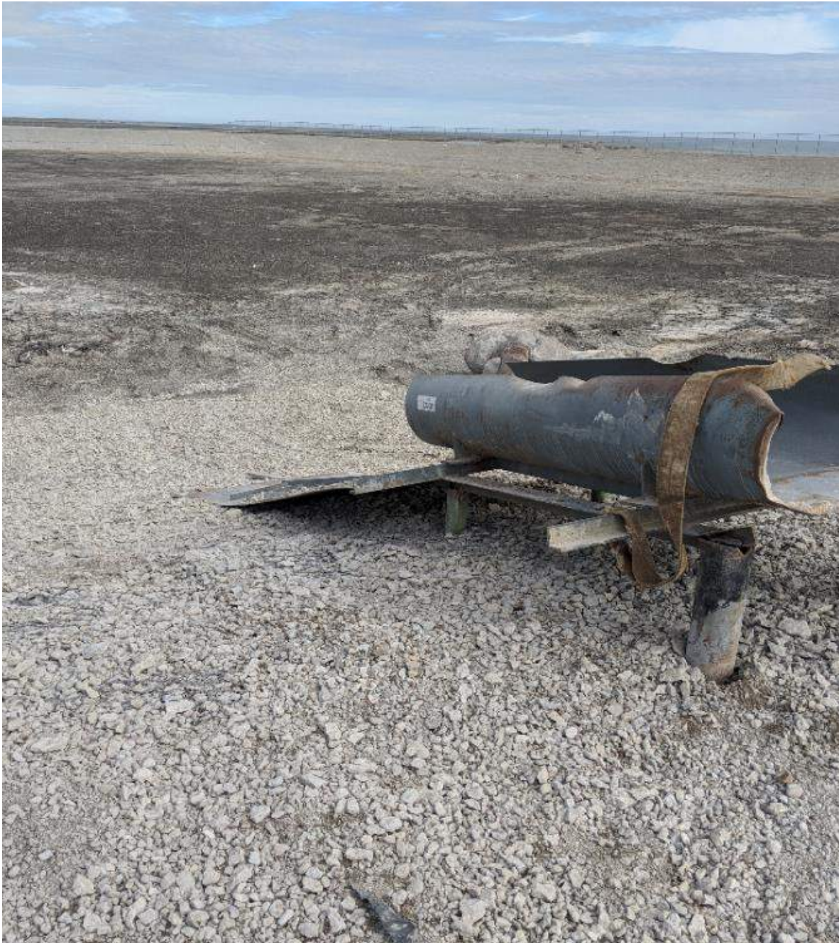
Photograph #1: The south discharge station's chute was placed onto its piles, but. The granular material is shaped over the gabion cages, and the riprap at the bottom of the chute will be installed once the chute is welded in place.
