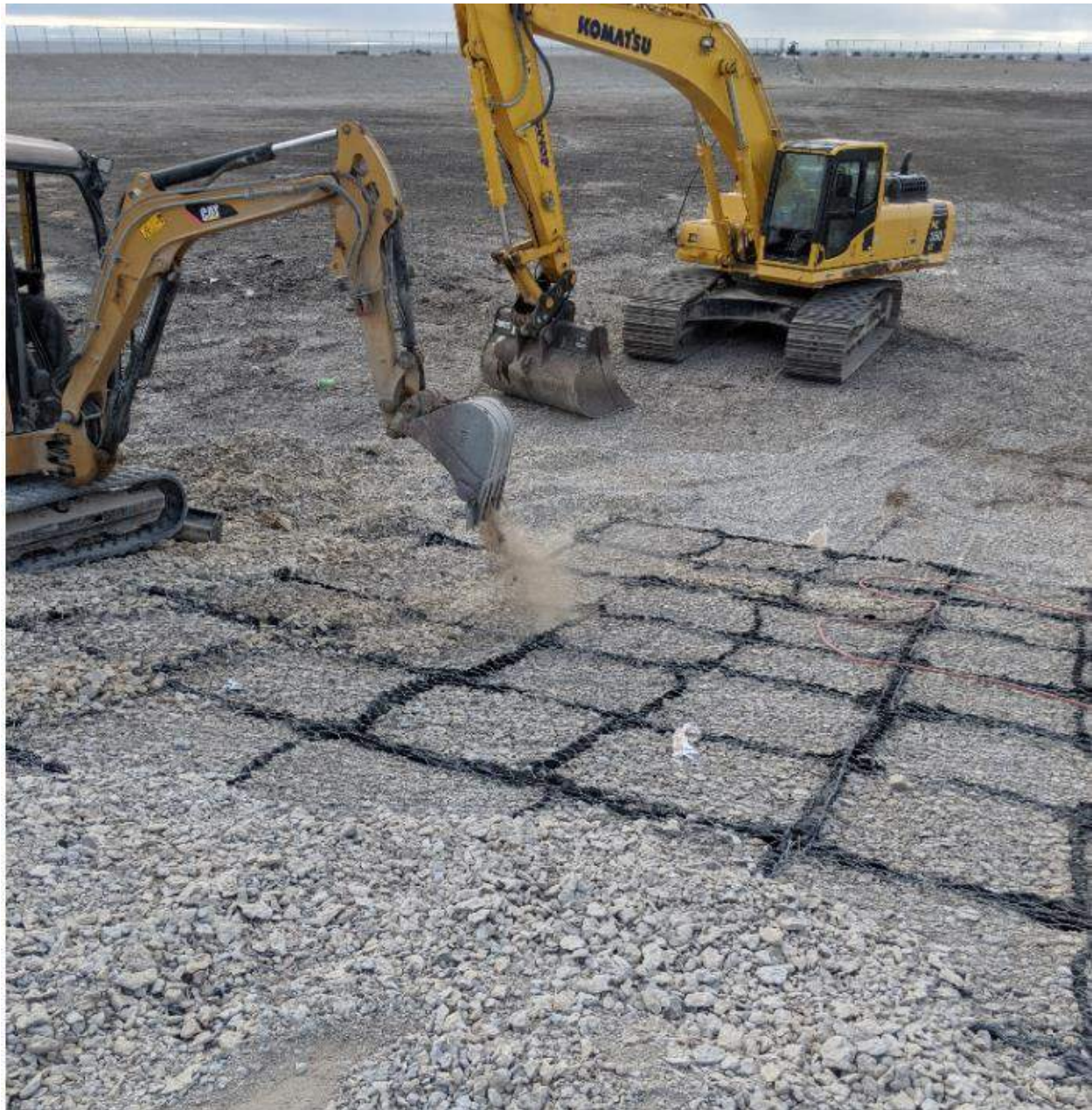
Photograph #1: Covering the newly installed gabion mat with a thin layer of aggregates.
