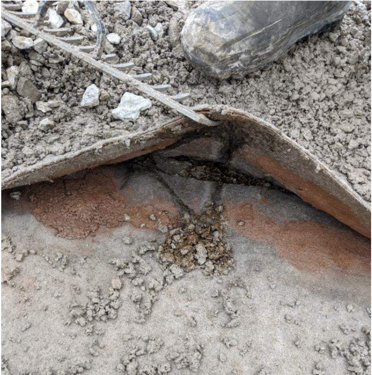
Photograph #3: Further evidence of water penetration within a liner seam. In this case, granular material was pushed within the seam, allowing water to wash out two paths into the subgrade.
