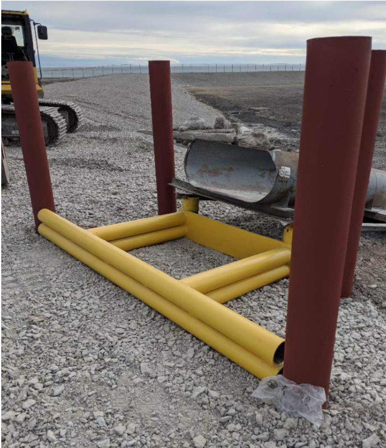
Photograph #2: Final configuration of discharge station, with bollards and truck bumper installed and painted.
