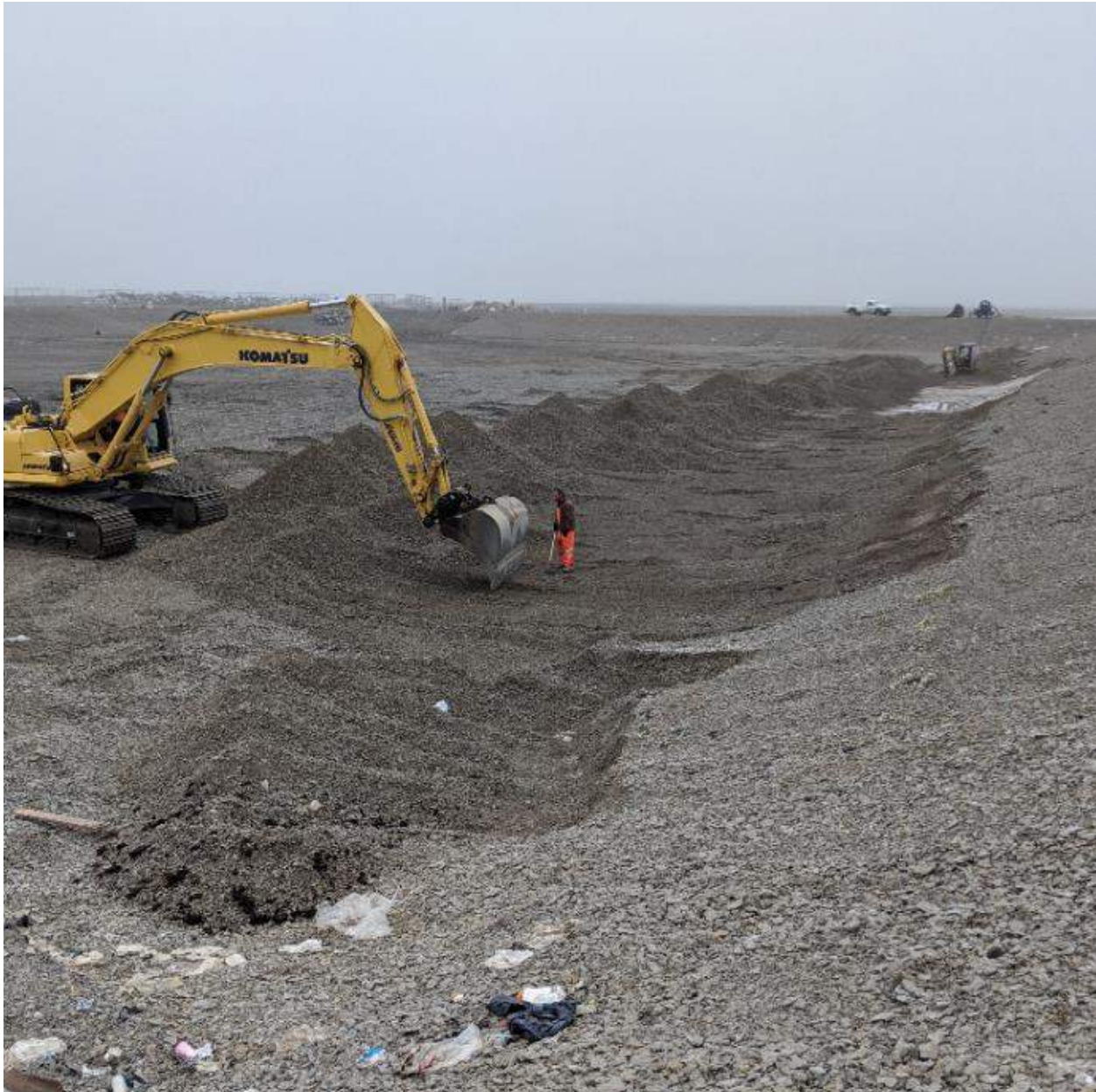
Photograph #1: Using the Komatsu to remove the top layer of aggregate. The final 100 to 150mm of sand will be removed using the mini-ex and hand tools for more accuracy and lower likelihood of damaging the liner.
