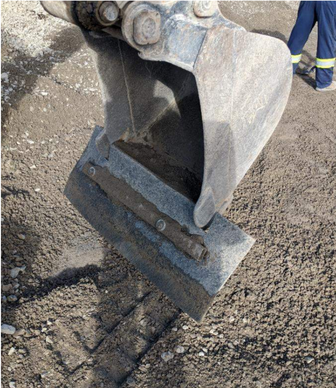
Photograph #3: Attaching a piece of 15mm thick flexible rubber to the front of the mini-excavator's bucket greatly sped up work by allowing the operator to scrape much closer to the liner, leaving less work to be done by hand. It also greatly reduced the incidence of accidental tearing of the liner by the excavator.
