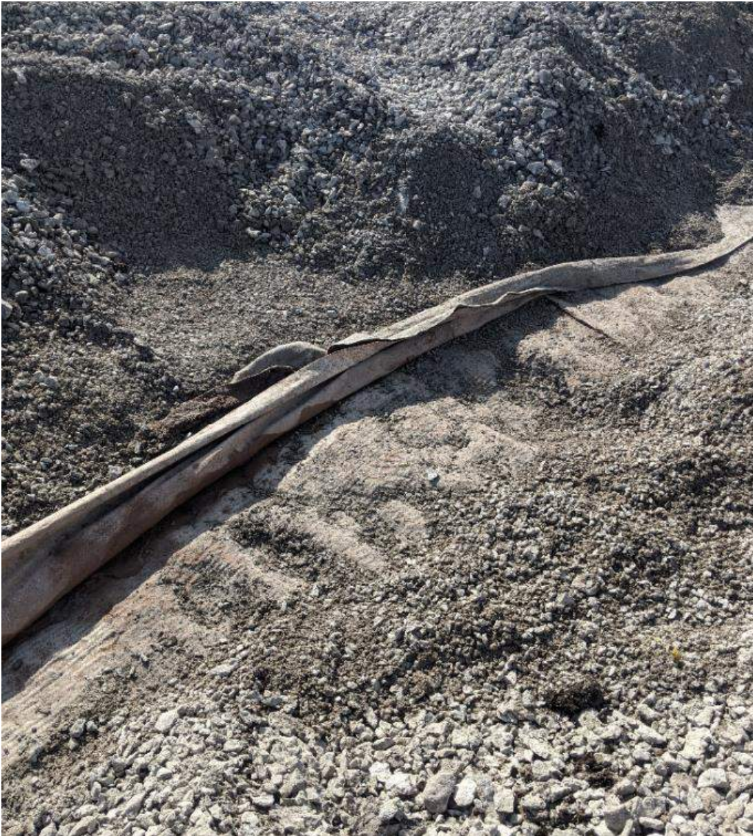
Photograph #2: In addition to damage to the seam's upper layer, gravel was present through the full width of this particular defect, creating a path for water to penetrate all the way to the bentonite seal, and potentially to the subgrade.
