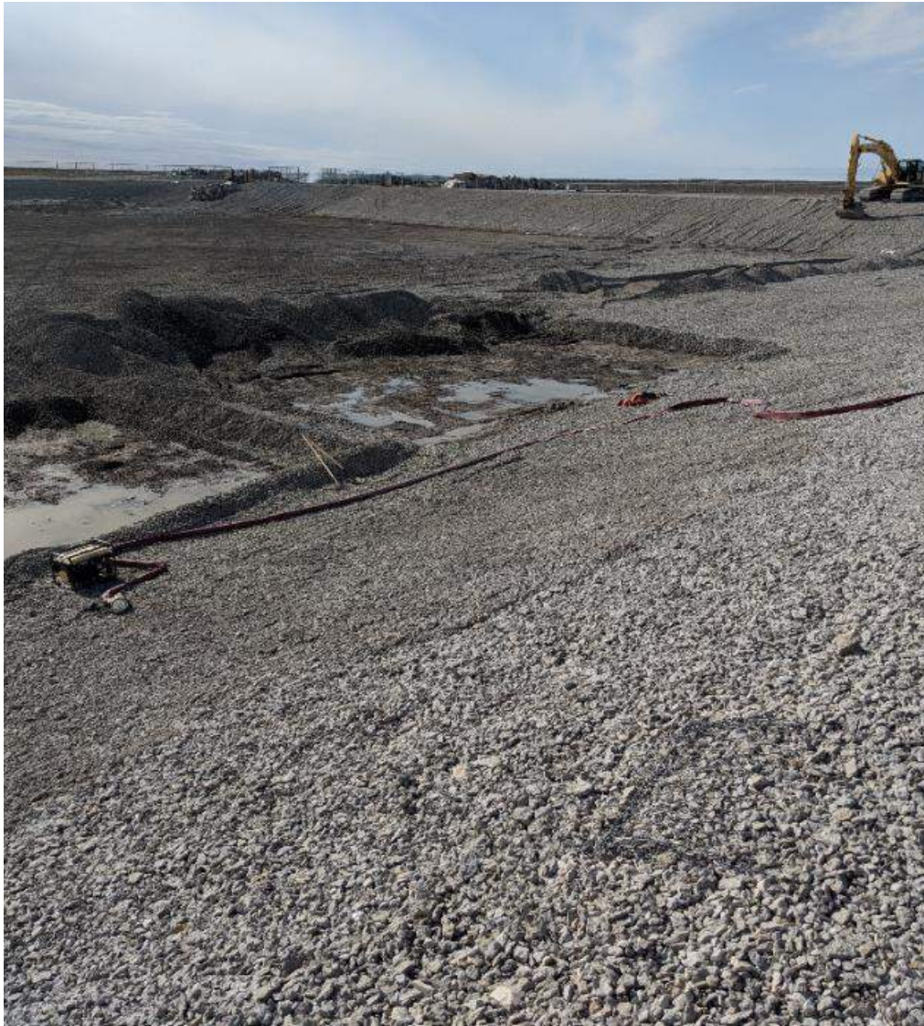
Photograph #2: Exposed area at end of day. Water appears to be retained on the liner in several areas, which was taken as an encouraging sign.
