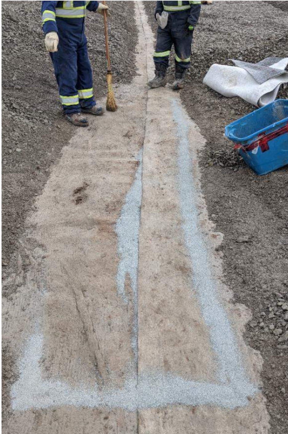
Photograph #1: Installation of patch over area where liner overlap is insufficient.
