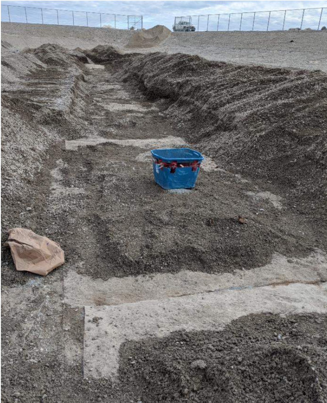
Photograph #3: The seams around each patch were exposed and resealed.
