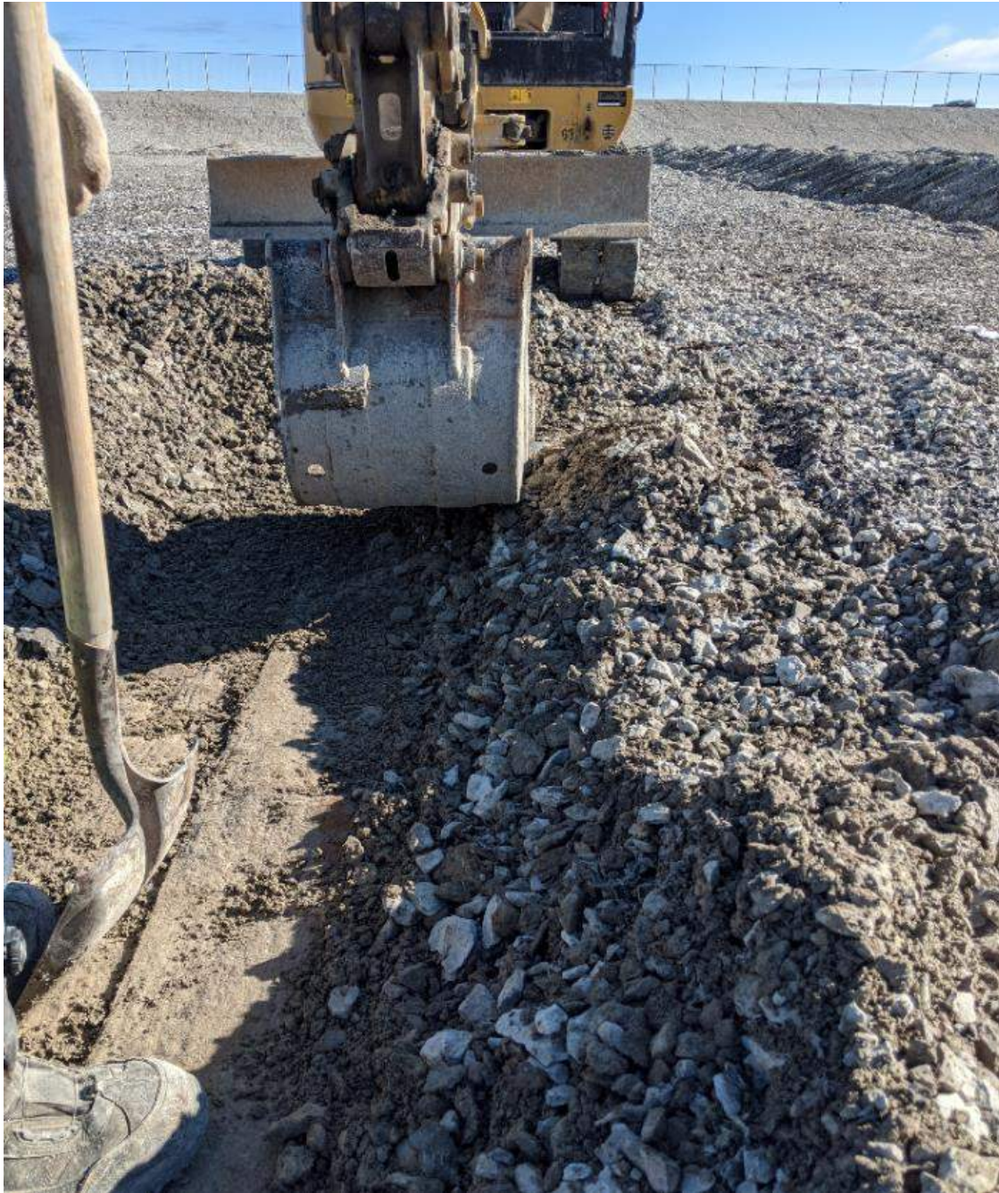
Photograph #1: In one location, the total depth to liner was less than 200mm. The mini-excavator's bucket is level with the undisturbed aggregate surface in this photo.
