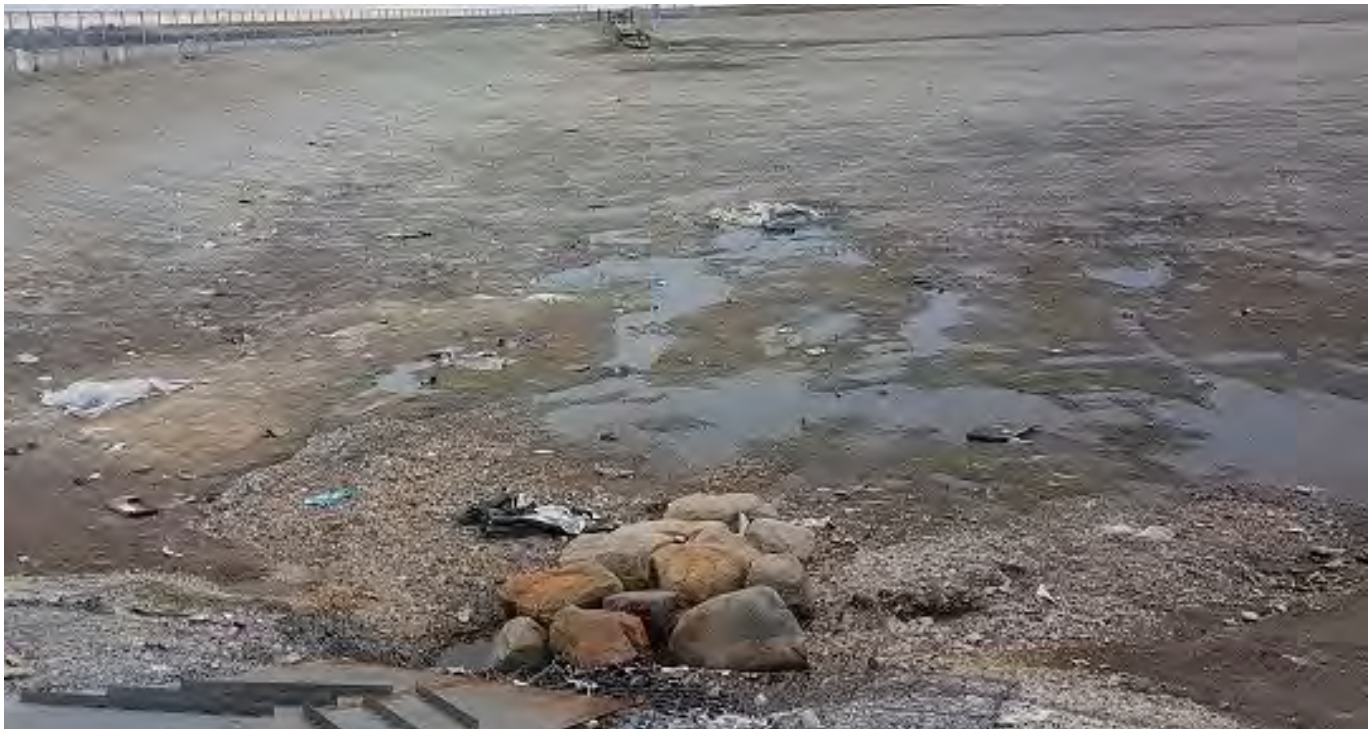
Photo 1: View of western side of the lagoon from the south discharge location. Hamlet had been using this cell for disposal, as evidenced by the liquid at the surface at both discharge locations.
