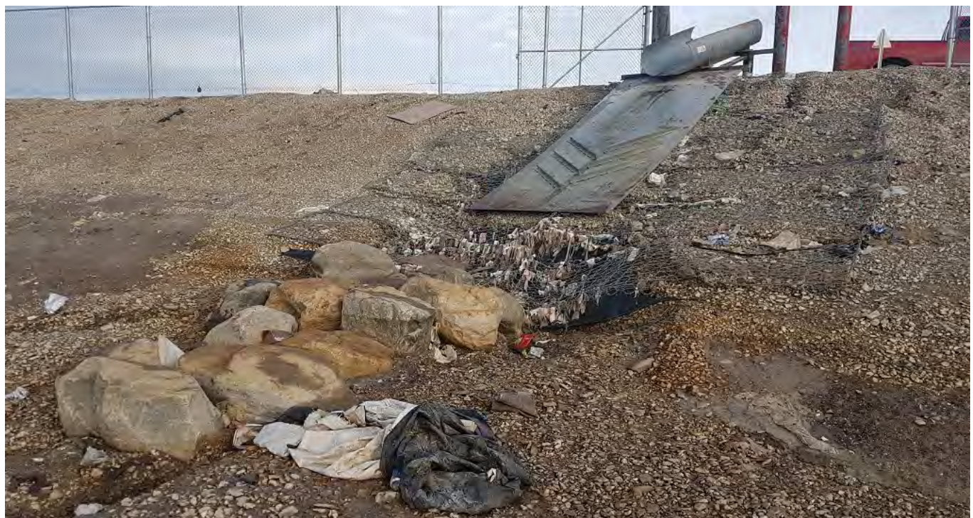
Photo 6: South discharge area. Areas of localized erosion to expose GCL. Gabion baskets eroded at bottom of discharge.
