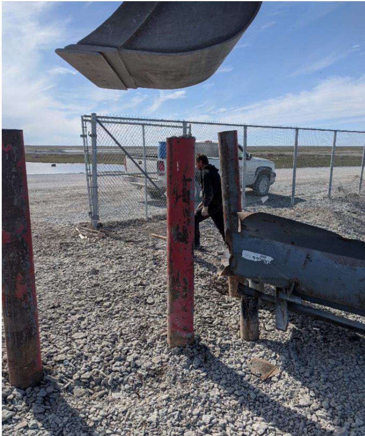
Photograph #1: Installation of the bollards.
