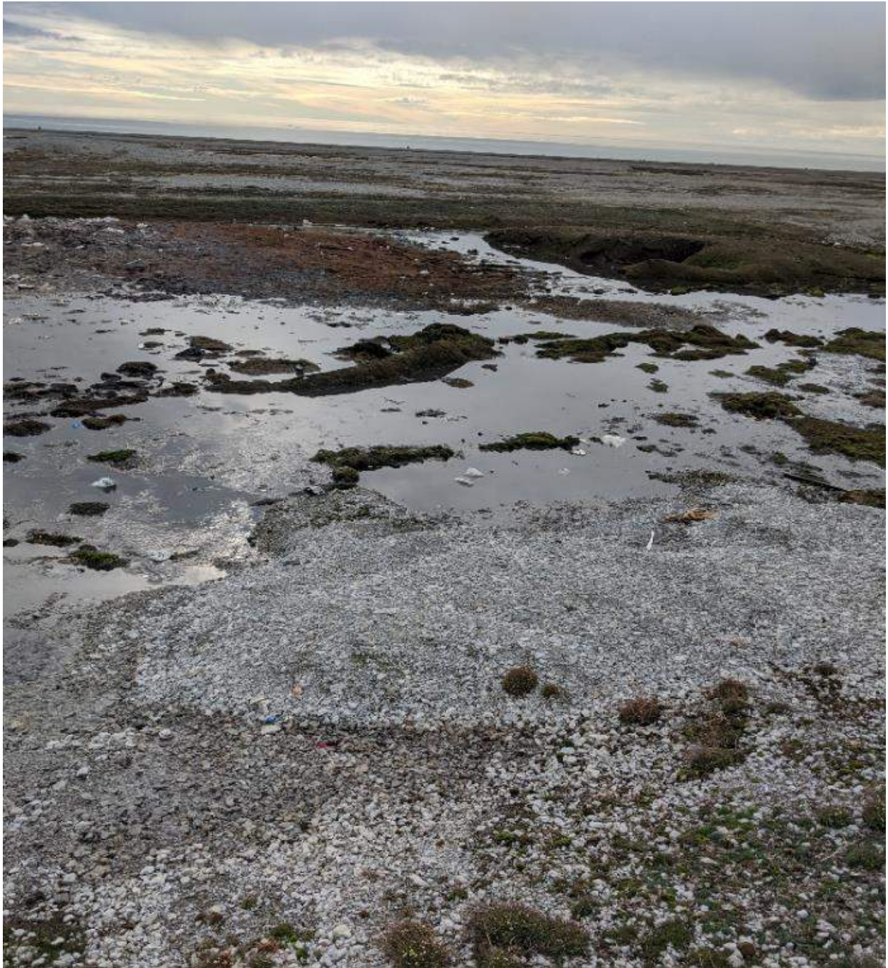
Photograph #2: Water coming out of the ground on the outside of the lagoon berm. This picture was taken at the bottom of the berm at the northeast corner of the lagoon's north cell, looking northeast.
