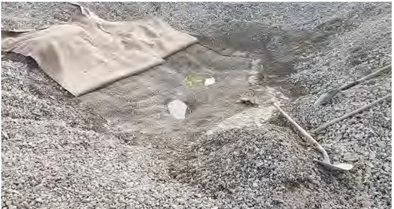
Photo 2: Area 1 upon removal of GCL. Standing water and depressions noted. Evidence of bulldozer tracks at the surface.
