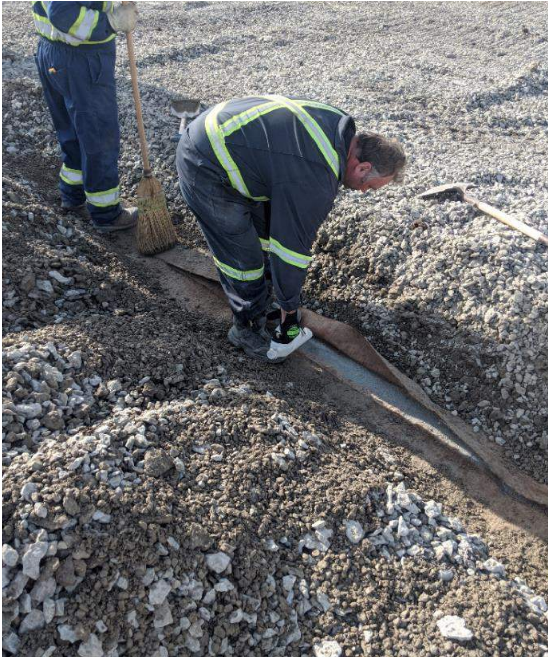
Photograph #2: North-south seam re-sealing.
