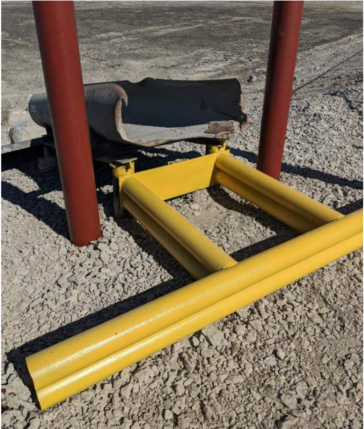
Photograph #1: The bumper at the south discharge station, installed and painted. Preference would have been for red paint to match the bollards, but the contractor could only obtain enough red paint to touch up the bollards themselves.
