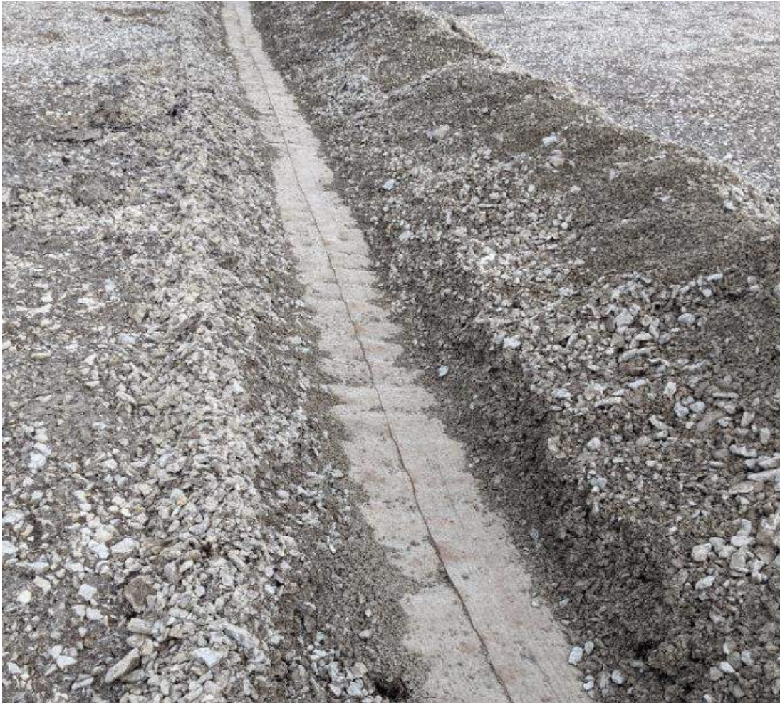
Photograph #2: The dozer track pattern is a common feature of every seam uncovered so far.
