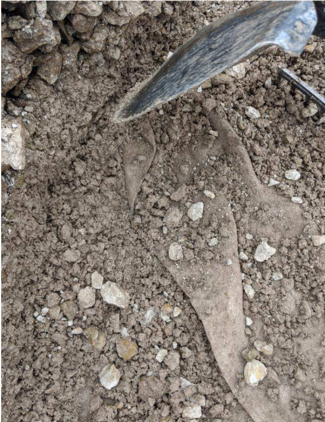
Photograph #1: Uncovering a wrinkle in a vertical seam on the lagoon's east embankment. This issue is directly across the berm from the area from which water was leaking.
