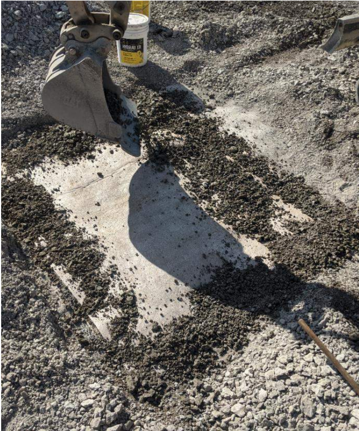
Photograph #1: A patch was placed over the damaged area in the liner, and covered with small-diameter aggregate.
