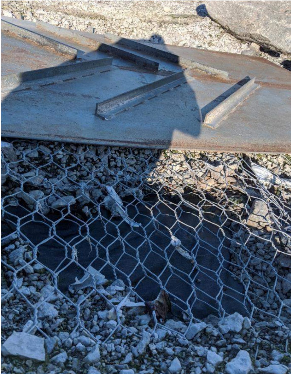
Photograph #2: Gabion baskets have a tendency to empty themselves over time owing to the small diameter of gravel contained within.
