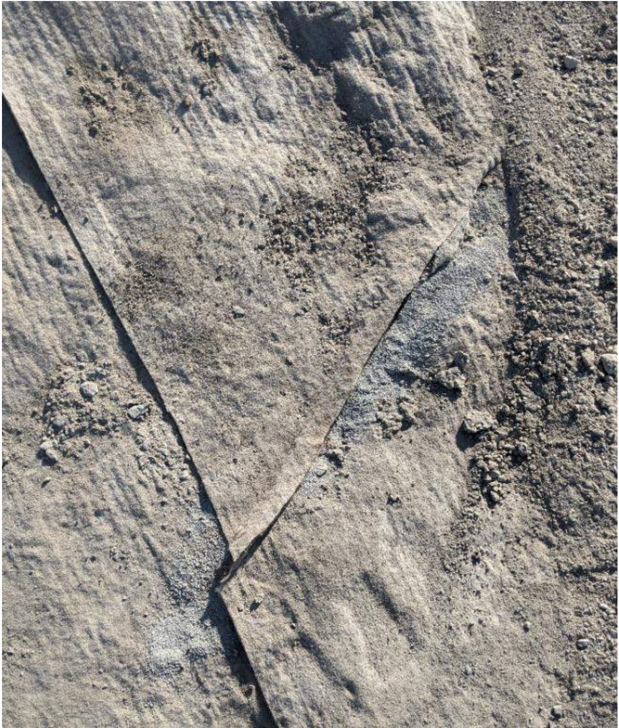
Photograph #3: Some wrinkles and folds were cut out in order to allow the liner to sit flat. The new liner will completely cover these cuts.
