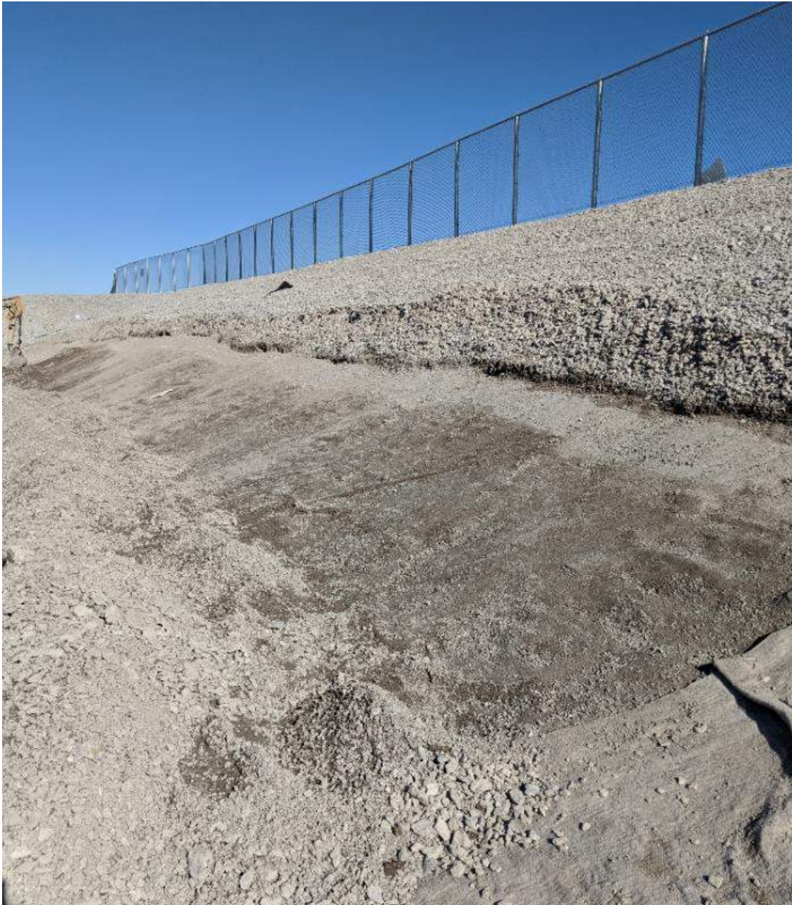
Photograph #1: Clearing of the existing liner along the east embankment, towards the north end of the cell.
