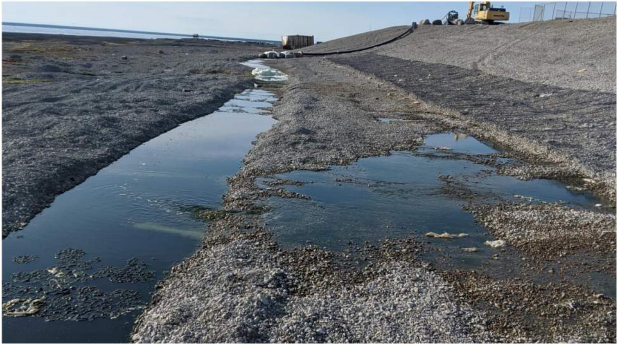
Photograph #1: Significant amount of water is leaking from the east side of the lagoon.
