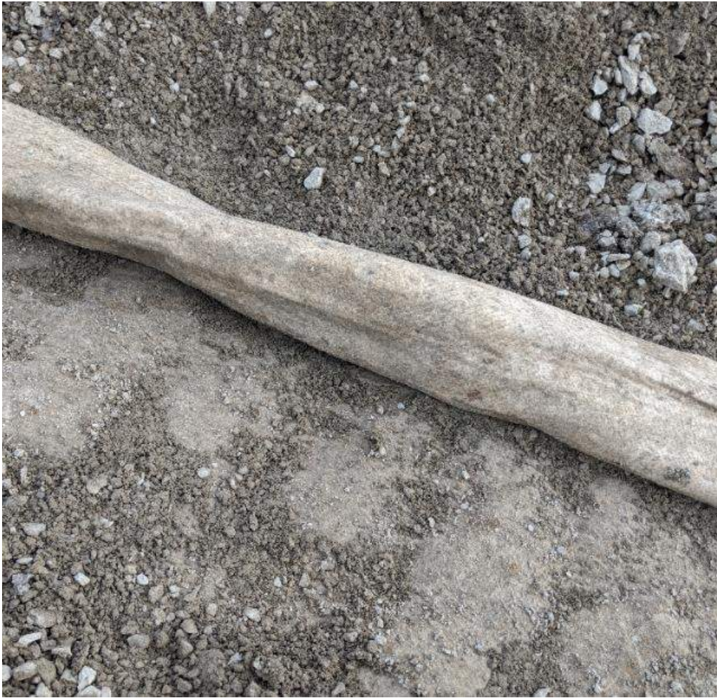
Photograph #3: Gravel was present throughout the width of this portion of the seam. A wider swath of liner will be exposed and the liner will be rolled back further, allowing for a thorough cleaning of the joint. Dozer track pattern still present here.
