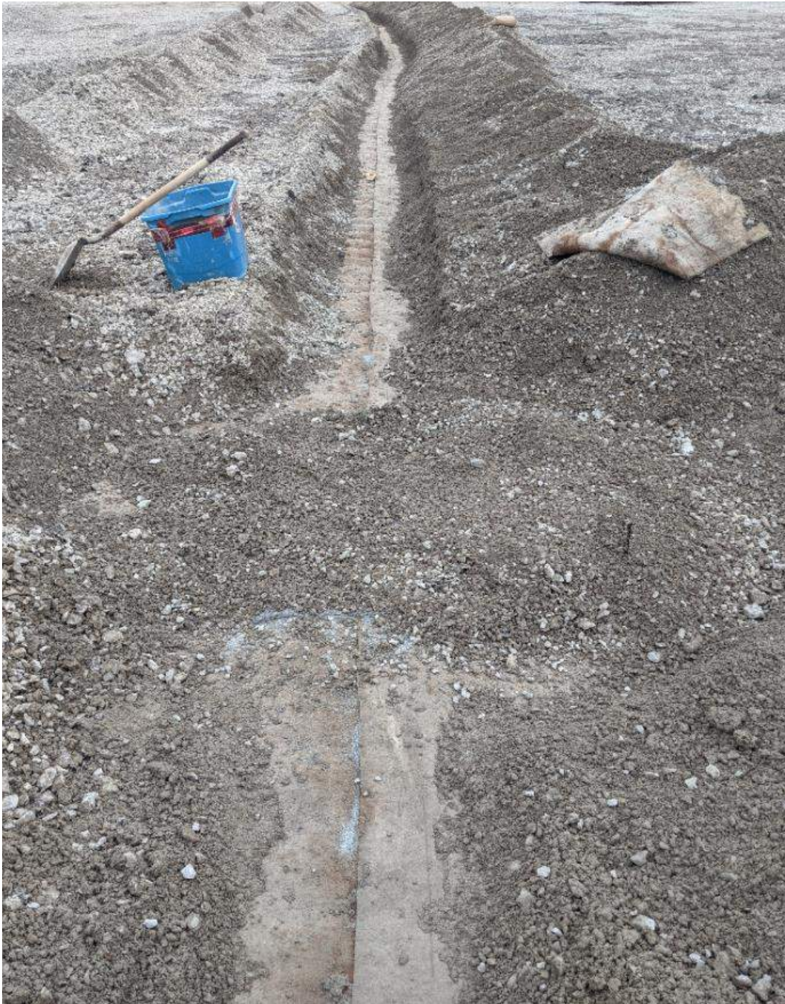
Photograph #2: Installation of patches over damaged areas, including partial backfill to hold the patch down, is being completed as resealing work progresses, with backfilling occurring at the end of the day.
