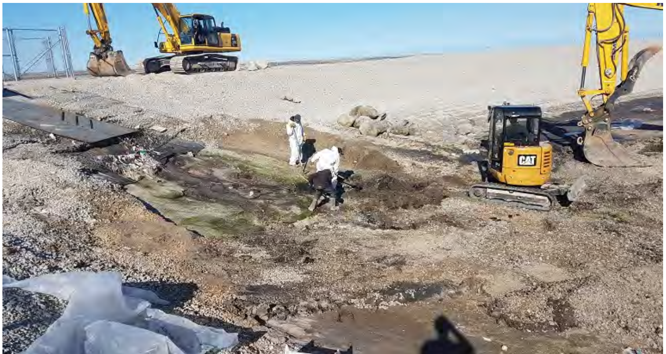
Photo 2: Mini Excavator and labourers removing the cover material above the GCL in the discharge area.
