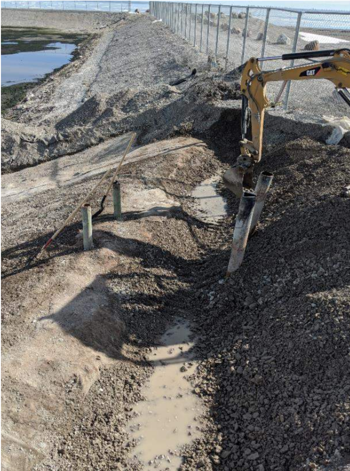
Photograph #4: Anchor trench for new liner is being dug behind existing anchor trench.
