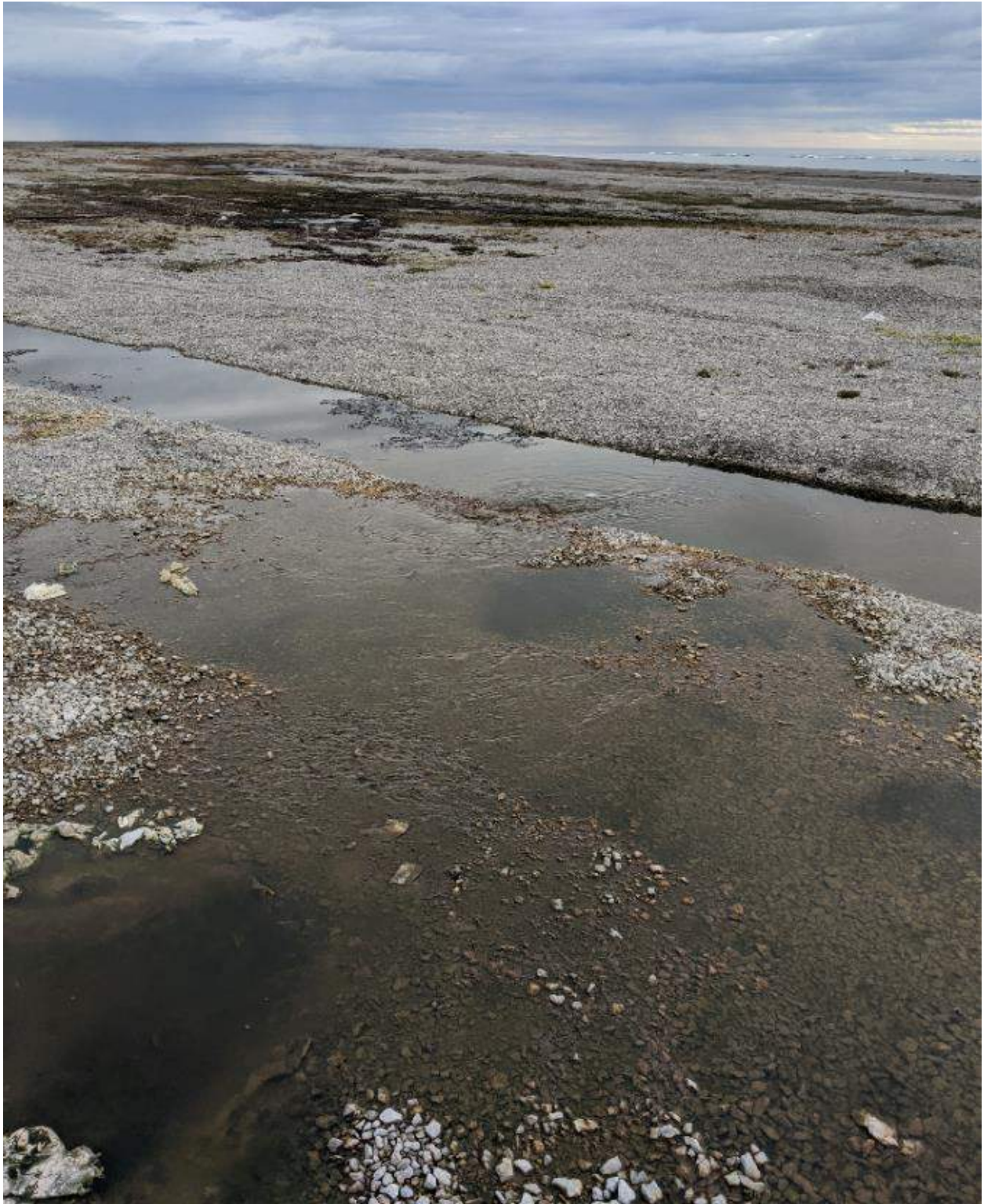
Photograph #4: Leak at east side of lagoon's south cell is still flowing at a significant rate.
