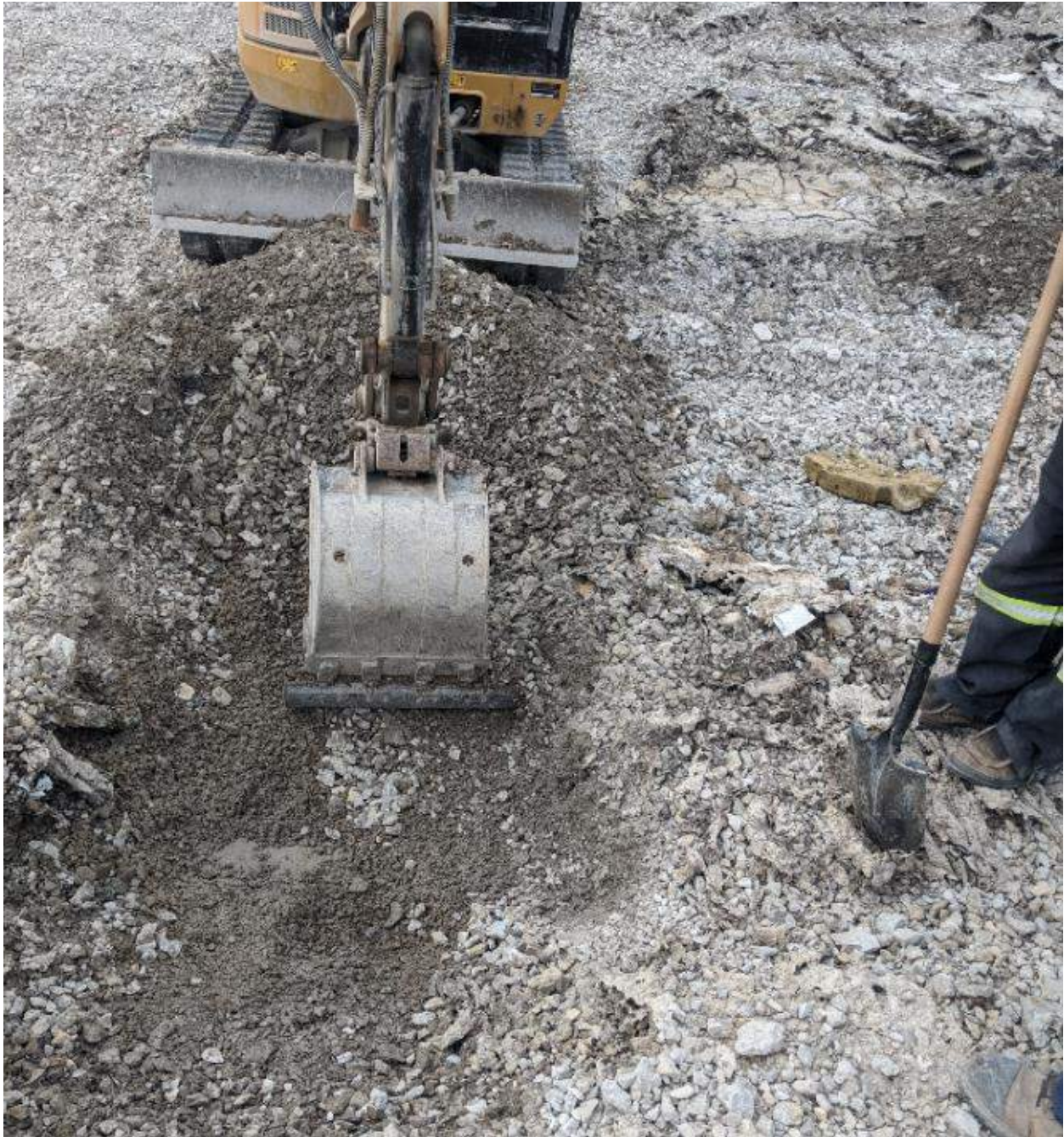
Photograph #2: Exposing the liner seams on the south berm of the south cell. No defects were found in any of the seams on the south berm.
