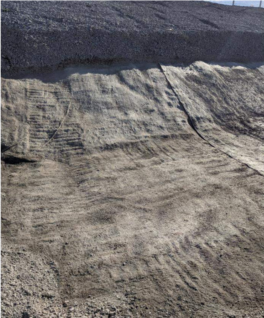
Photograph #2: Evidence of equipment having travelled on the liner. By the shape and width of the imprints, it is suspected to have been an excavator.
