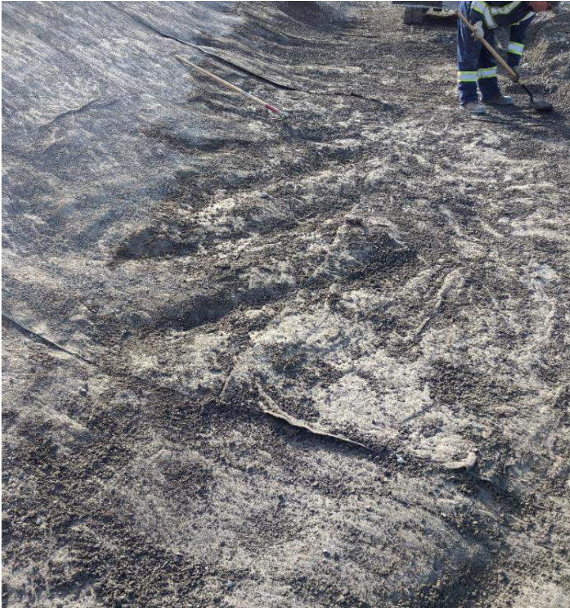
Photograph #1: Subgrade forming a wave pattern along the bottom of the cell.
