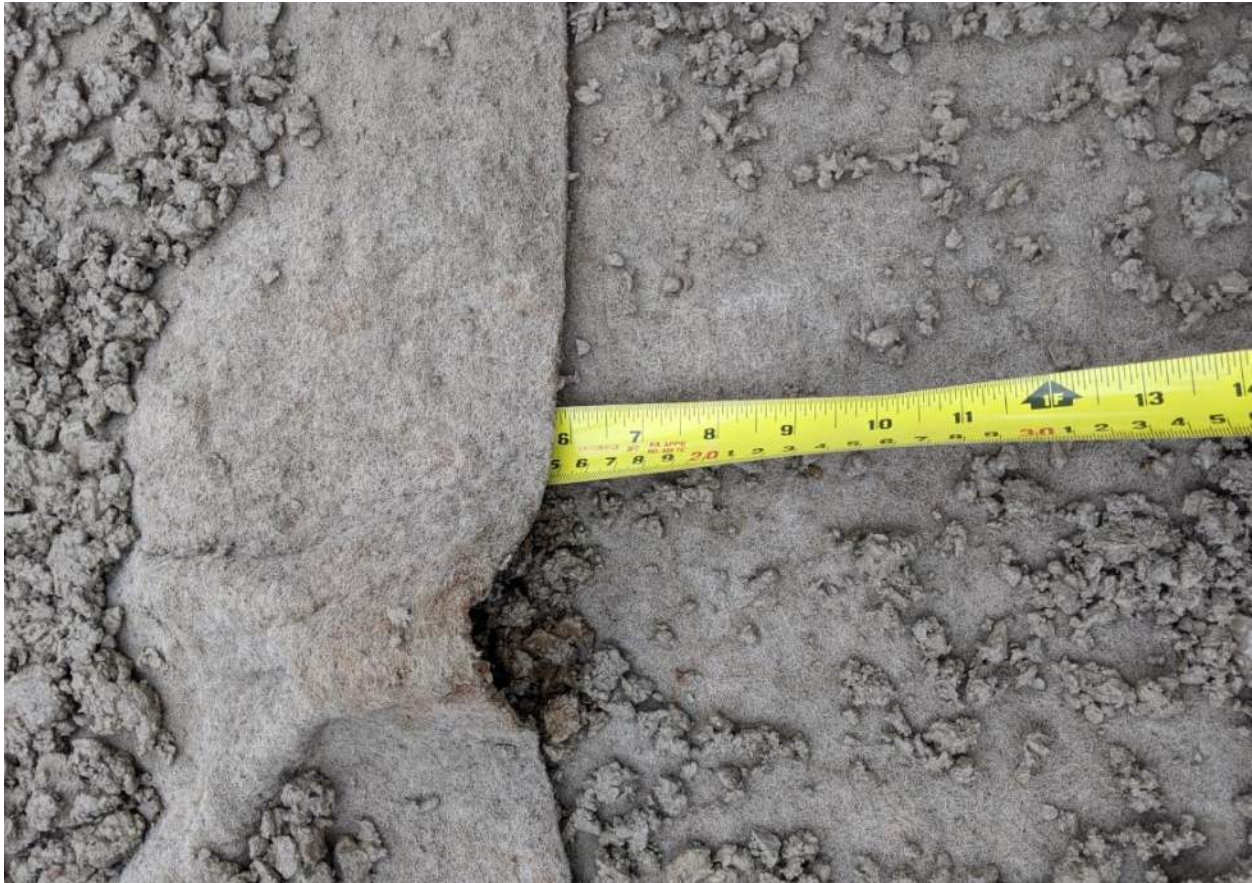
Photograph #4: Narrow lap distance in one of the inspected seams. Manufacturer recommends at least 200mm lap distance.
