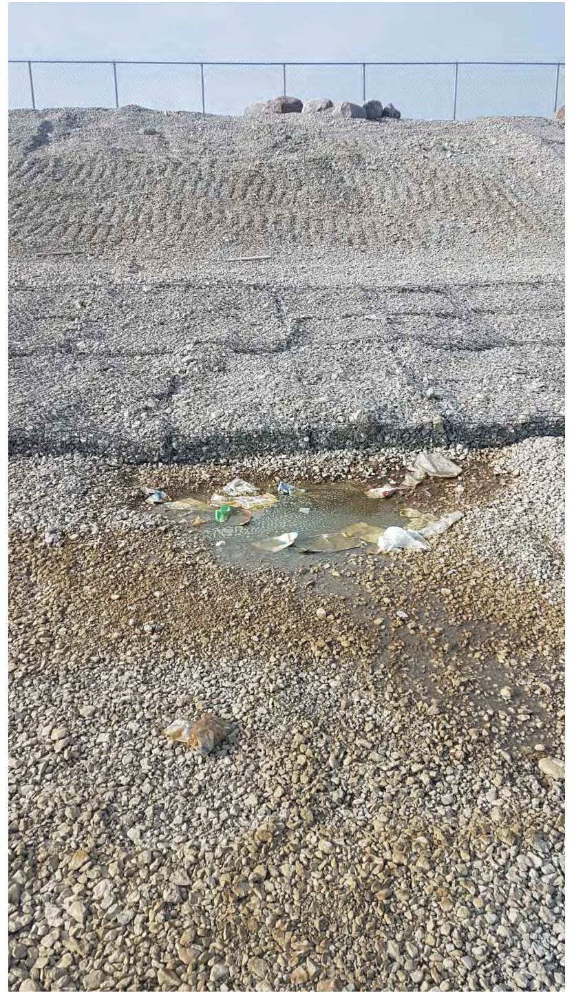
P4 DETAIL PHOTO - SEEPAGE OBSERVED AUGUST 2018
