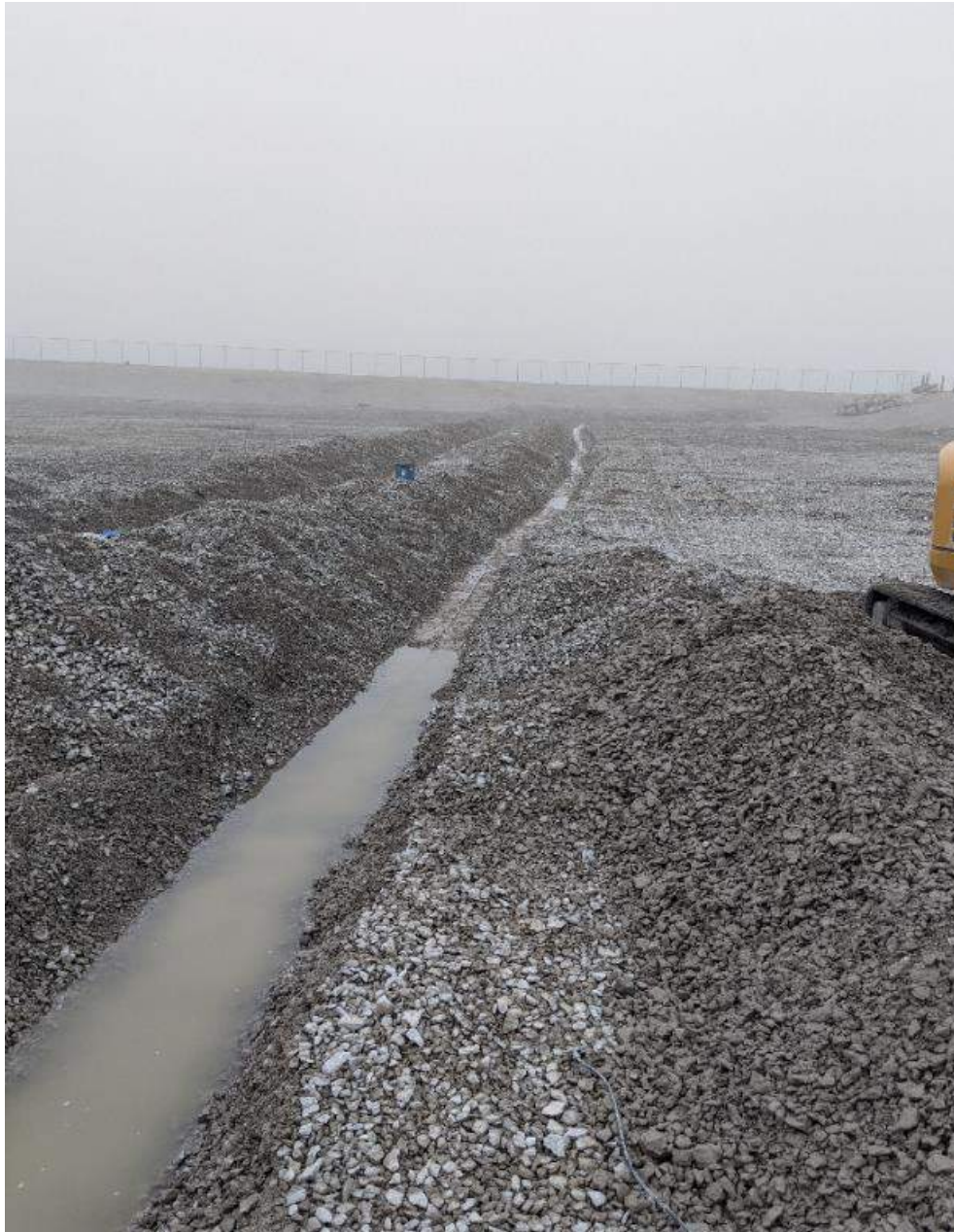
Photograph #1: Seam exposure in the east-west direction. Heavy rain all day caused water to pool in the exposed area.
