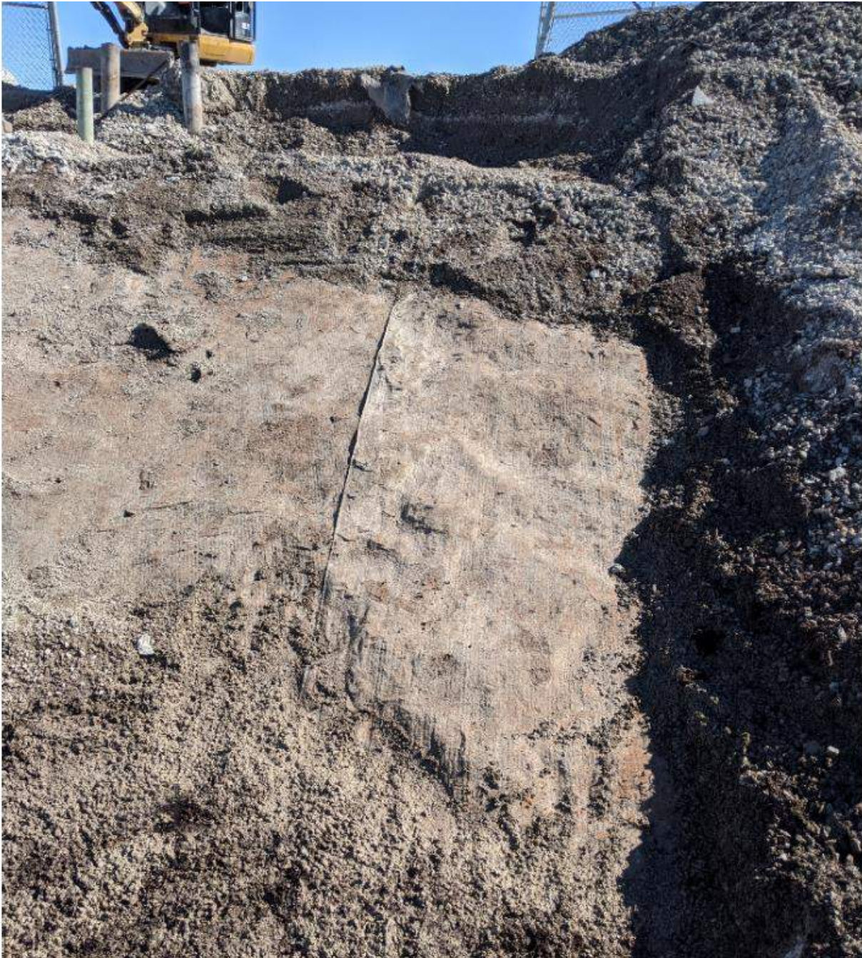
Photograph #3: Seam within existing liner. New liner will be glued to existing liner using bentonite as per manufacturer's instructions. Existing liner will be cleaned off with broom at location of seam prior to applying bentonite.
