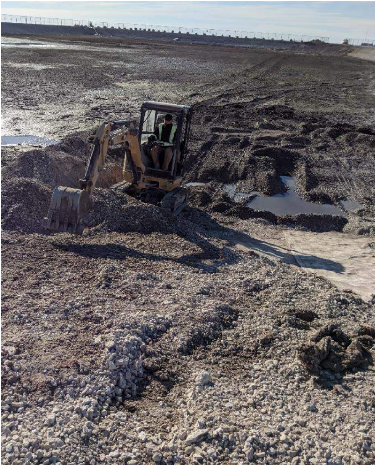
Photograph #1: A thin layer of granular material was left on the liner until dried. This allowed the liner to recover some of its structural strength before being exposed.
