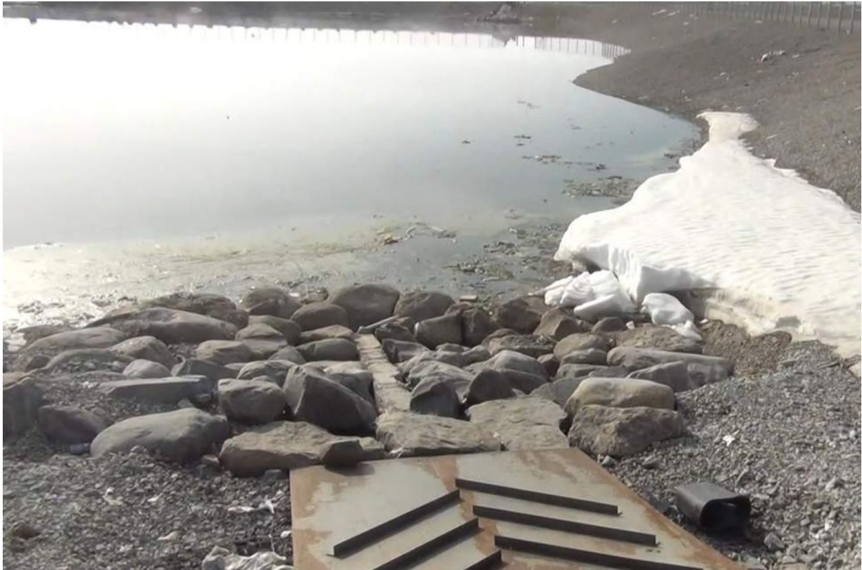
Photograph #5: North discharge station. Very few fines between large rocks, concrete slab running down centerline of discharge path quite apparent.
