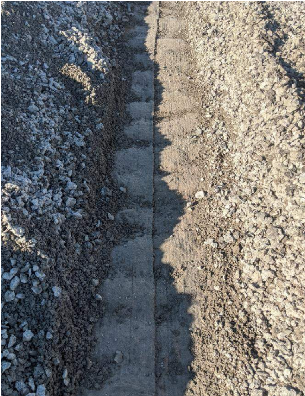
Photograph #2: Dozer tracks over the joint.
