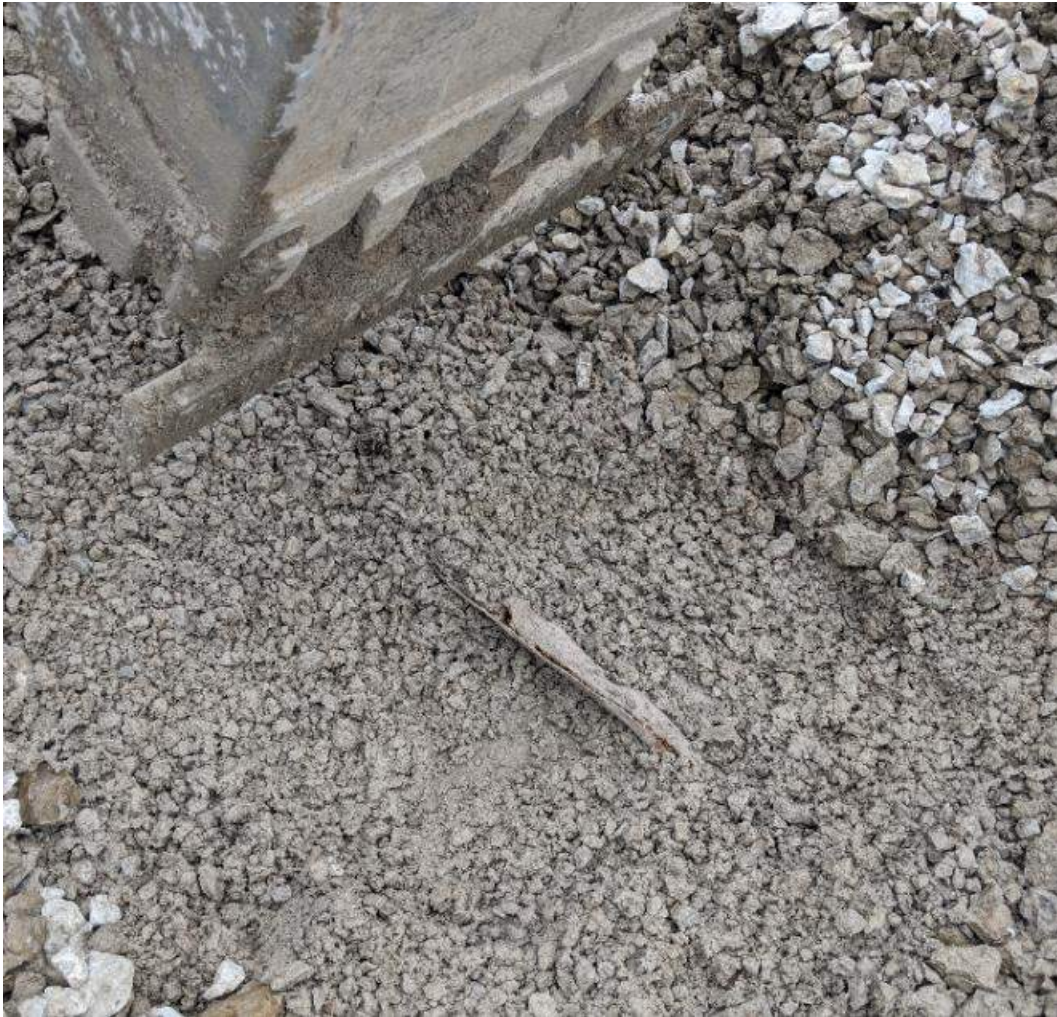
Photograph #3: Liner edge sticking straight up as it is uncovered. The bottom side of the liner (lower left side of liner as seen here) is full of gravel, preventing the seam from properly closing.
