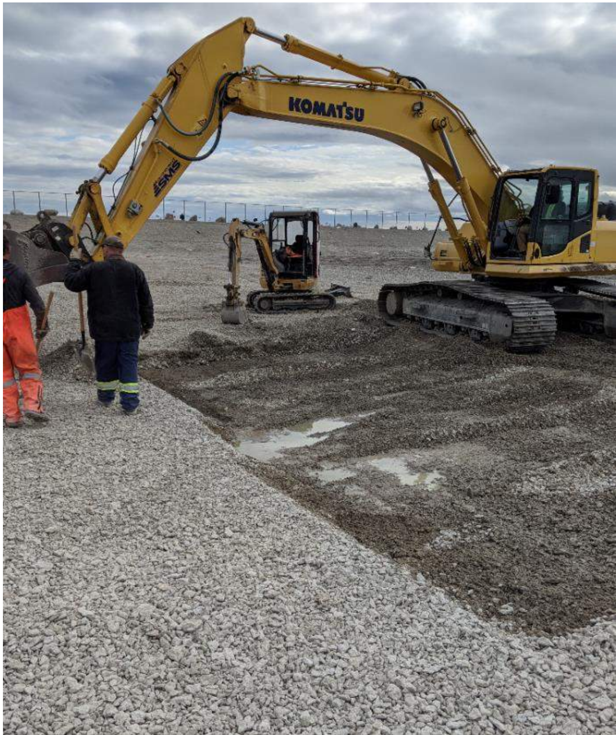
Photograph #3: Exposing liner to check for leaks.
