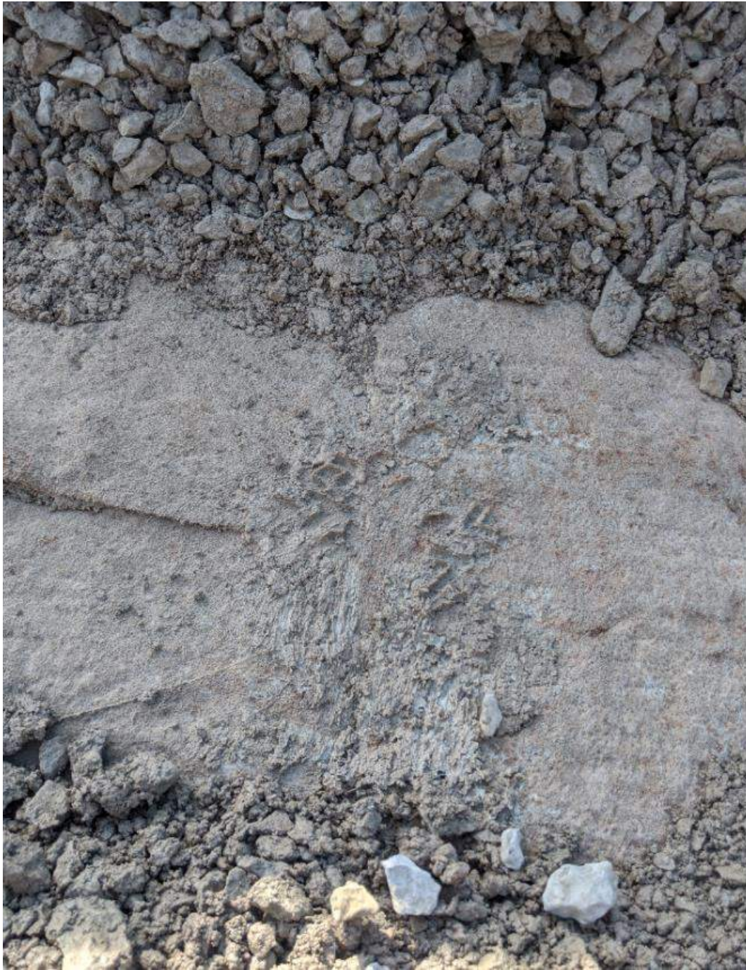
Photograph #1: Bentonite being squeezed out of the joint around a patch.
