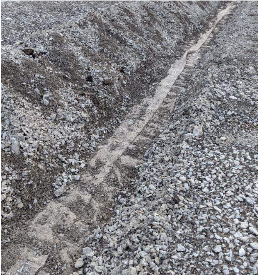
Photograph #2: Dozer track pattern along seam. Liner on right hand side was imprinted deeper than its counterpart, allowing gravel to slip between the liners.
