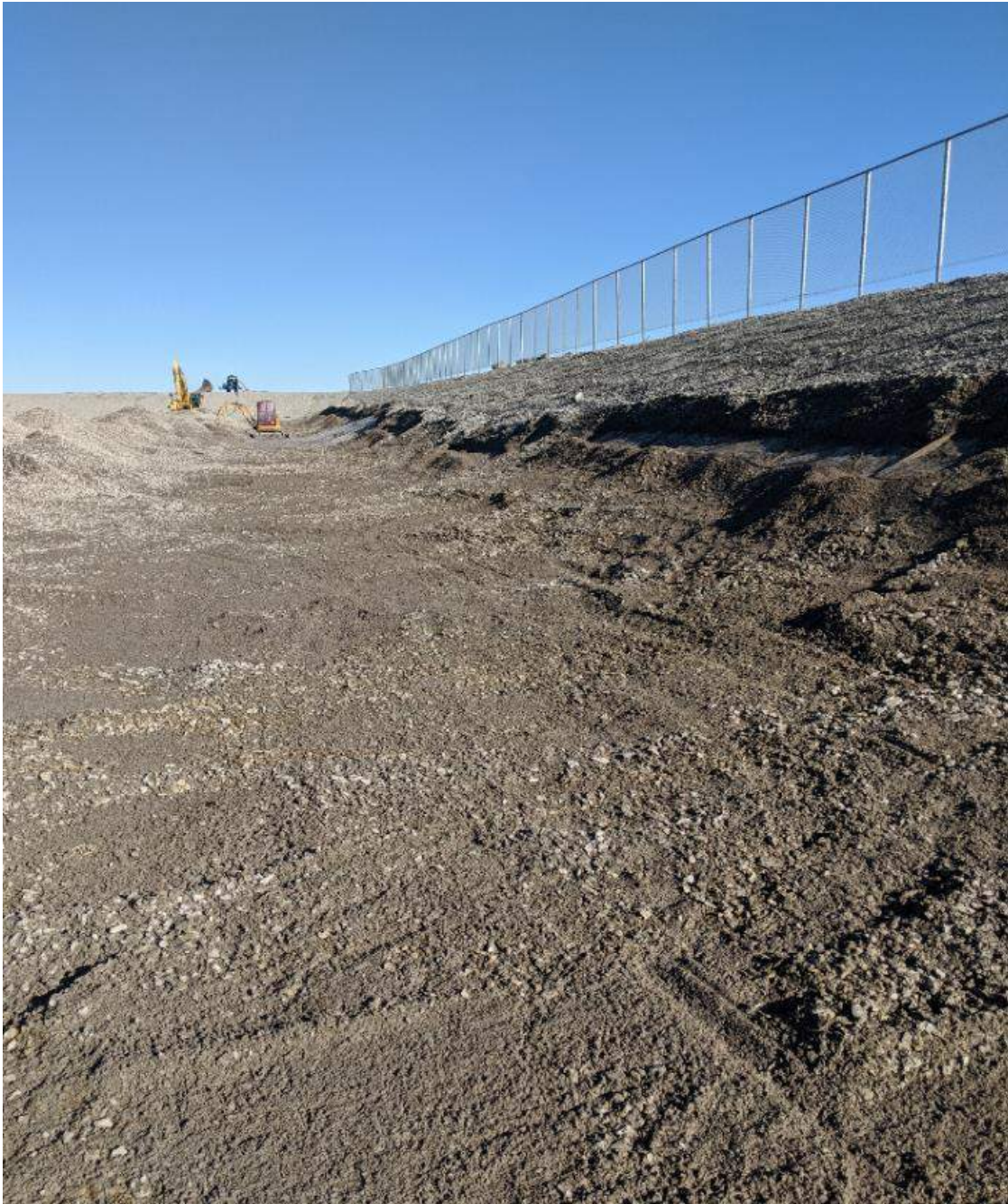
Photograph #1: East bank, with most of the aggregate layer removed, leaving only the sand layer.
