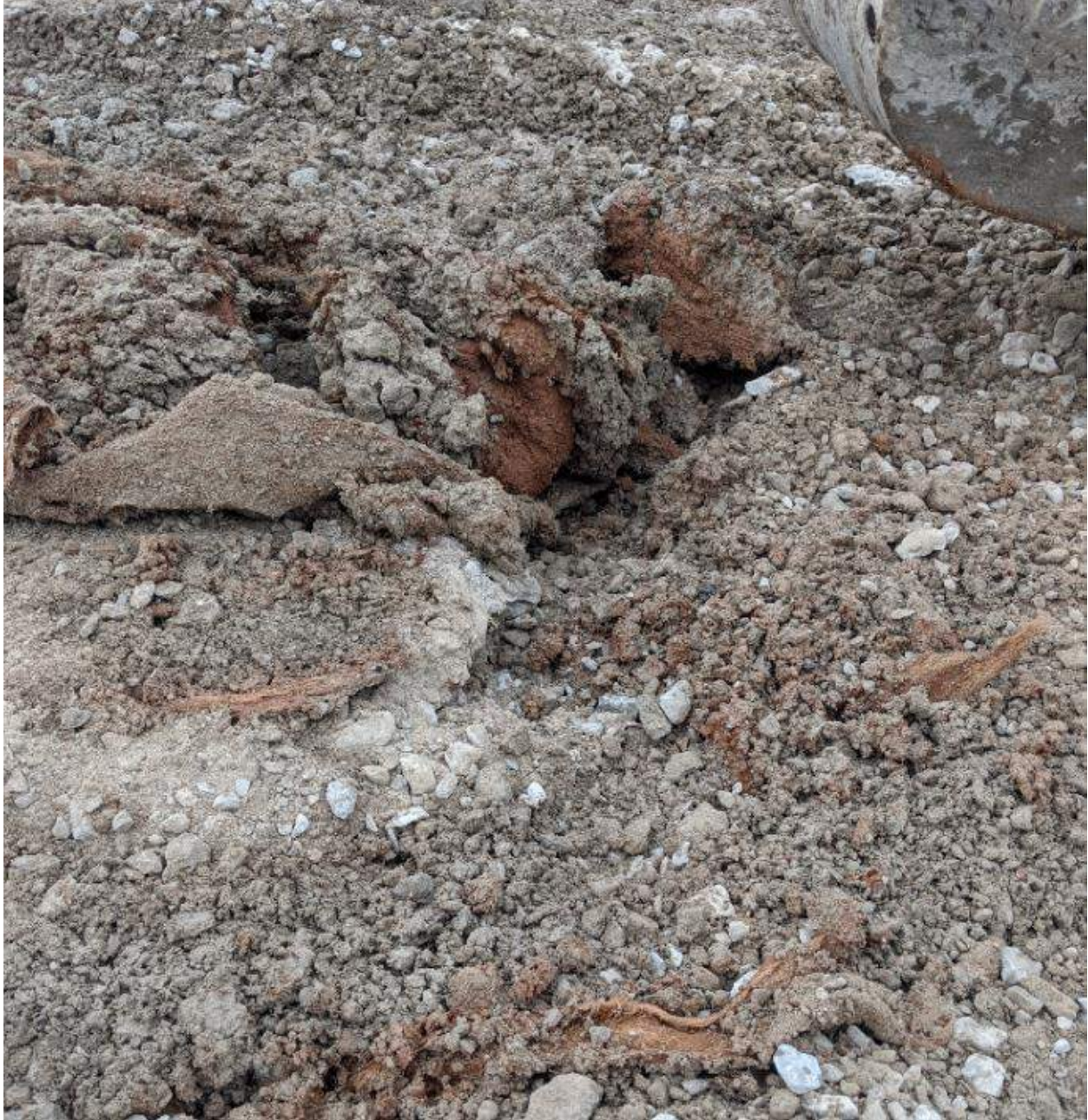
Photograph #7: Liner in some areas at the north discharge station is rolled and torn, and no longer sealed to underlying liner.
