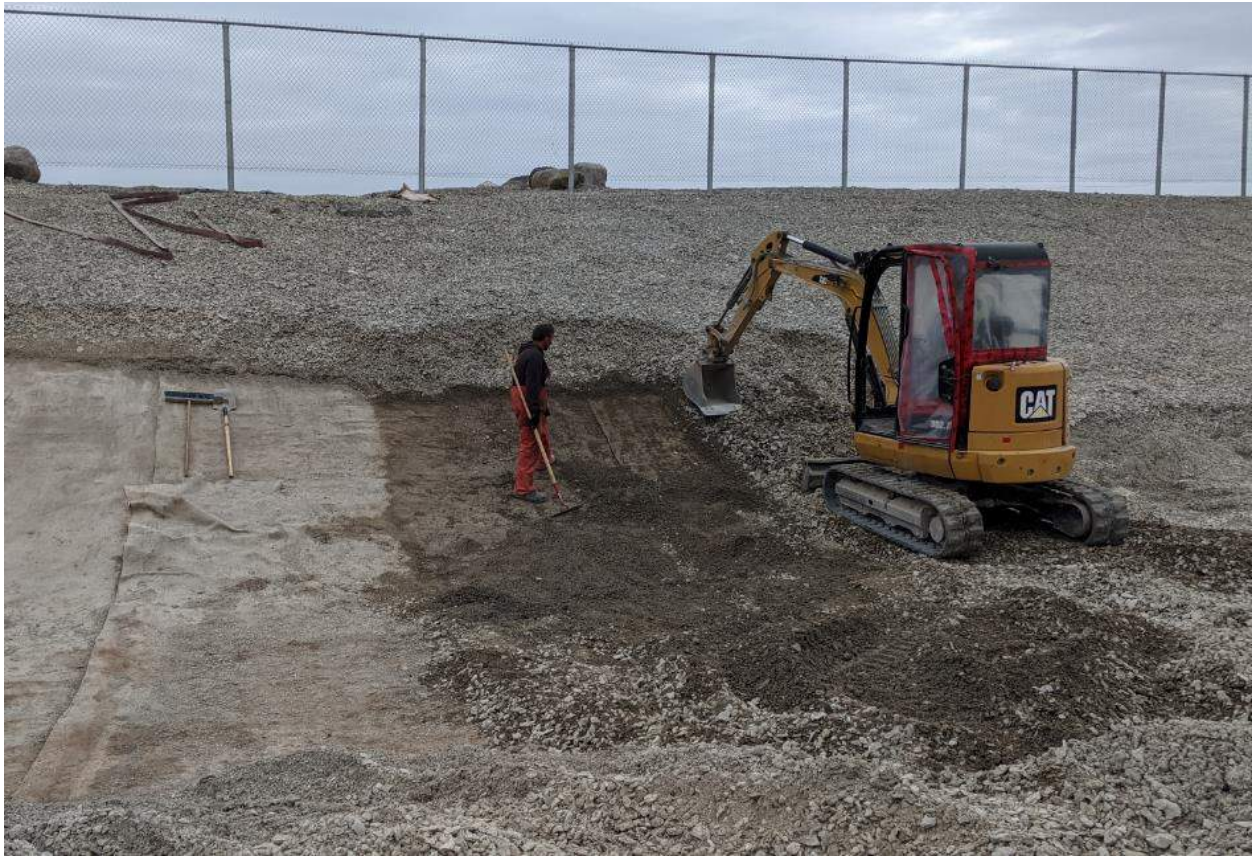
Photograph #1: Liner exposure operations continue along the east bank.
