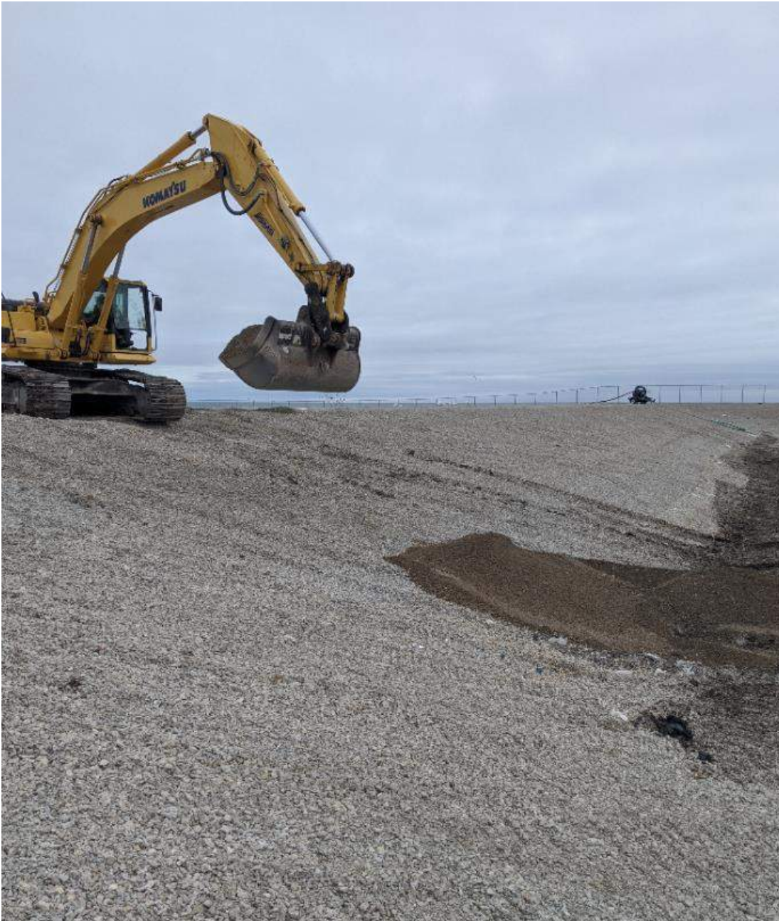
Photograph #3: Sand was lowered into the lagoon using the excavator, rather than repeatedly driving equipment down the slope, which could damage the underlying liner.
