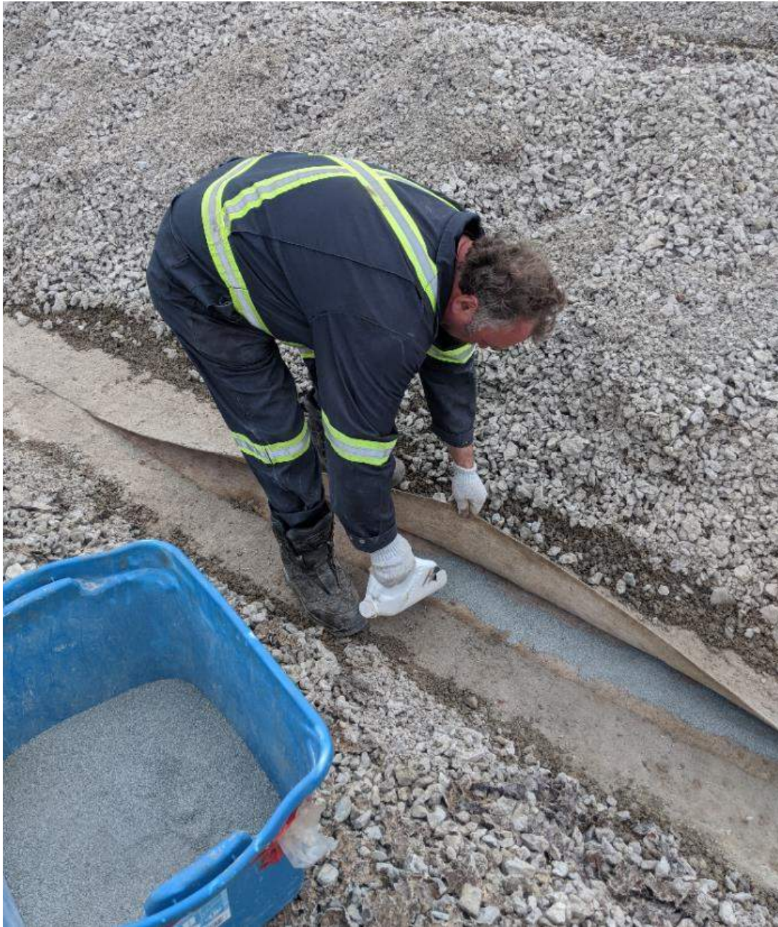
Photograph #1: Placing bentonite within the seam, in a strip running parallel to the existing strip (further into the seam, not visible in this photo).
