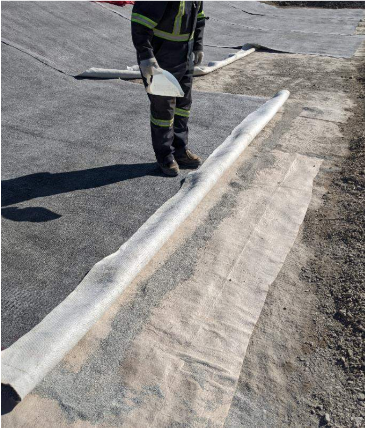
Photograph #1: Sealing the liner seams with bentonite.
