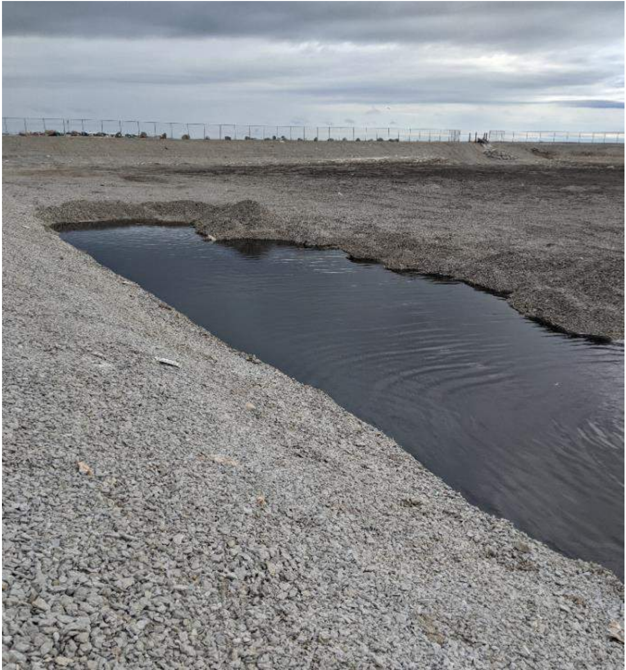
Photograph #3: Flooded lagoon as of the end of the day. Water depth is approximately 0.6m at the deepest.
