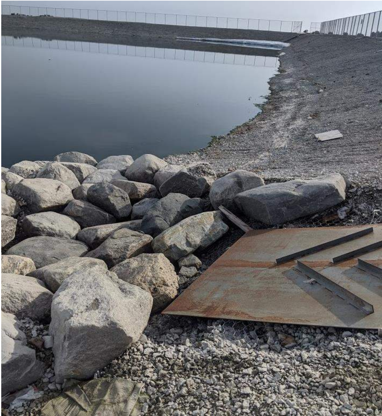
Photograph #2: South discharge station, showing significant erosion of fines between larger rocks.
