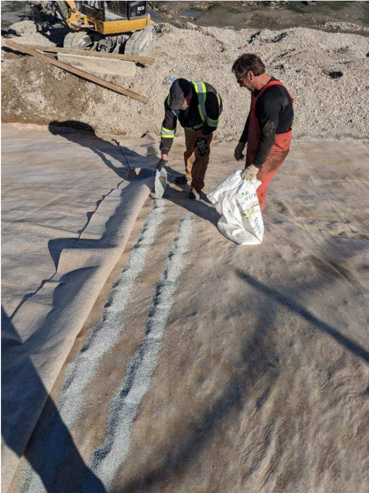
Photograph #2: A double line of bentonite was used to seal liner at the edges.
