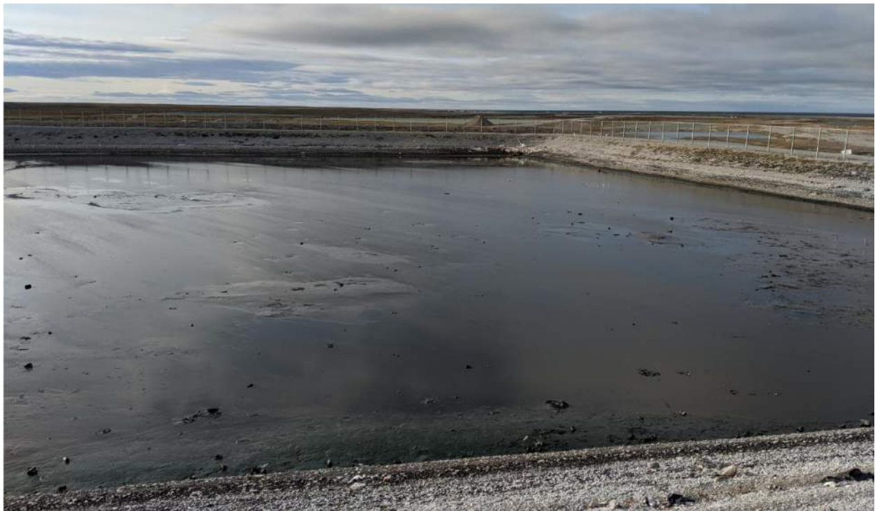
Photograph #4: The North cell is rapidly depleting, and the bottom is visible in most of the cell.
