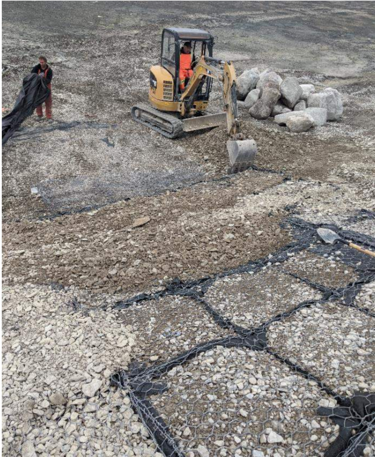
Photograph #2: The day was spent installing gabion cages at the south discharge station.
