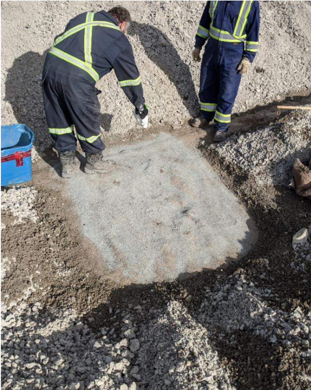
Photograph #2: Ample bentonite was applied to this patch, which replaces the patch placed in 2018.
