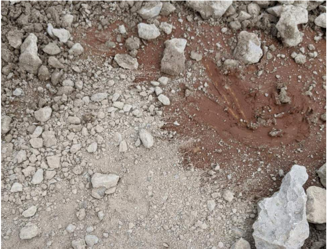
Photograph #6: Liner in some areas is delaminating, with the frayed and worn top geotextile coming apart to expose the bentonite within the liner. In areas where this is occurring, a new liner will be placed.
