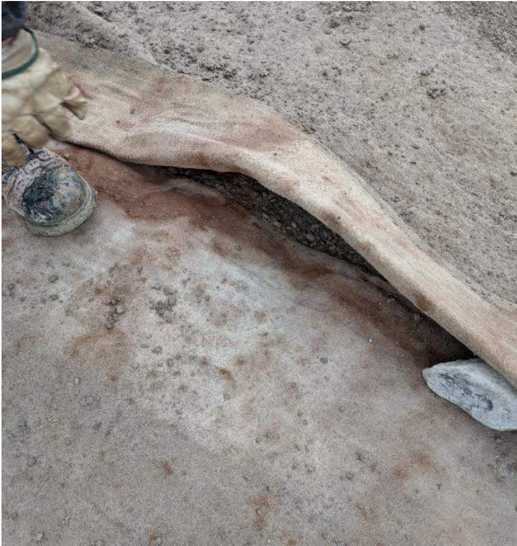
Photograph #1: Non-continuous bentonite strip within seam.
