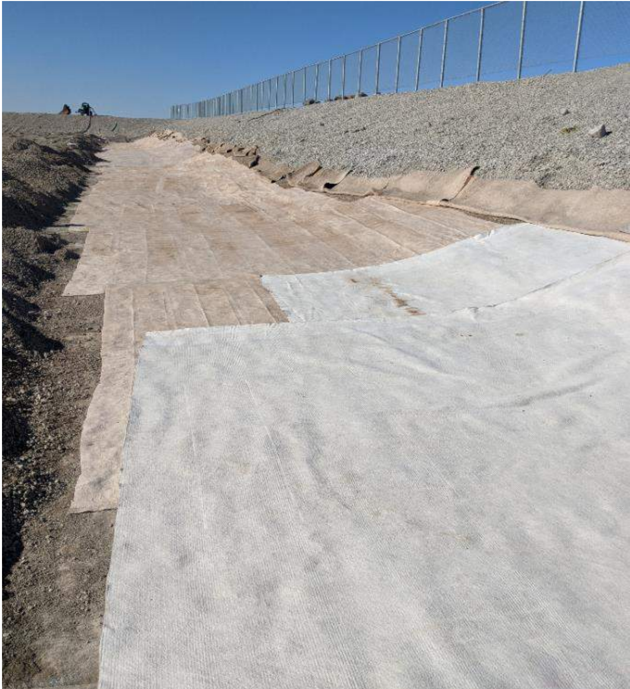
Photograph #5: The final panels of the new liner are a different material than the rest of the panels. The new material is from a different shipment, and is approximately twice as thick as the rest of the liner.
