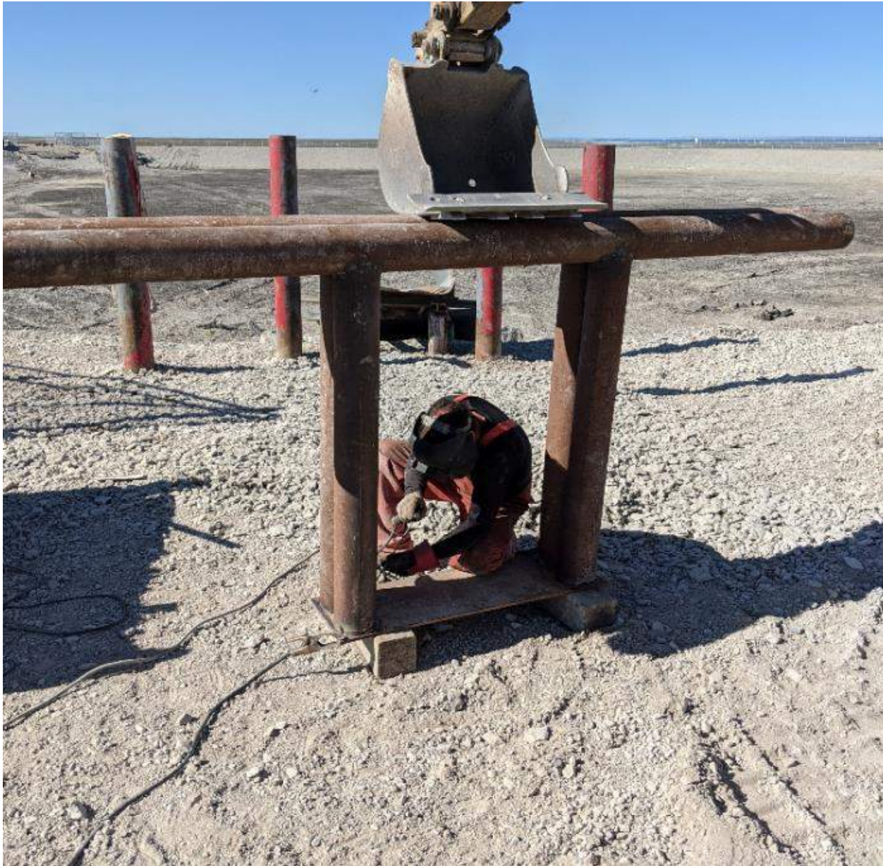
Photograph #2: Welding the truck bumper onto the 12 mm steel plate that will in turn connect to the discharge station piles.
