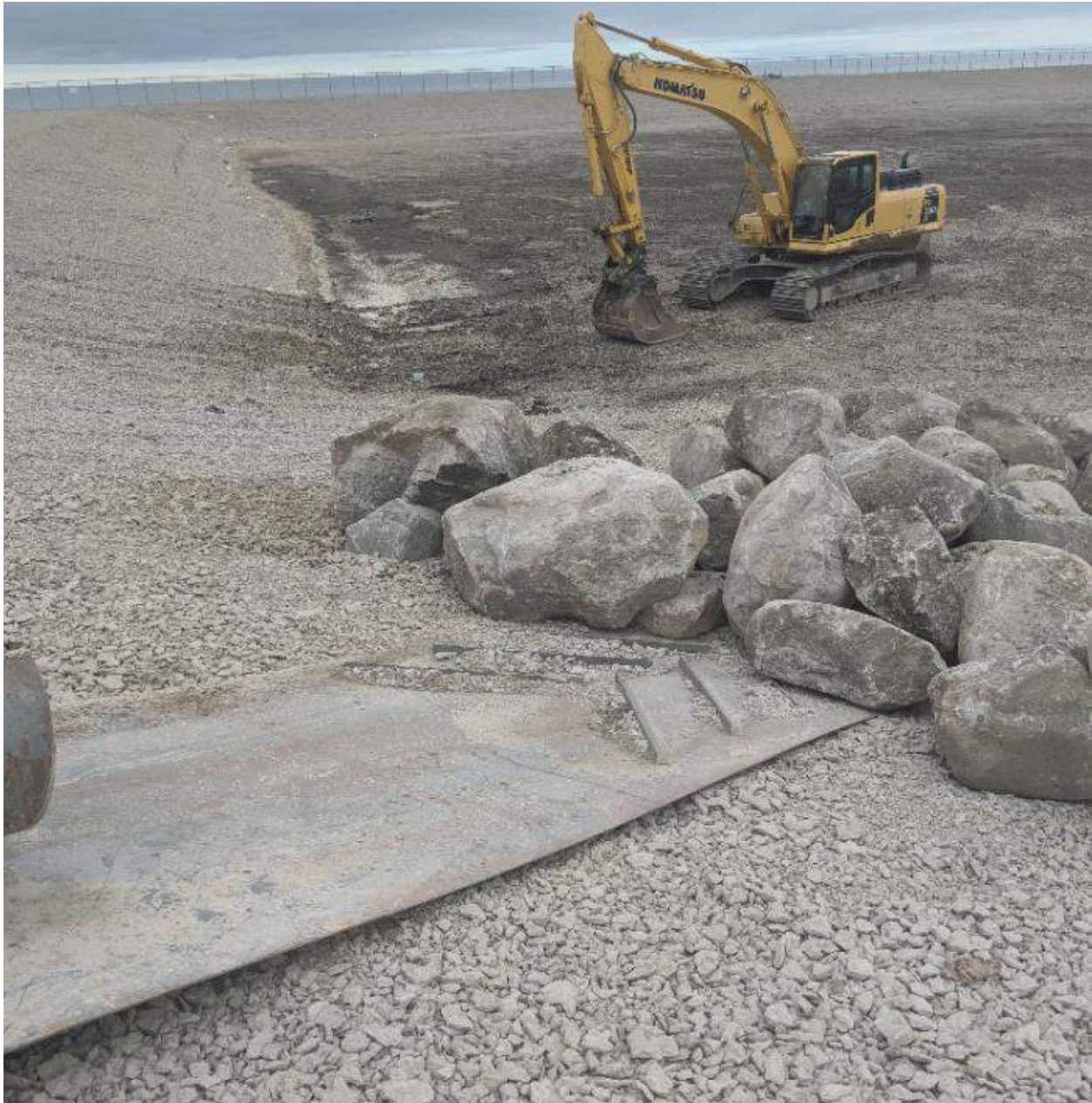
Photograph #2: Riprap placed at the bottom of the chute.
