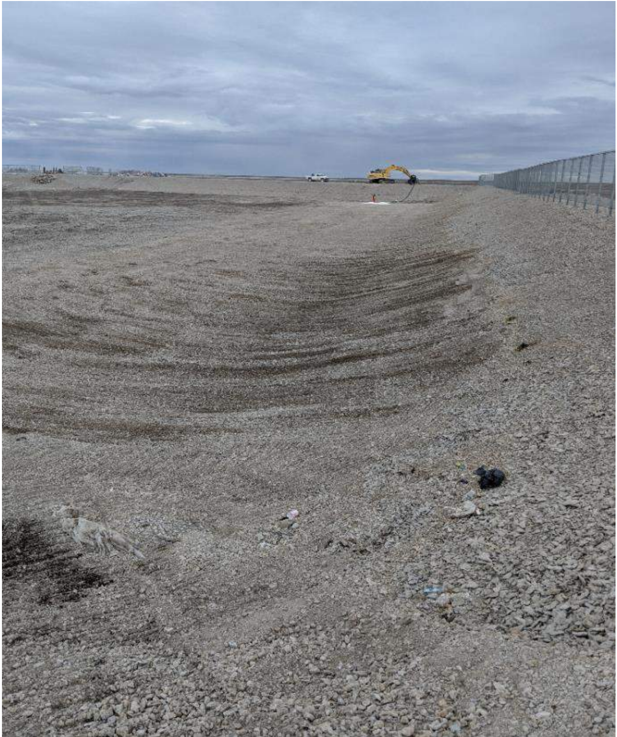
Photograph #1: Completed backfill of new liner along east berm.
