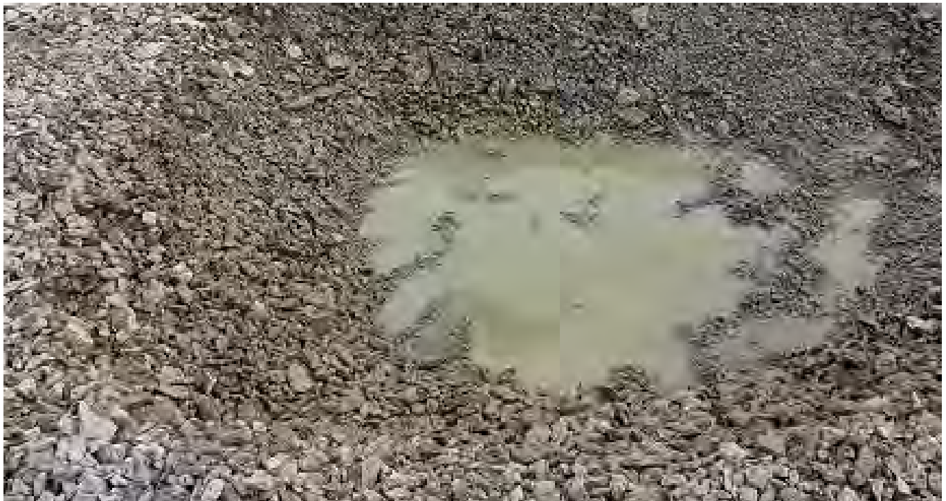
Photo 4: Area 4 during excavation. Cover material underlain by a coarse sand, with about 100mm of liquid before the GCL.
