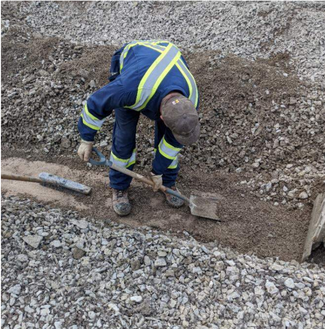
Photograph #2: A mini-excavator is used to remove most of the aggregates, the sand layer is removed by hand, and a broom is used to clean off the liner.
