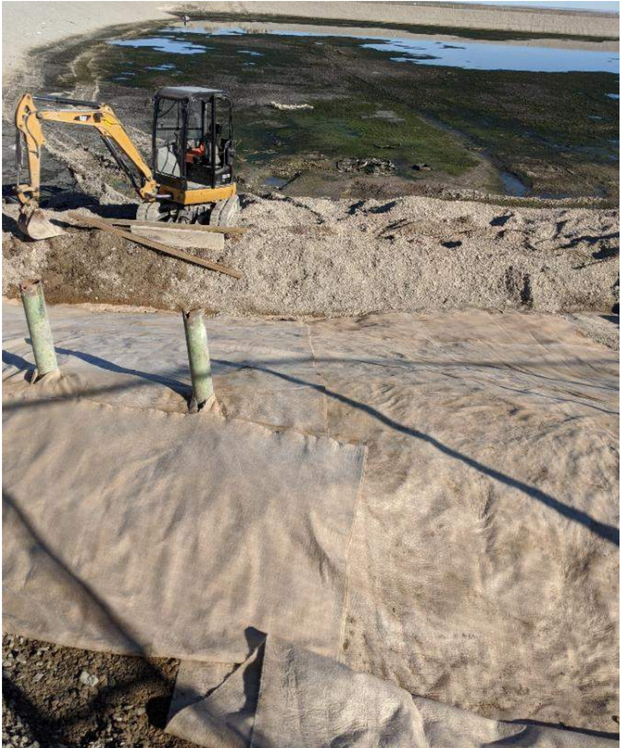
Photograph #1: Liner was placed on embankment and tucked into anchor trench. Excess material was trimmed before burial.
