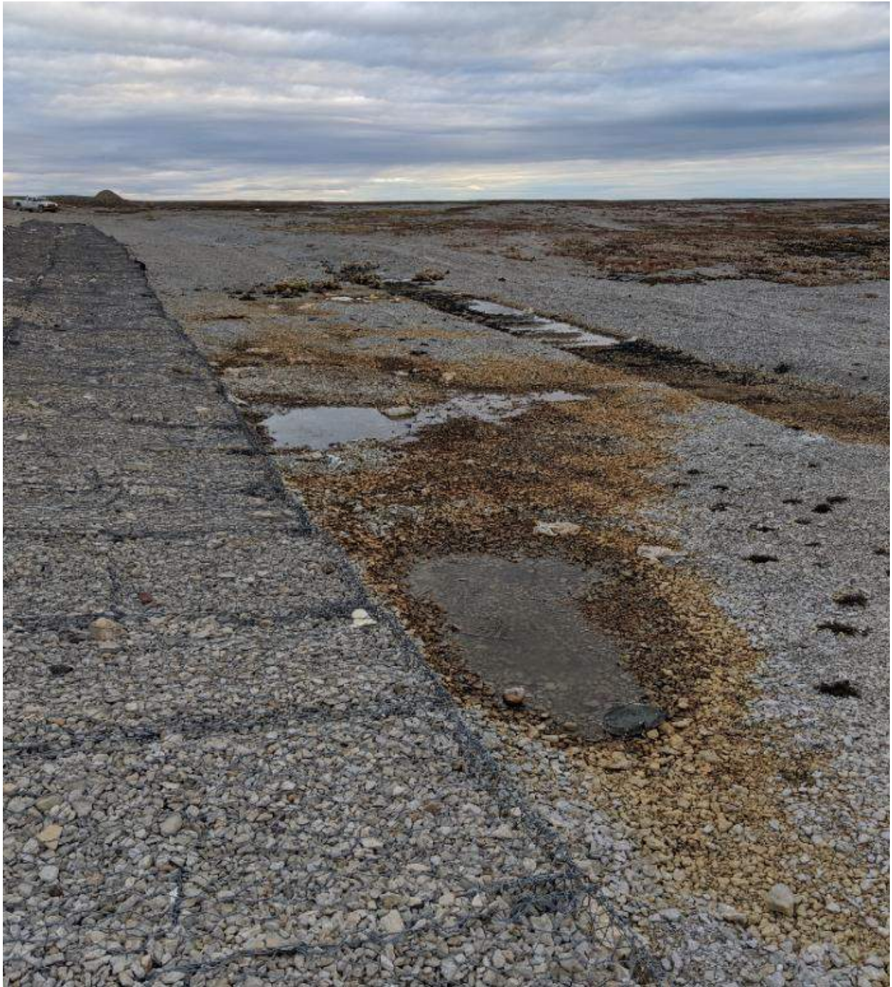
Photograph #1: New leak noted at the location of previous leak.
