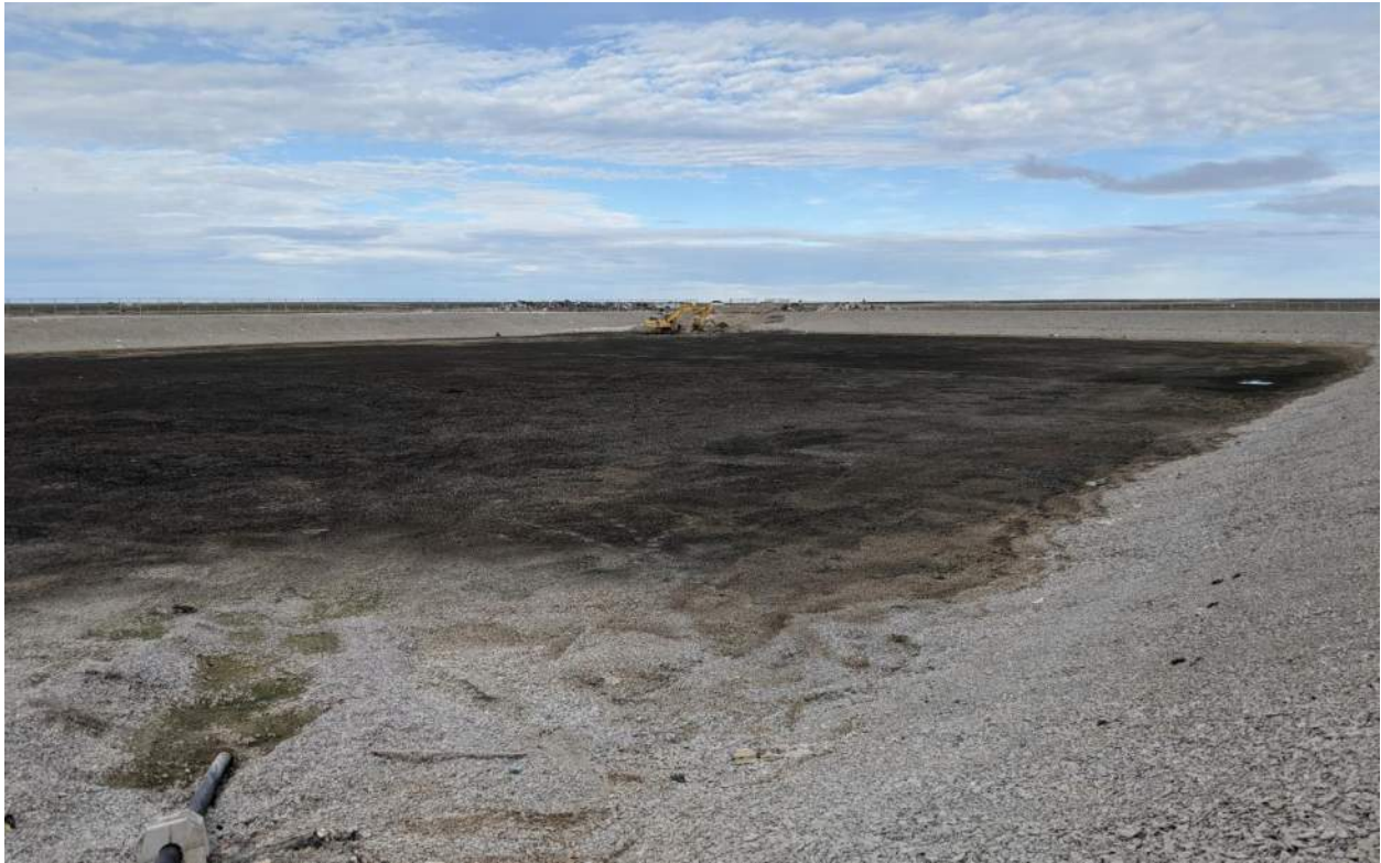
Photograph #1: Apart from a very small puddle, the lagoon cell is now completely empty. Note that there is still >300mm of water in much of the cell, above the liner but below final grade.
