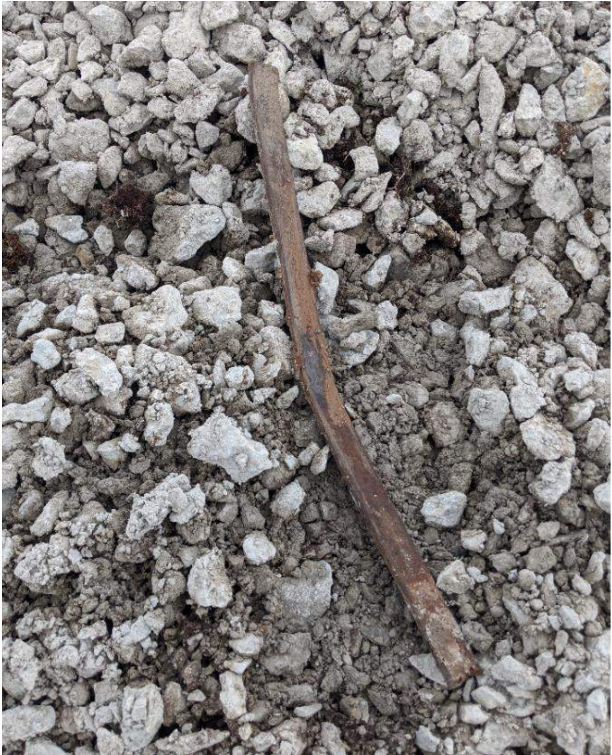
Photograph #2: Piece of steel found within a seam during excavation and removed. Length is approximately 40cm.
