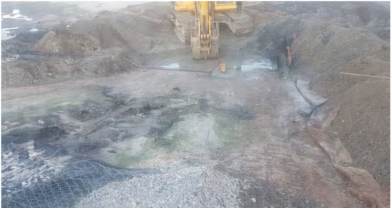
Photo 3: Limits of excavation on August 29. Seams on right side of photo had about 150mm of granular between layers, with no evidence of bentonite. Repairs to GCL evident in this area.
