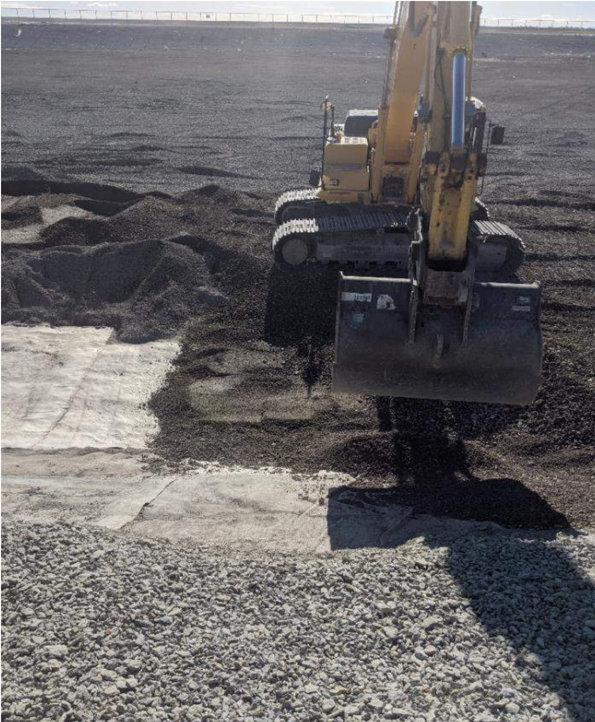
Photograph #2: Sand was placed onto the liner using the excavator. The excavator did not travel onto the liner or the sand layer and did not travel onto the embankment even once the aggregates had been placed down.
