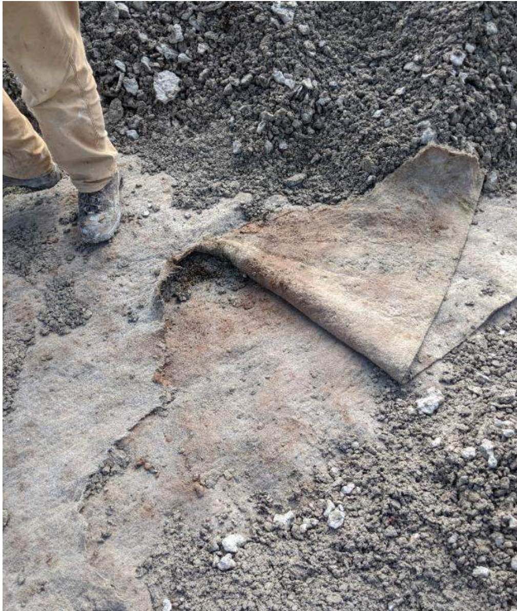
Photograph #1: Tear in the liner. While the flap has been cleaned and unfolded in this photo, the patch of subgrade visible at the back of the tear was found completely uncovered., allowing water a direct pathway into the subgrade.
