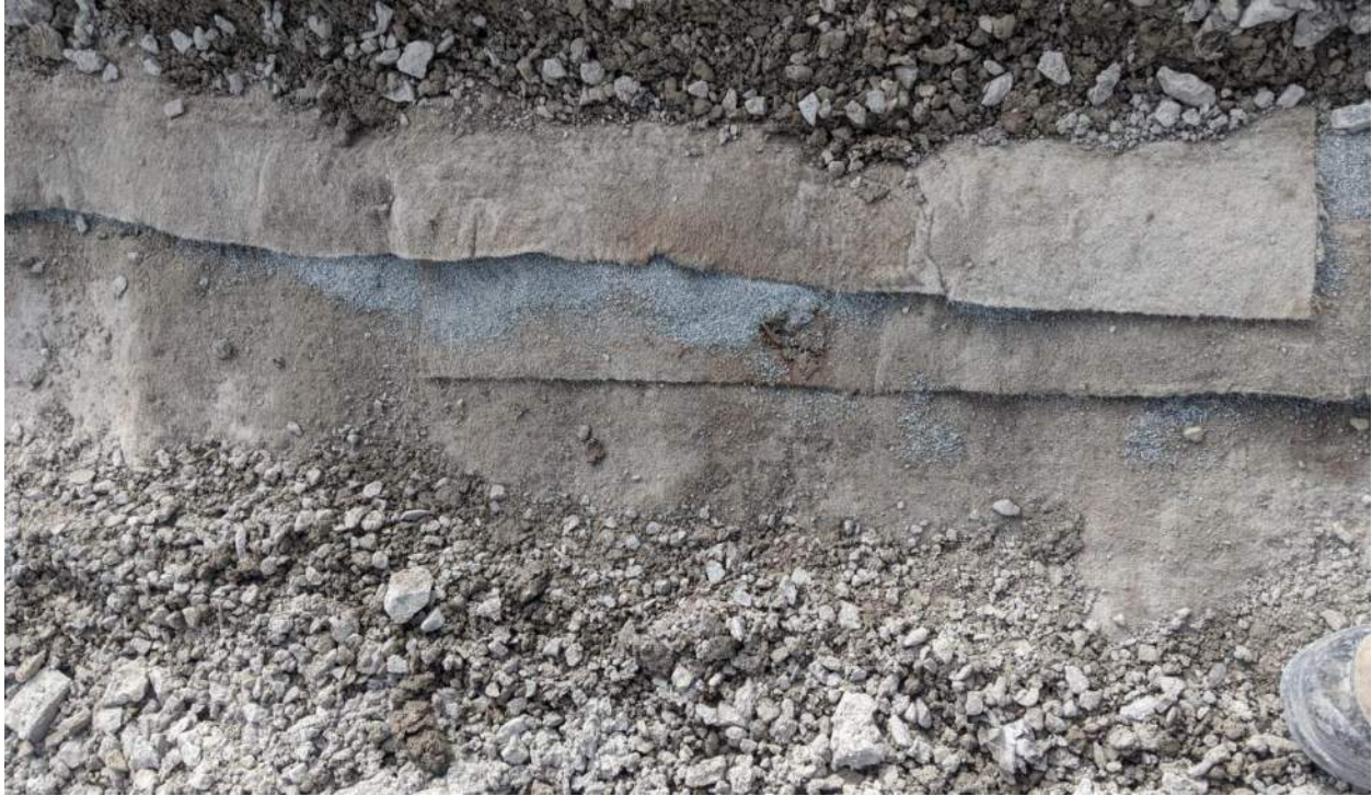
Photograph #2: In areas where multiple layers of liner are stacked, all layers are being re-sealed with bentonite.
