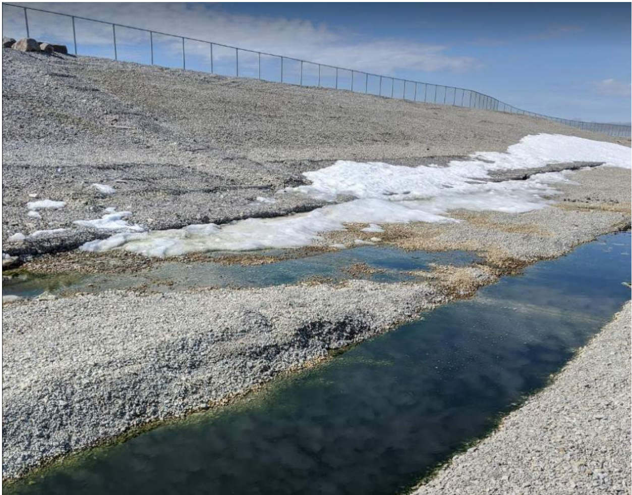
Photograph #1: Potential leak at east side of lagoon.
