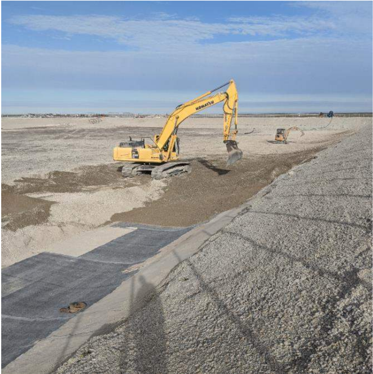
Photograph #1: Covering the newly installed liner with sand, then aggregates.
