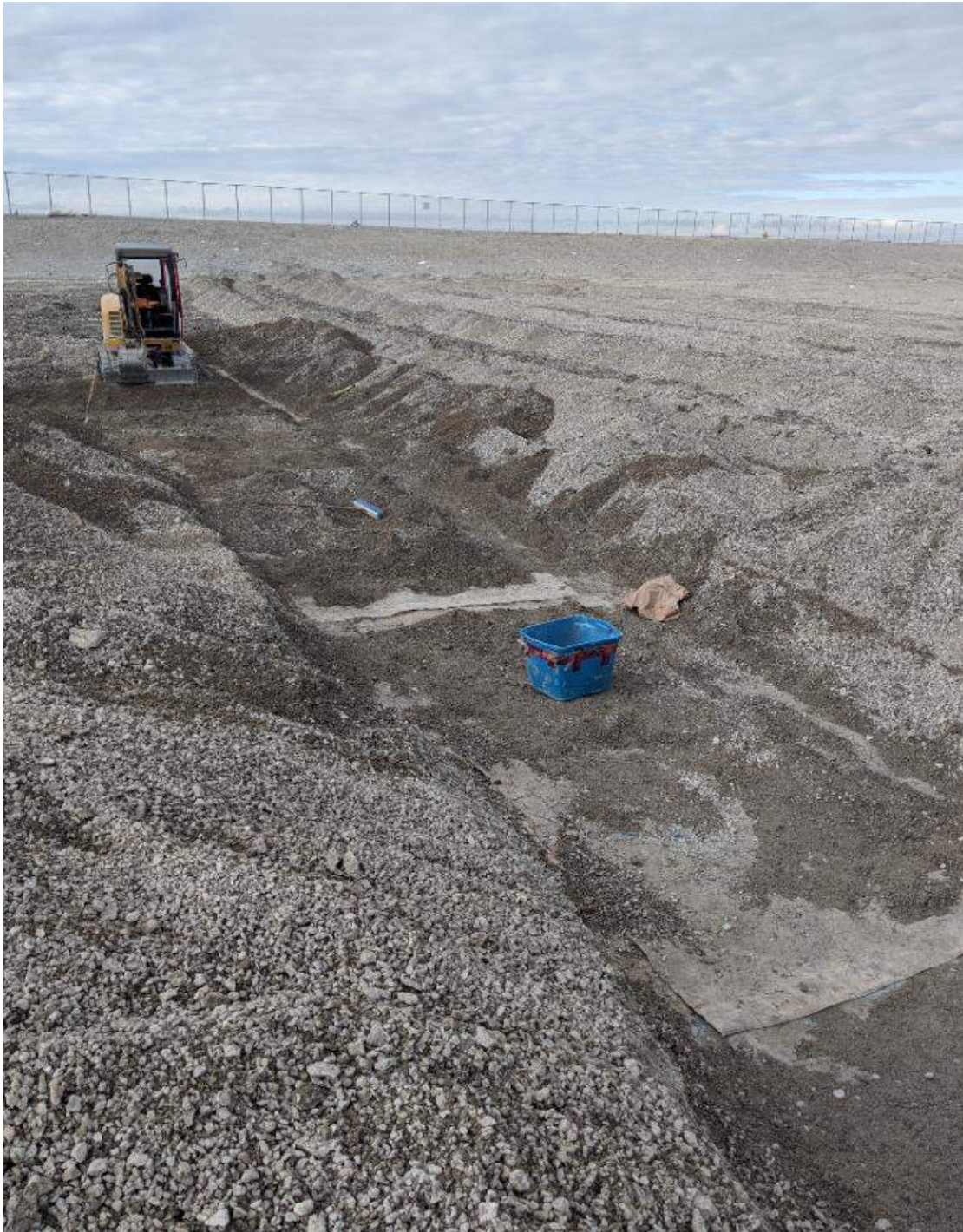
Photograph #2: Patches bridging the gap over the widening divergence between two liner panels. The patches get wider as they get closer to the west bank.
