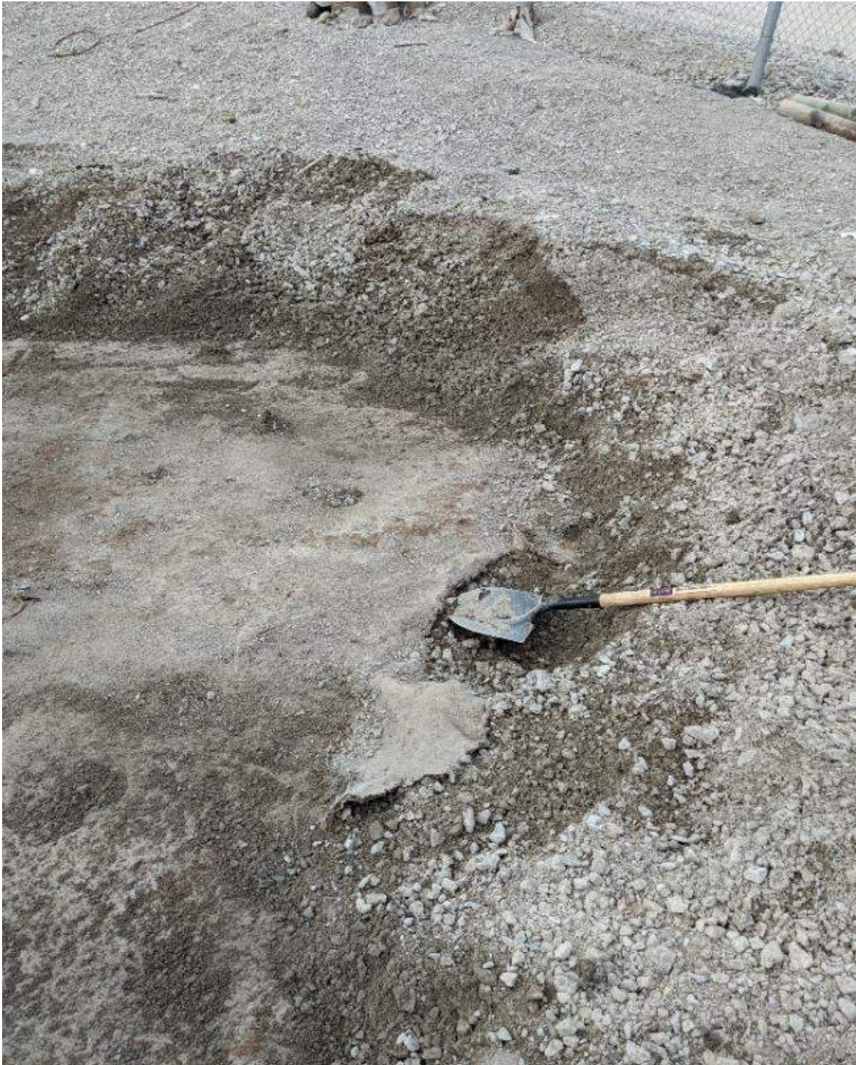
Photograph #1: Damaged existing liner at the top of the embankment, north discharge station.
