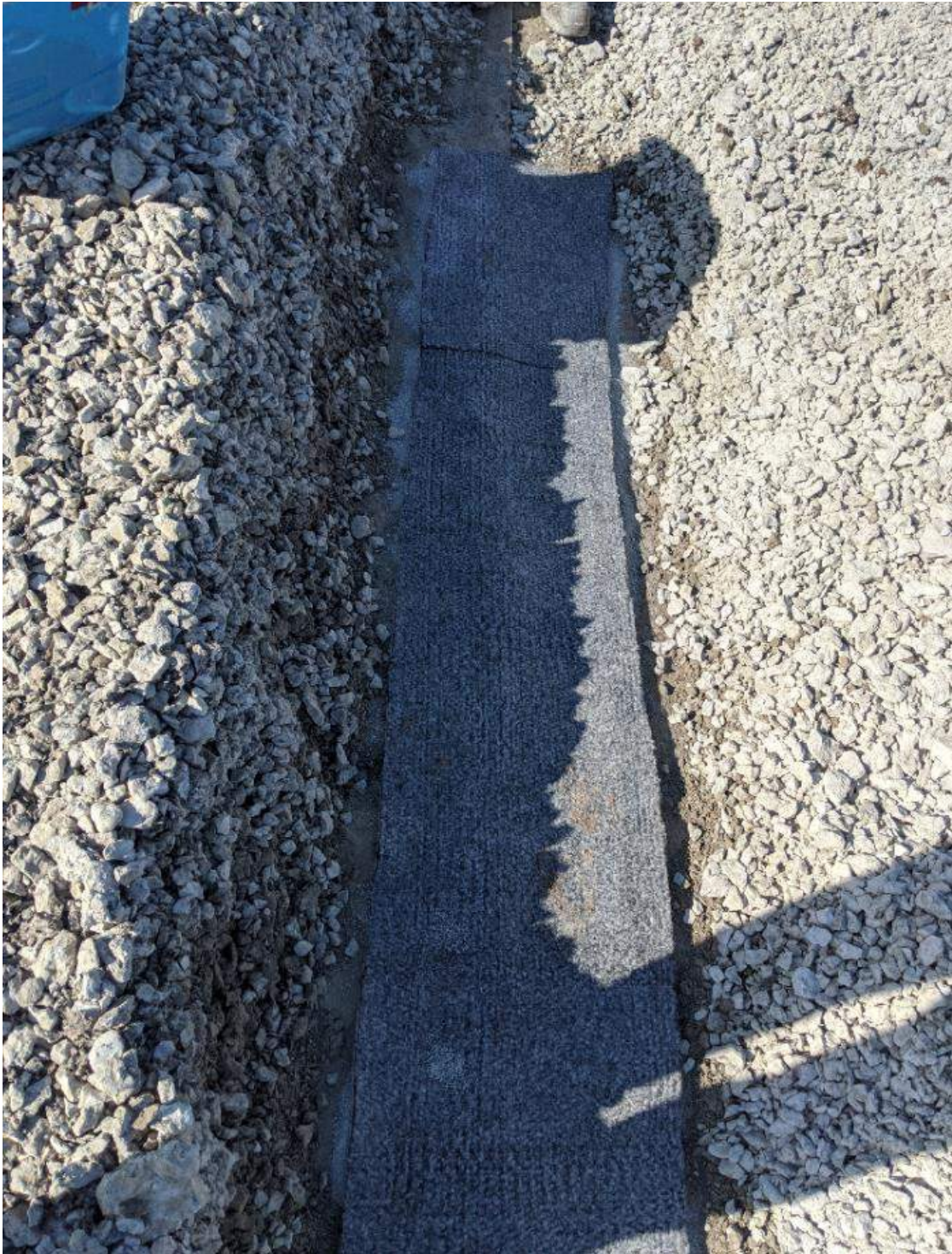
Photograph #1: Strip of liner placed over the existing seam, in a location where the existing overlap was too narrow.
