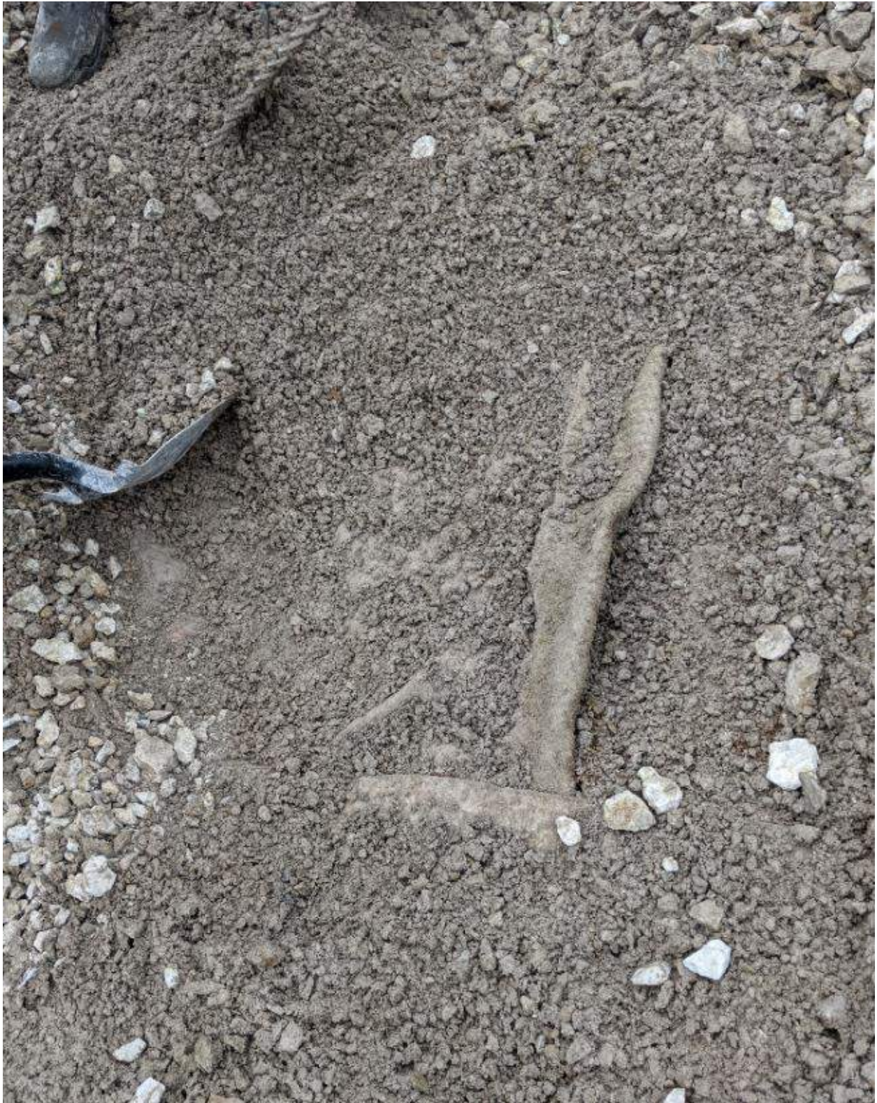
Photograph #5: Horizontal seam has rolled. Top of embankment is towards the right in this photo.
