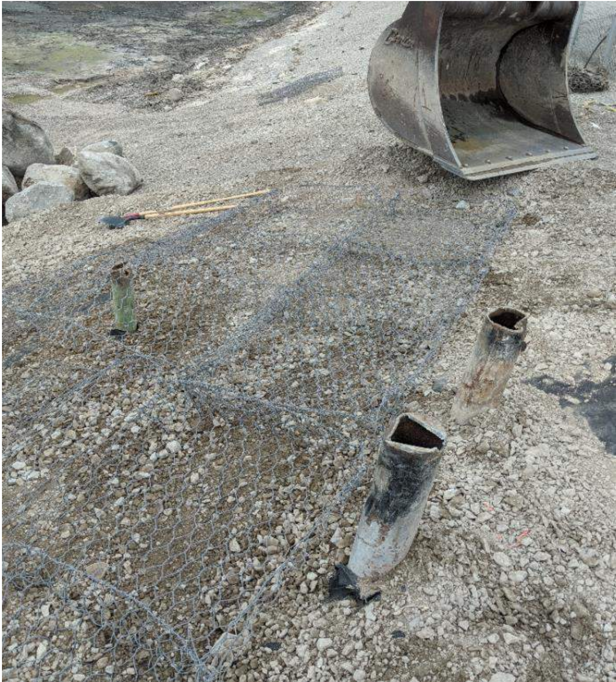
Photograph #2: Installation of gabion cages. The discharge station's lower piles pass through the second row of cages, anchoring the entire gabion mat in place.
