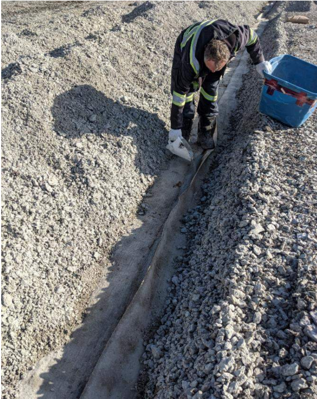
Photograph #2: Re-sealing the seams with bentonite. - END OF REPORT -
