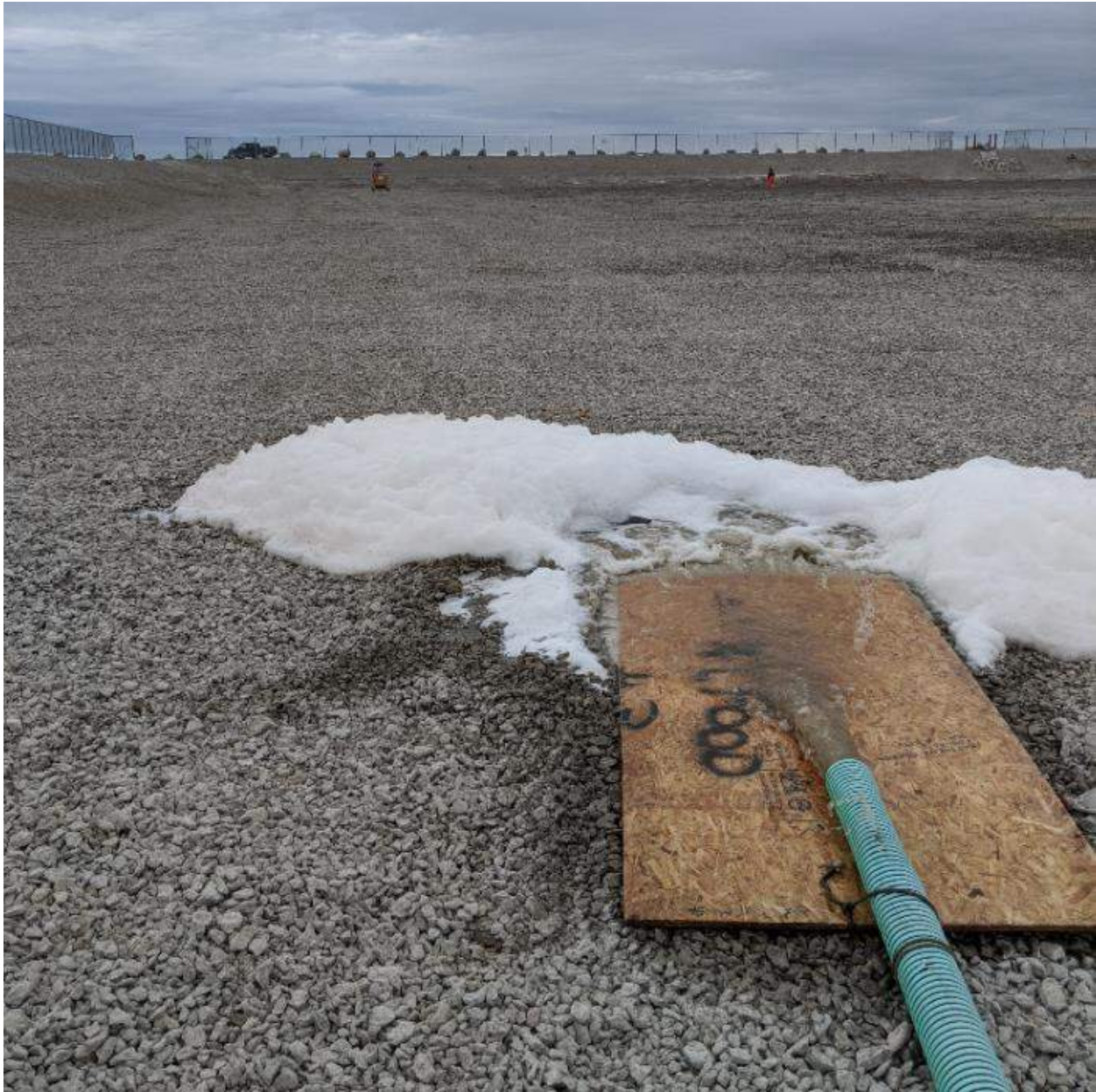
Photograph #2: Water being pumped form the North cell into the South cell.
