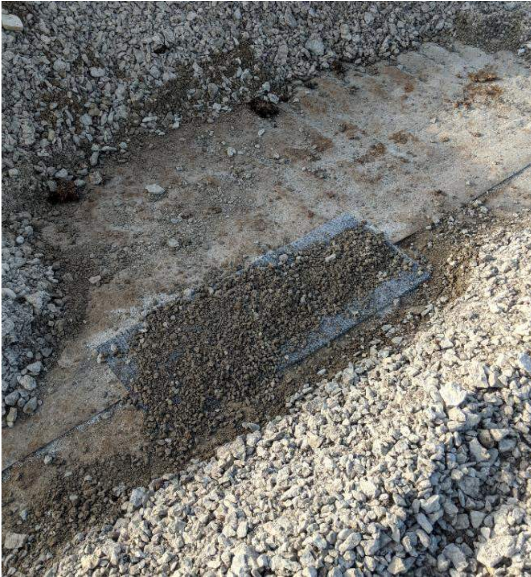
Photograph #1: Patch covering a local defect within one of the seams.
