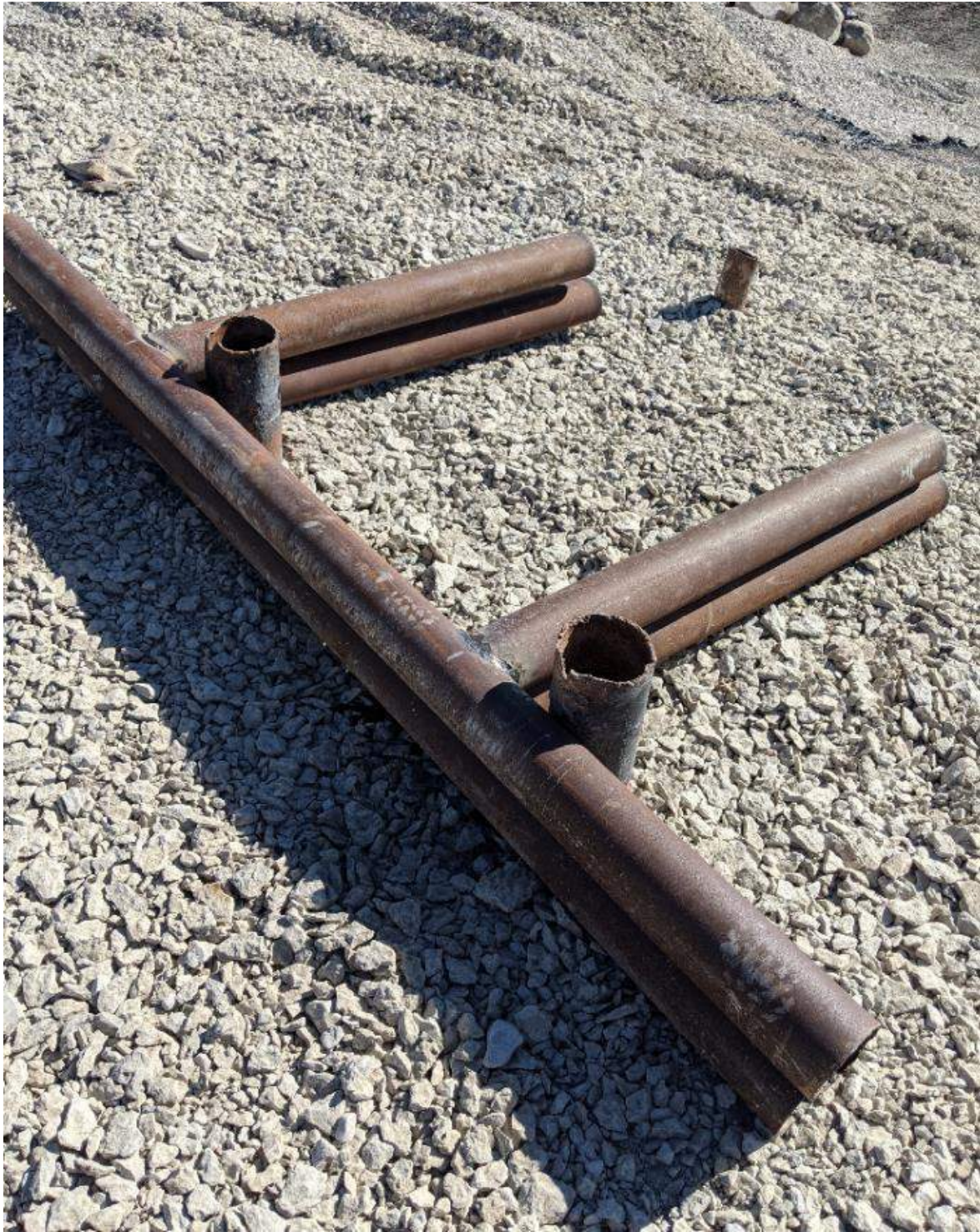
Photograph #1: Final design of the truck bumper (north station). The structure will eventually be moved so that the back end of the truck bumper, to the right in this picture, is against the front piles of the discharge station.
