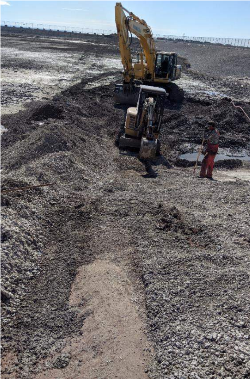
Photograph #3: Competent liner was found approximately five meters further than originally exposed. This is where the new liner will seal onto the existing liner once the latter is cleaned.
