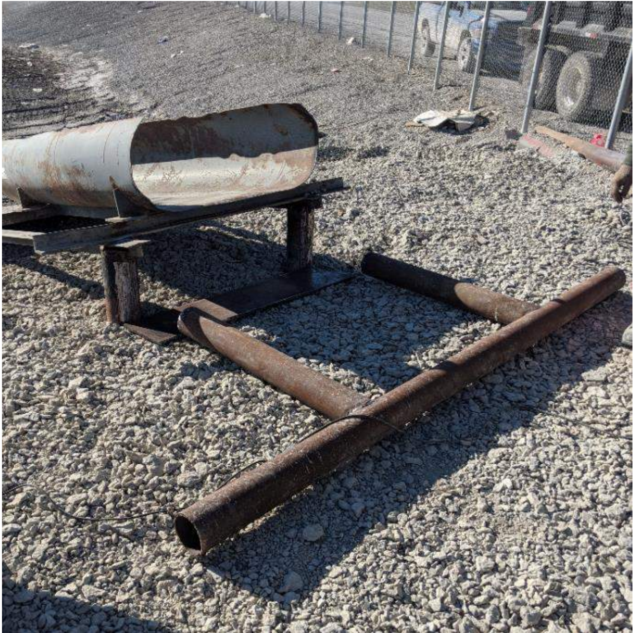
Photograph #1: Various pieces of the truck bumper prior to assembly onto the discharge station piles.
