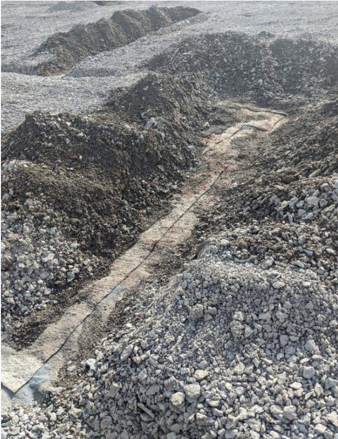
Photograph #1: North-south seam, exposed and re-sealed, awaiting backfilling. This particular seam features a key cut into the edge of the panel. No apparent feature was observed that would require this key, but it does not appear to compromise the liner integrity.
