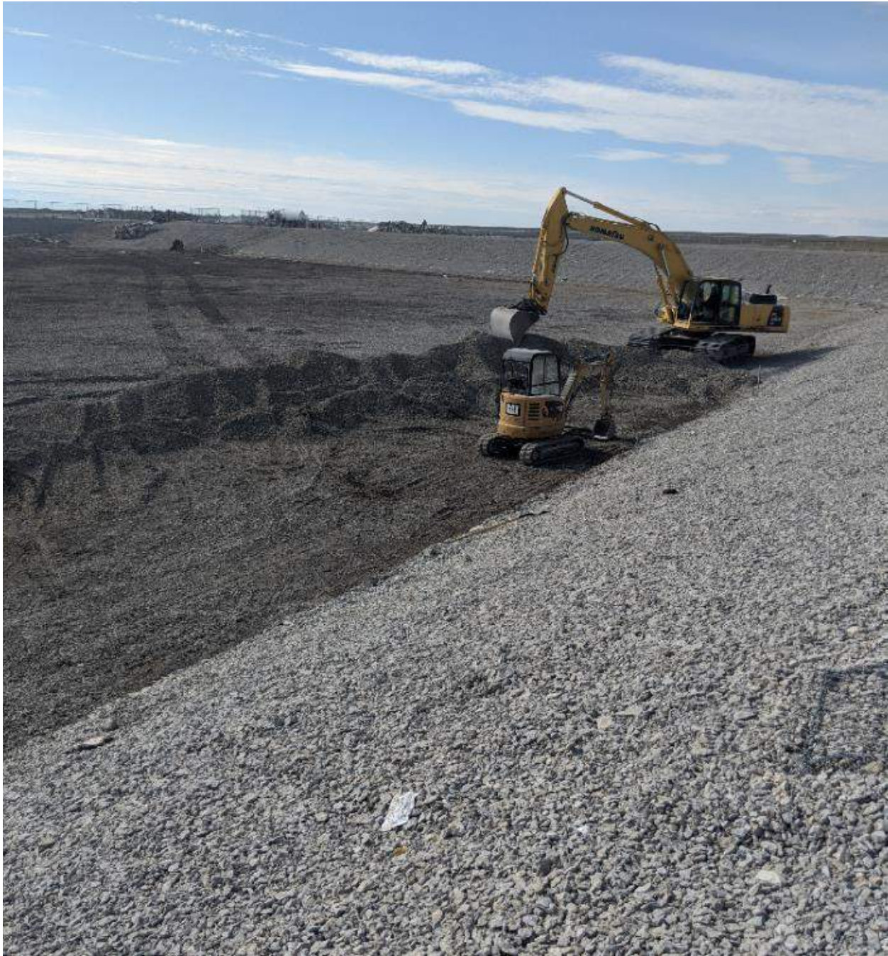
Photograph #2: Clearing aggregate from along the East berm of the south cell.
