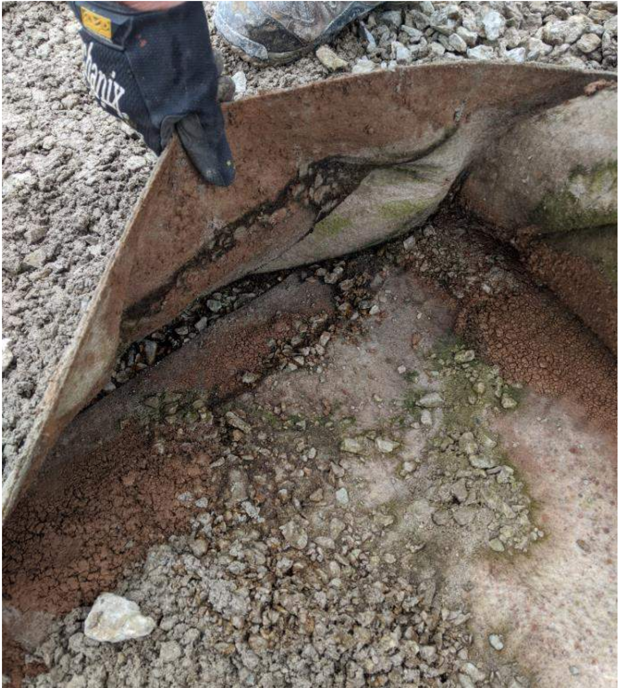
Photograph #6: Evidence of significant water flow under the liner, with algal growth suggesting this area was quite wet and nutrient-rich.
