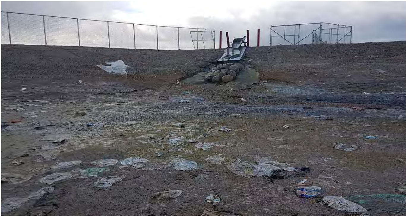
Photo 5: North discharge area. GCL exposed around the larger stone. Gabion baskets highly eroded.
