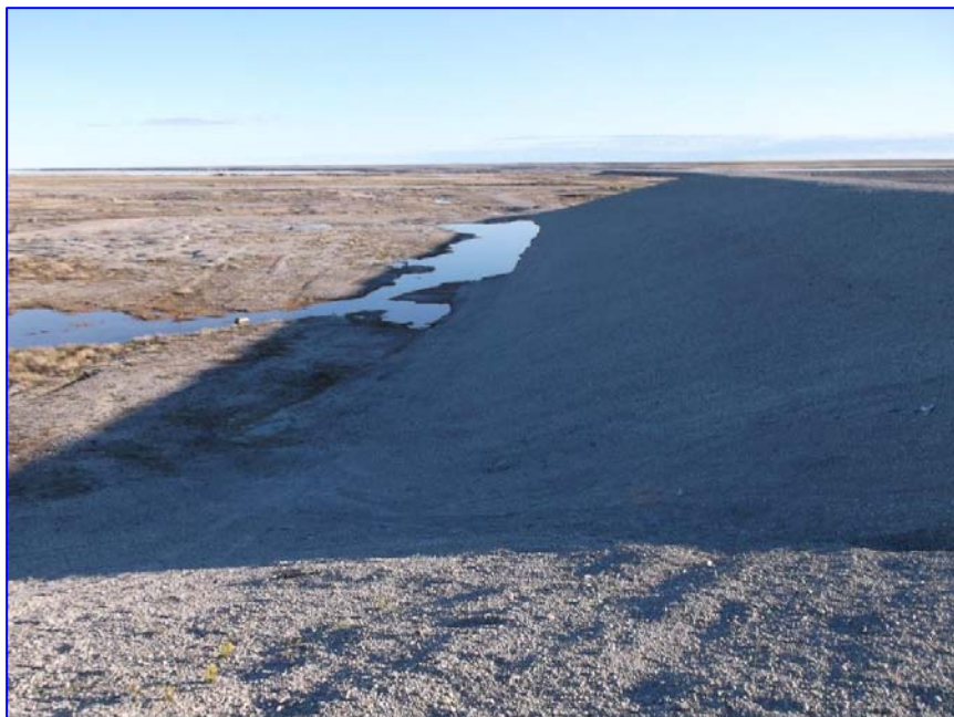
Photograph No. 15 Ponded water close to the toe of the east berm of the water reservoir
