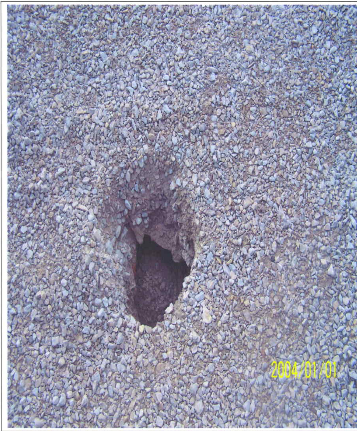
Hole developed outside of the E-W containment berm of Lagoon cell 1, Which drained out cell 1. Photo taken, July 25, 2008.
