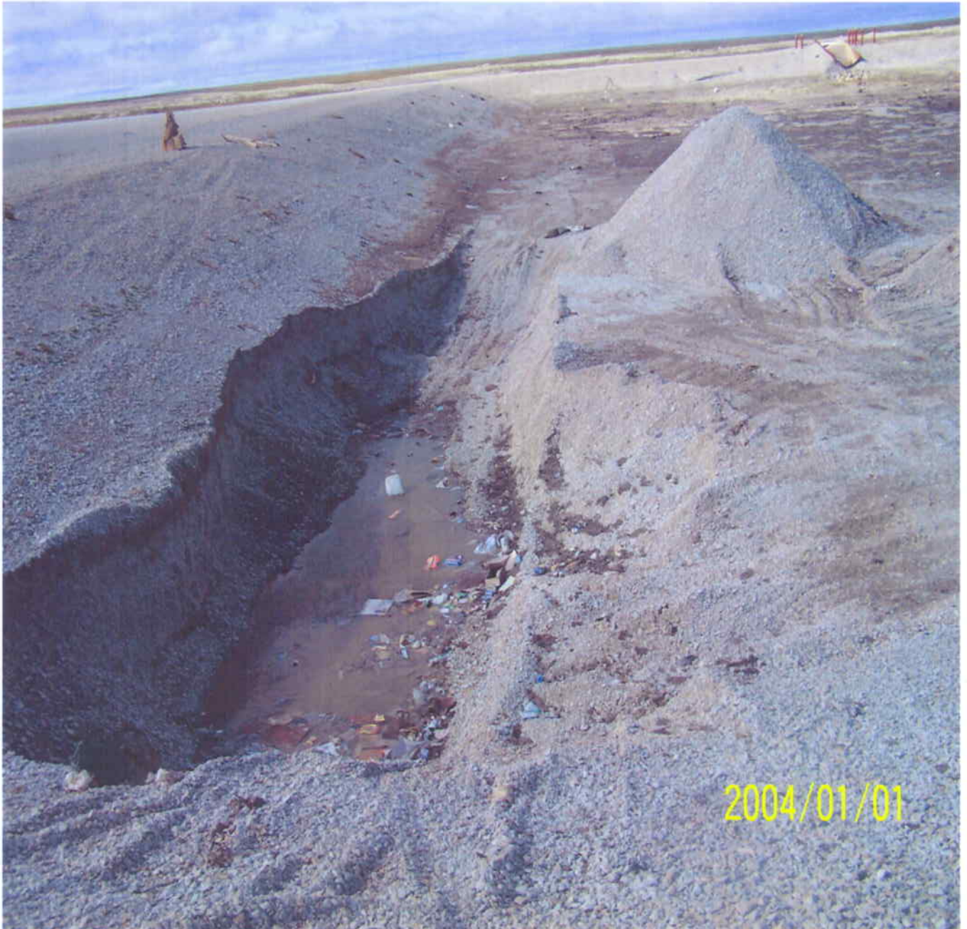
Excavated along the E-W berm where leakage occurred of Lagoon cell 1 Photo taken in July 25, 2008
