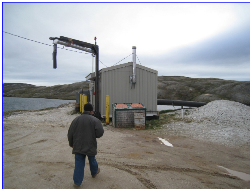
Photograph No. 10 Intake pipe and truck fill station
