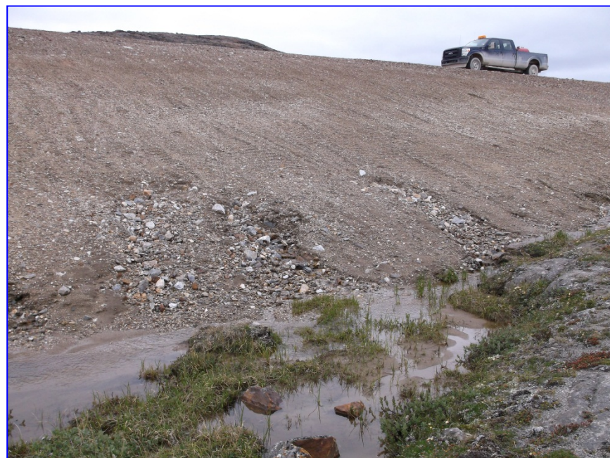
Photograph No. 6 Leakage of lower sewage lagoon berm
