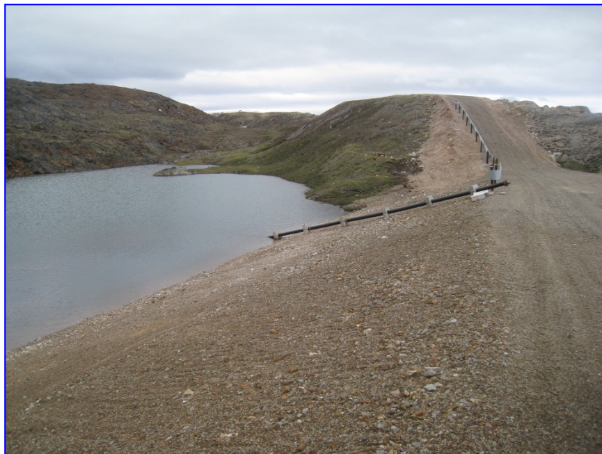
Photograph No. 4 Inlet pipe of lower sewage lagoon
