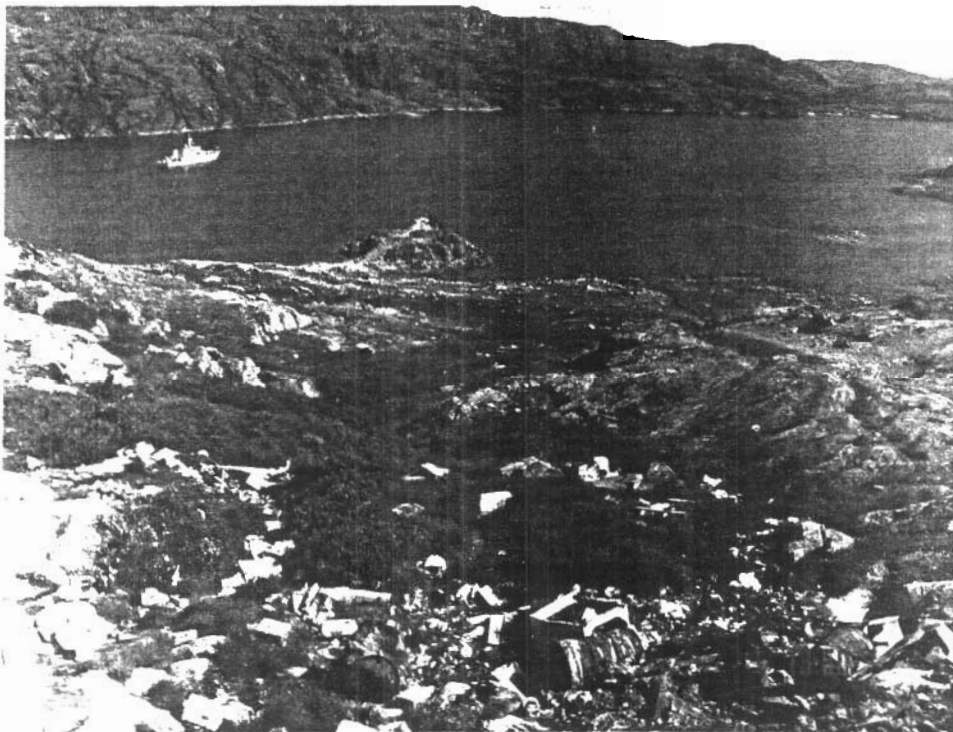
Photo # 8 Flow path of sewage effluent flows through solid waste disposal facility. Note at front of photo refuse that sewage stream has carried from the tipping face.
