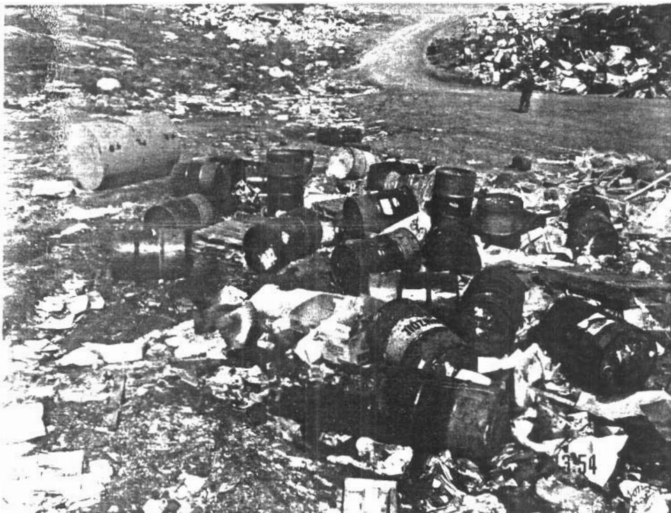
Photo # 6 Waste oil and drum storage area at Solid Waste Disposal Facility. Note that there is oil staining in the area.
