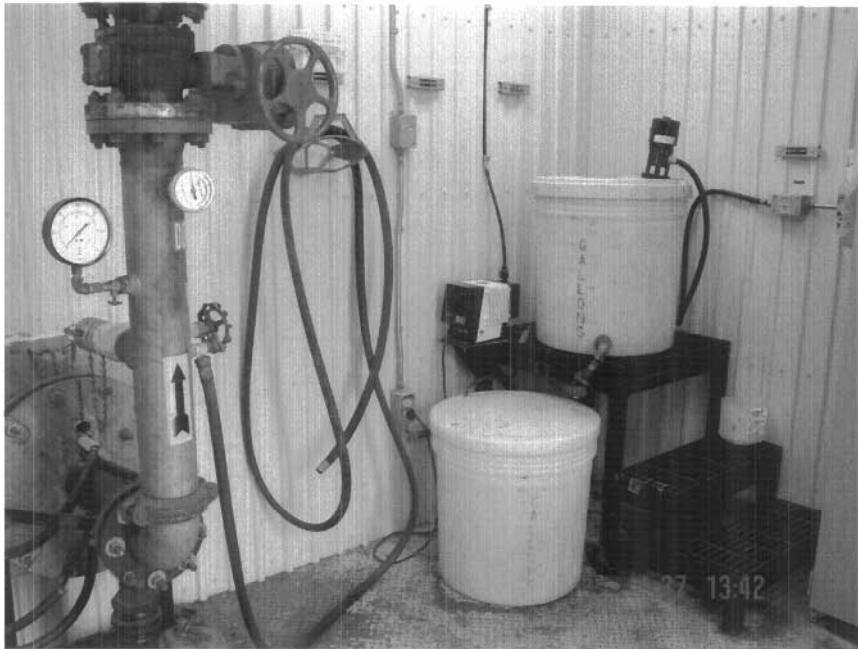
Photo 3. Chlorination system at Water Intake Facility.
