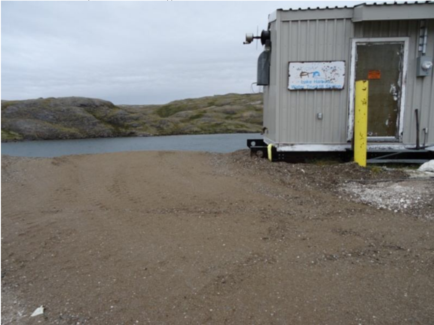
Figure 2 Intake station - Note removal of fuel tanks and re-grading of ground adjacent to building
