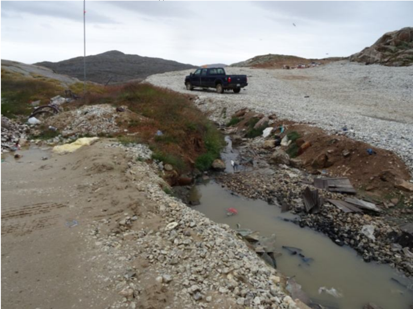
Figure 10 Ditch where raw effluent is deposited. Cover materials over the burn and bury in the back ground
