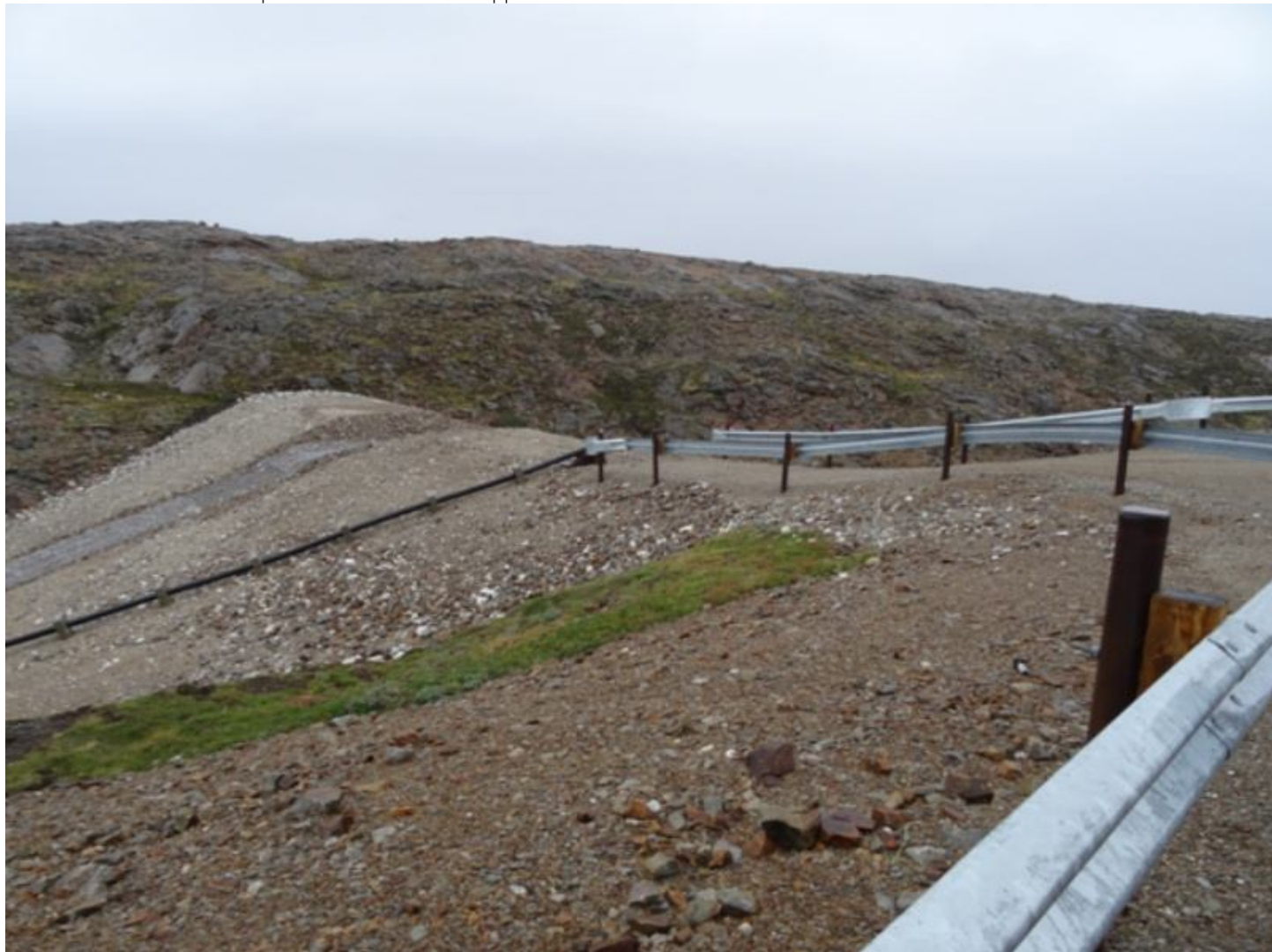
Figure 14 new lagoon with recontoured cell wall ( upper cell)
