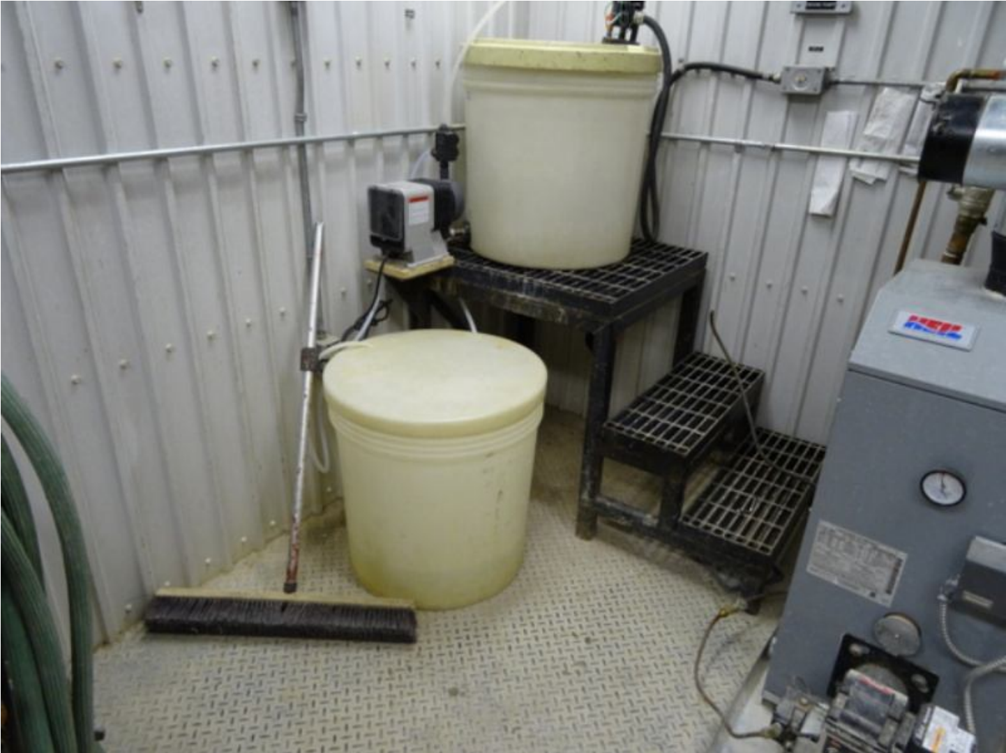
Figure 7 Chlorine system required regular monitoring to ensure it is not drawn down
