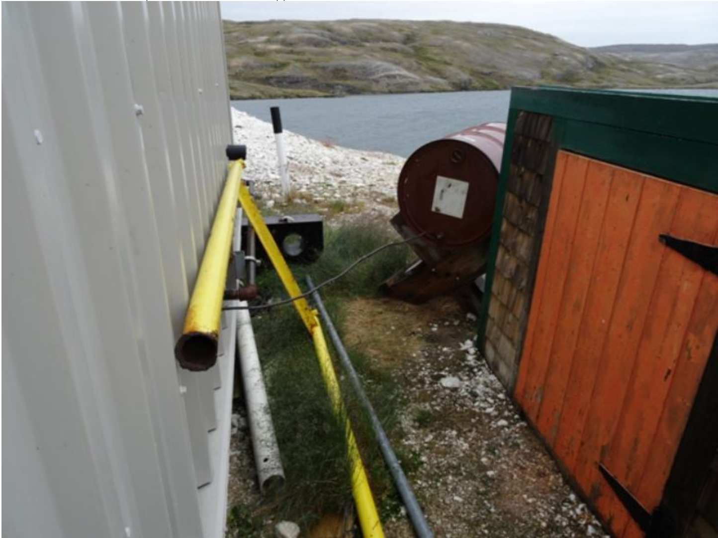
Figure 4 Drum feeding fuel oil into building
