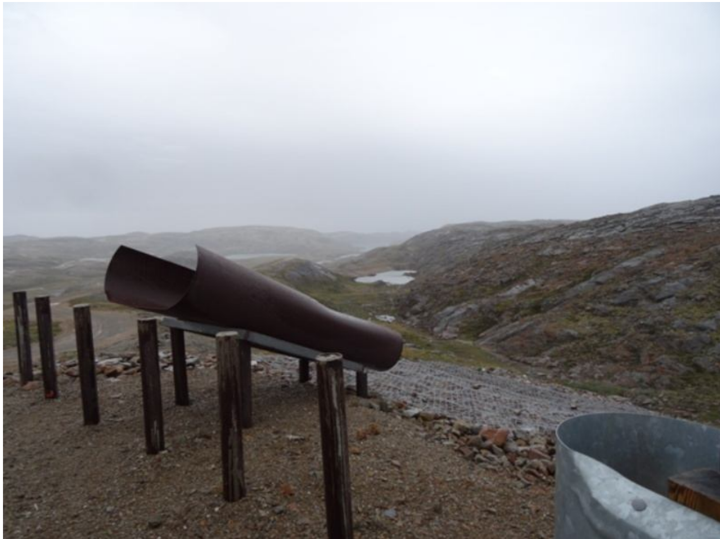
Figure 15 Upper cell of new lagoon - truck drop off. Below in background is lower cell berm wall with ponded water
