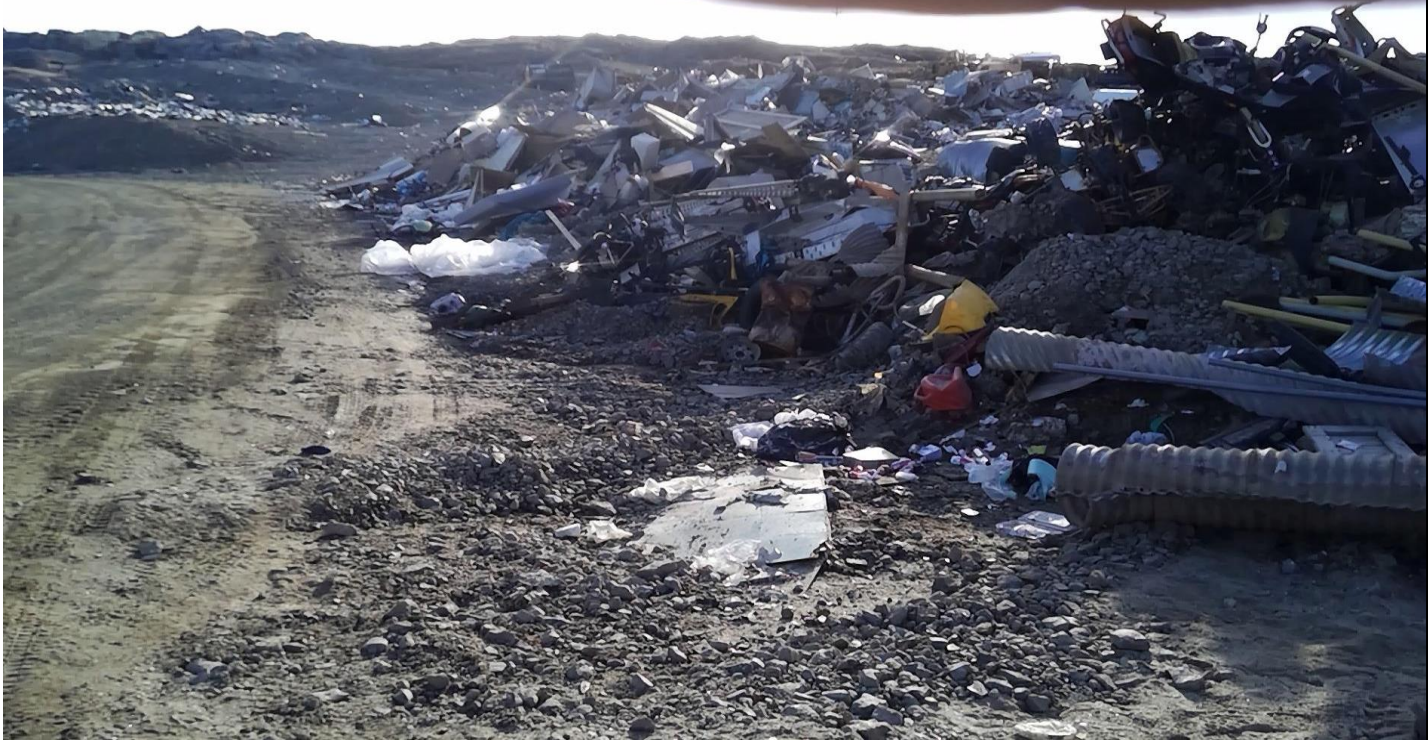
Description: With the exception of domestic burning and capping waste, all other waste such as bulk wood, bulk metal, hazardous waste, and gravel have been deposited into the pile along the road. The trench the direct any leachate from the pile was covered as directed in 2020.
