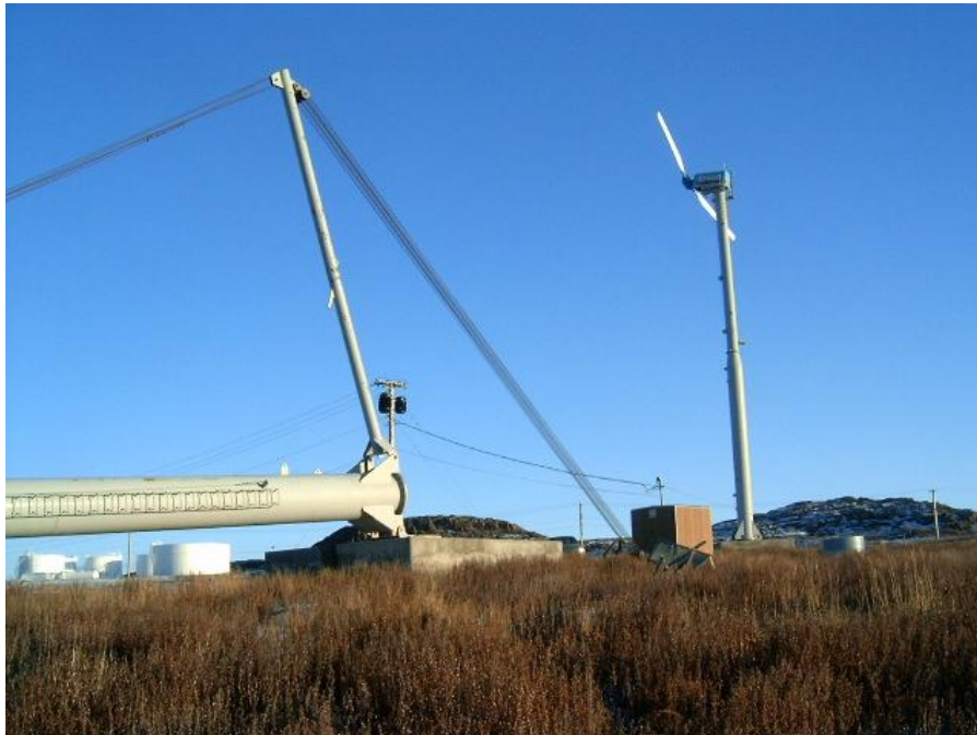
Photo 28 Wind generators west of Hamlet.
