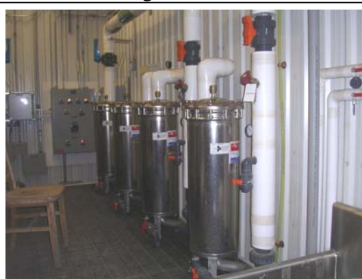
Cartridge Filters in WTP
