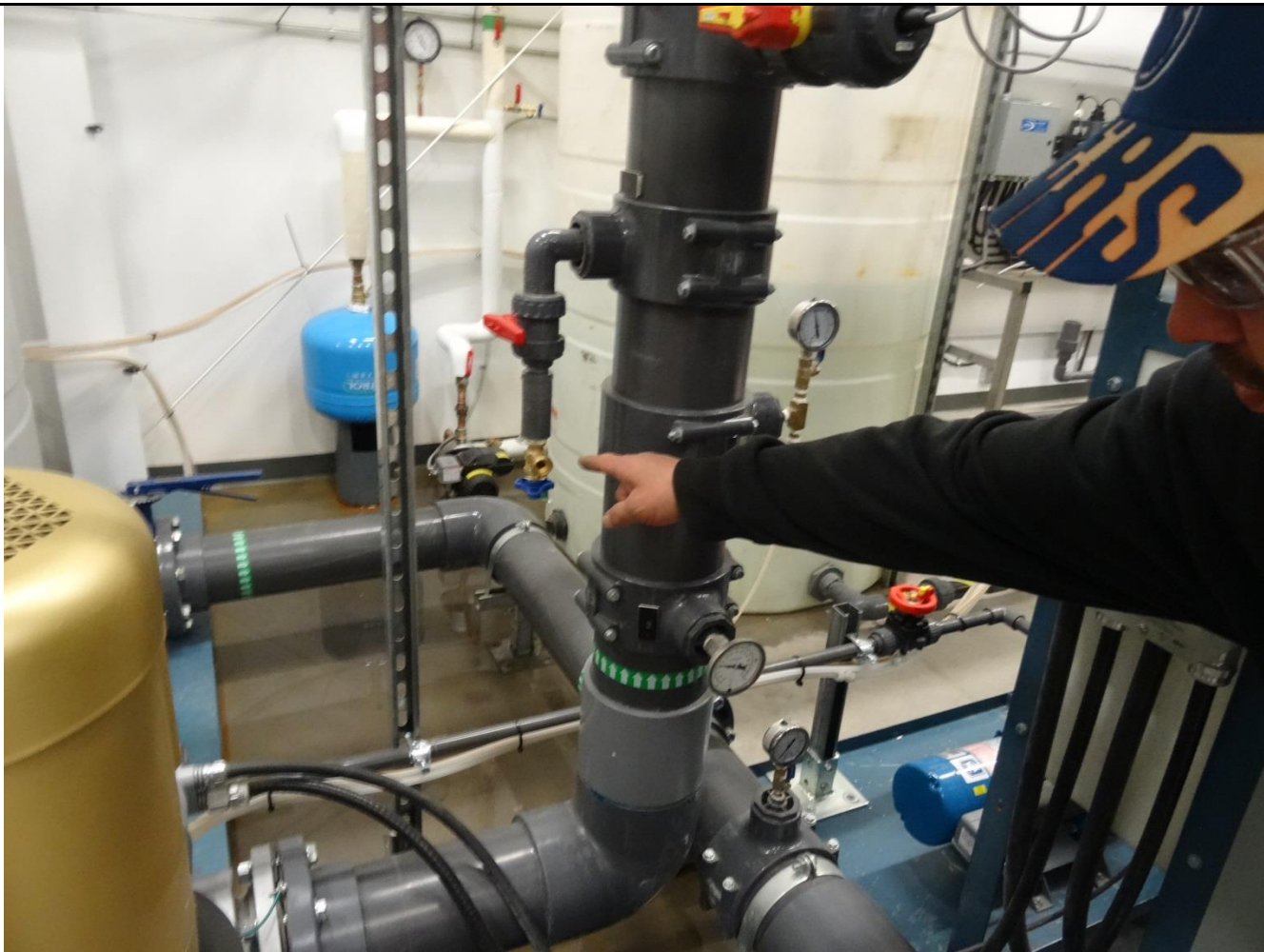
Description: No Signage for Sample Station KUG-1C – Raw Water Test Point in New Water Treatment Plant
