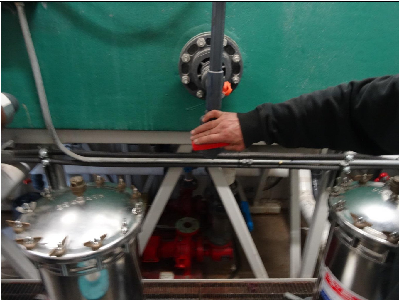
Description: No Signage for Sample Station KUG-1B – Raw Water Spout in Old Water Treatment Plant
