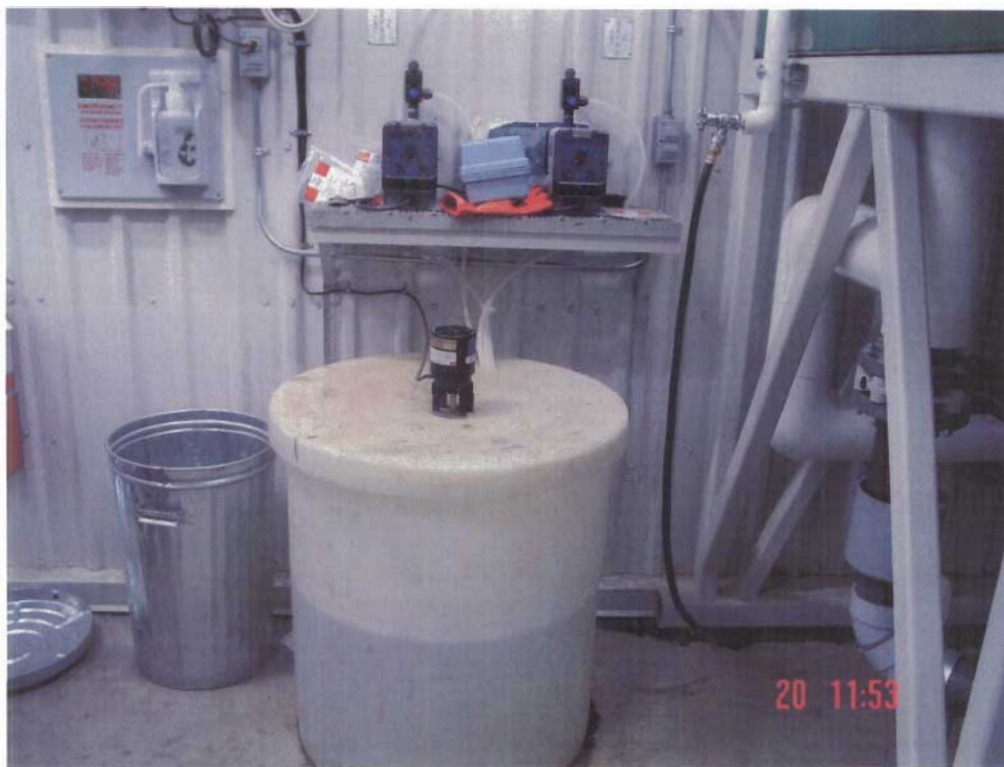
Photo # 4 Chlorination system in use at Water Treatment Plant. No formula found for concentrated chlorine mixture; Log book up to date.
