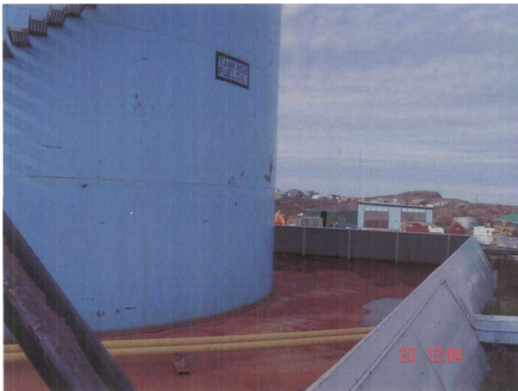
Photo # 8 Tank farm shown with metal berms no leakage noted; tank farm within 50 metres of water reservoir.
