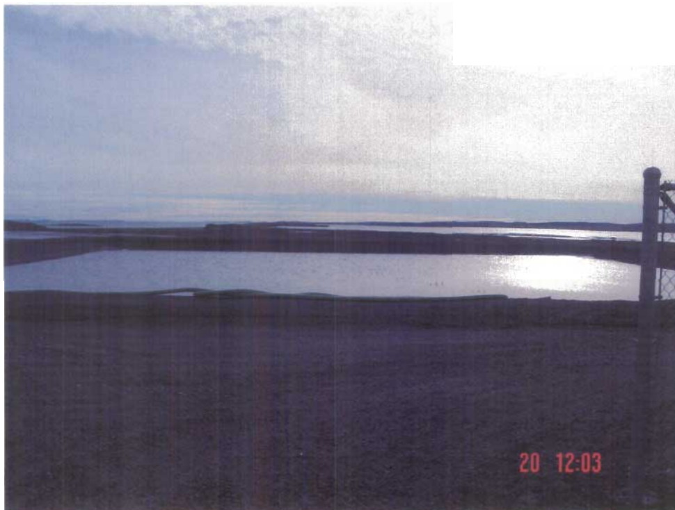
Photo # 2 Water reservoir at Kugluktuk located by Water Treatment Plant. Reservoir holds about 10 days supply for community.
