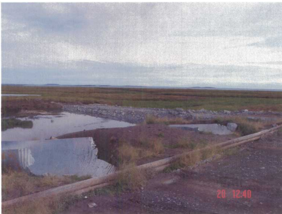
Photo # 10 Sewage truck discharge structure at sewage treatment facility; seepage berm shown to the right.
