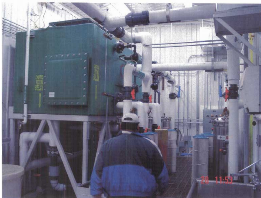
Photo # 3 Filtration system shown in Water Treatment Plant. Filters unable to remove silt from drinking water.
