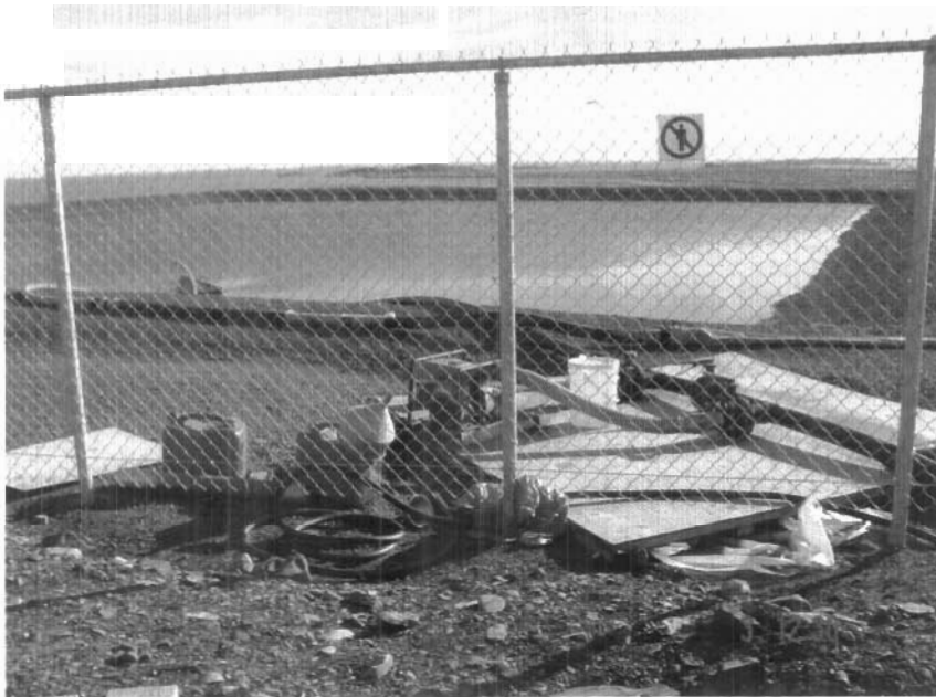
Photo 10. Water reservoir gas powered water supply pump within berm.
