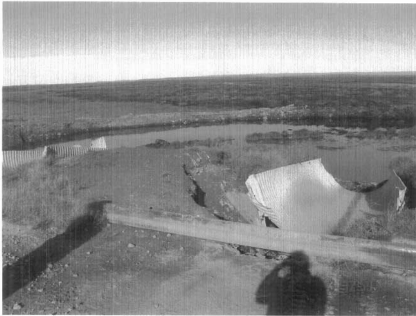
Photo 17. Sewage truck discharge structure at Sewage lagoon.
