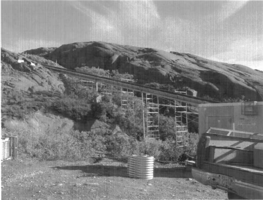
Photo 1. New water conveyance line under construction.
