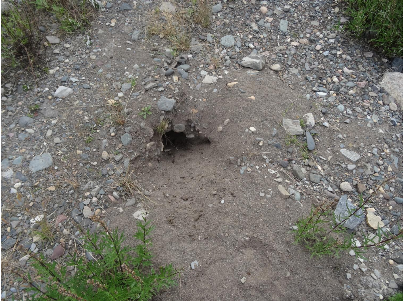
Description: 1 of a number of Animal Burrow Holes found in the Sewage Lagoon Berm
