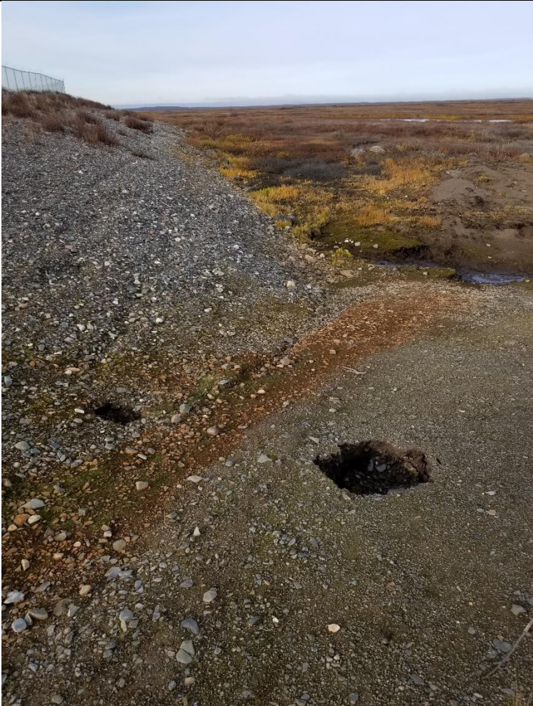
Description: Holes appearing in Buttress due to Leakage Flow underneath from Sewage Lagoon, View 2 as seen on 2020 September 25
