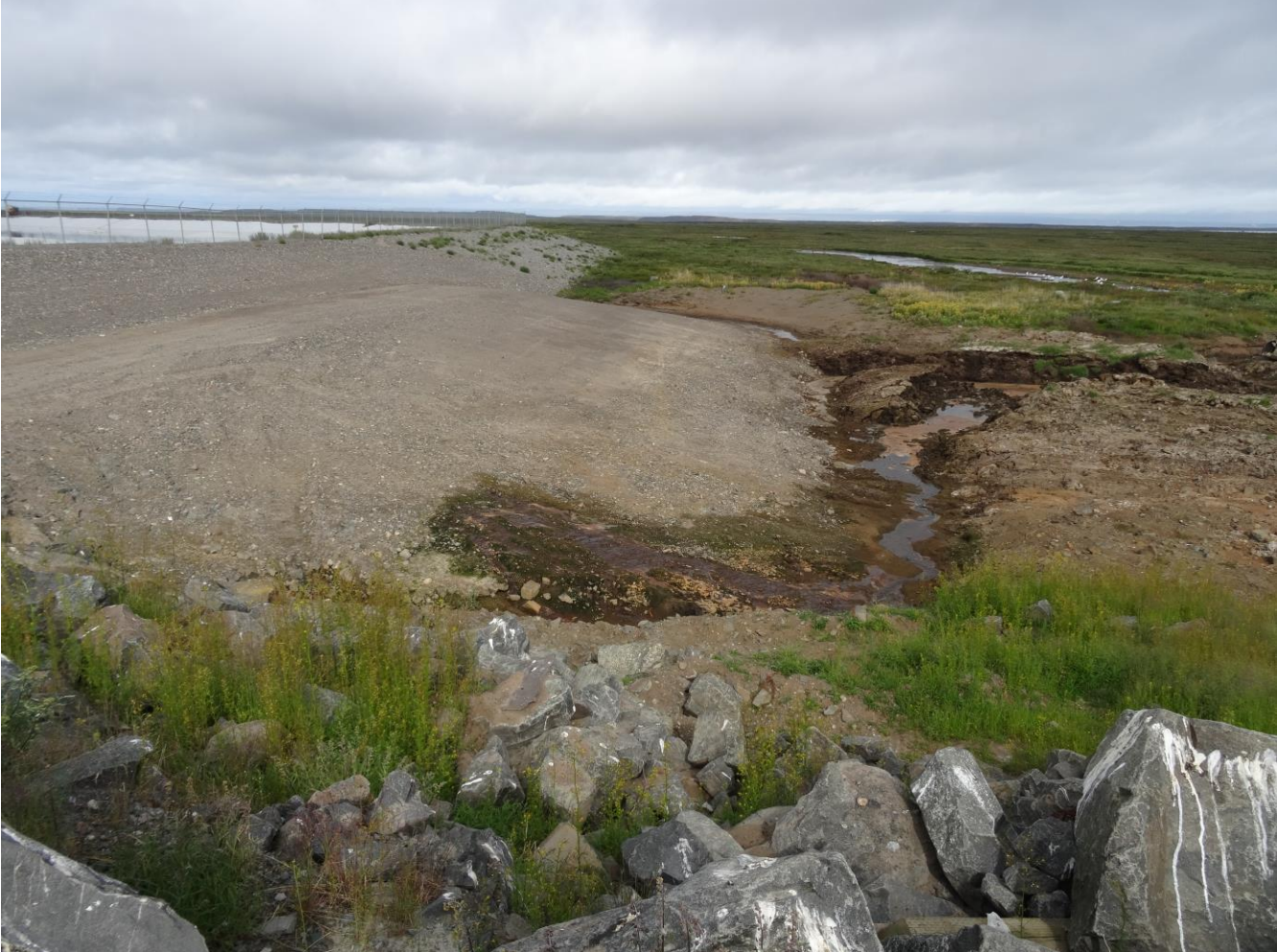
Description: Leakage through the Sewage Lagoon Buttress on the North side of the Berm
