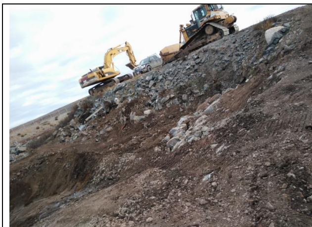
Pic 1: Lagoon Berm protection buttress
