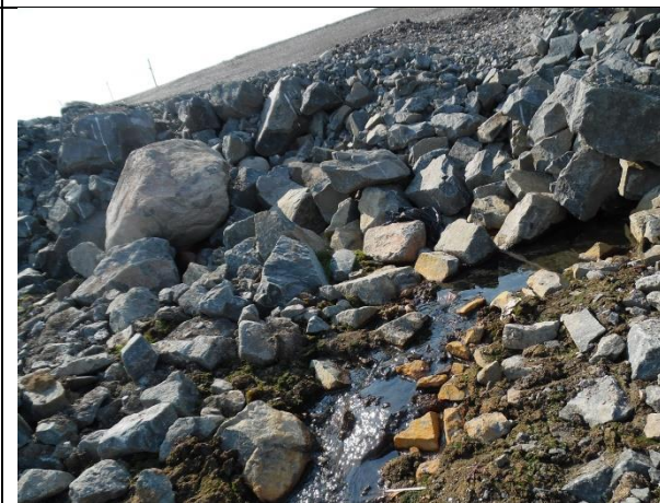
Pic 12: Sewage lagoon leak continued
