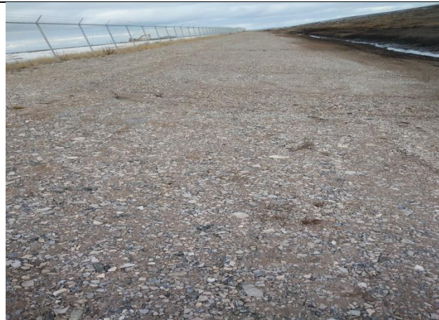
Pic 6: Lagoon side berms slumping repair
