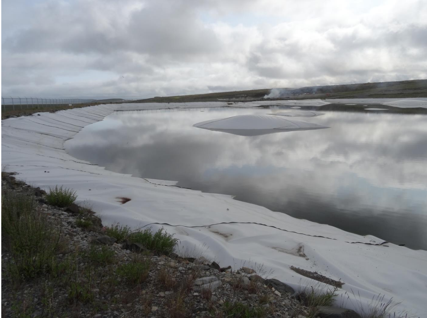
Description: Extremely Low Levels within the Lagoon BEFORE Decant Program showing large volume of continuous Leakage
