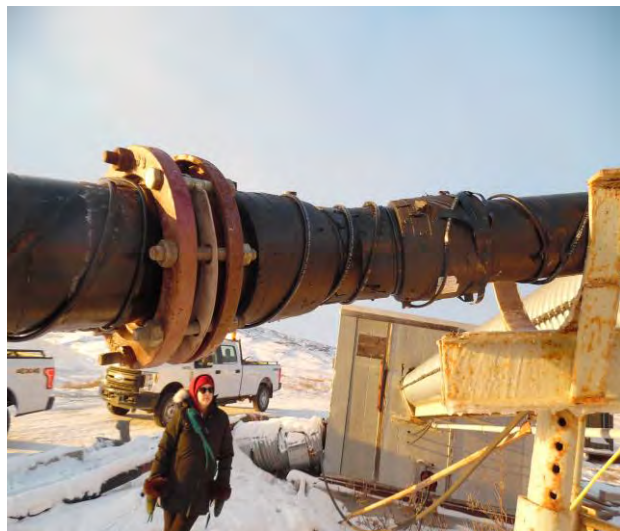
Insulation reinstates at the heat trace burnt section of the old IPH
