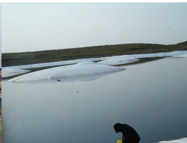
air bubbles in lagoon liner
