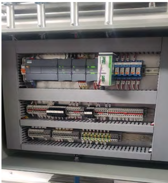
New PLC remote I/O at new WTP
