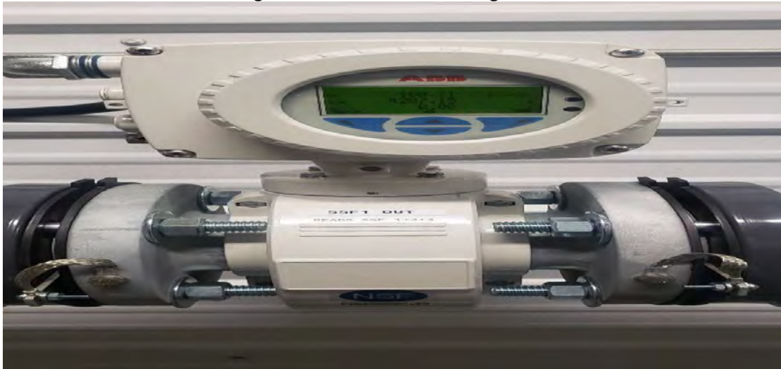
New ABB flow meter for Slow sand filter
