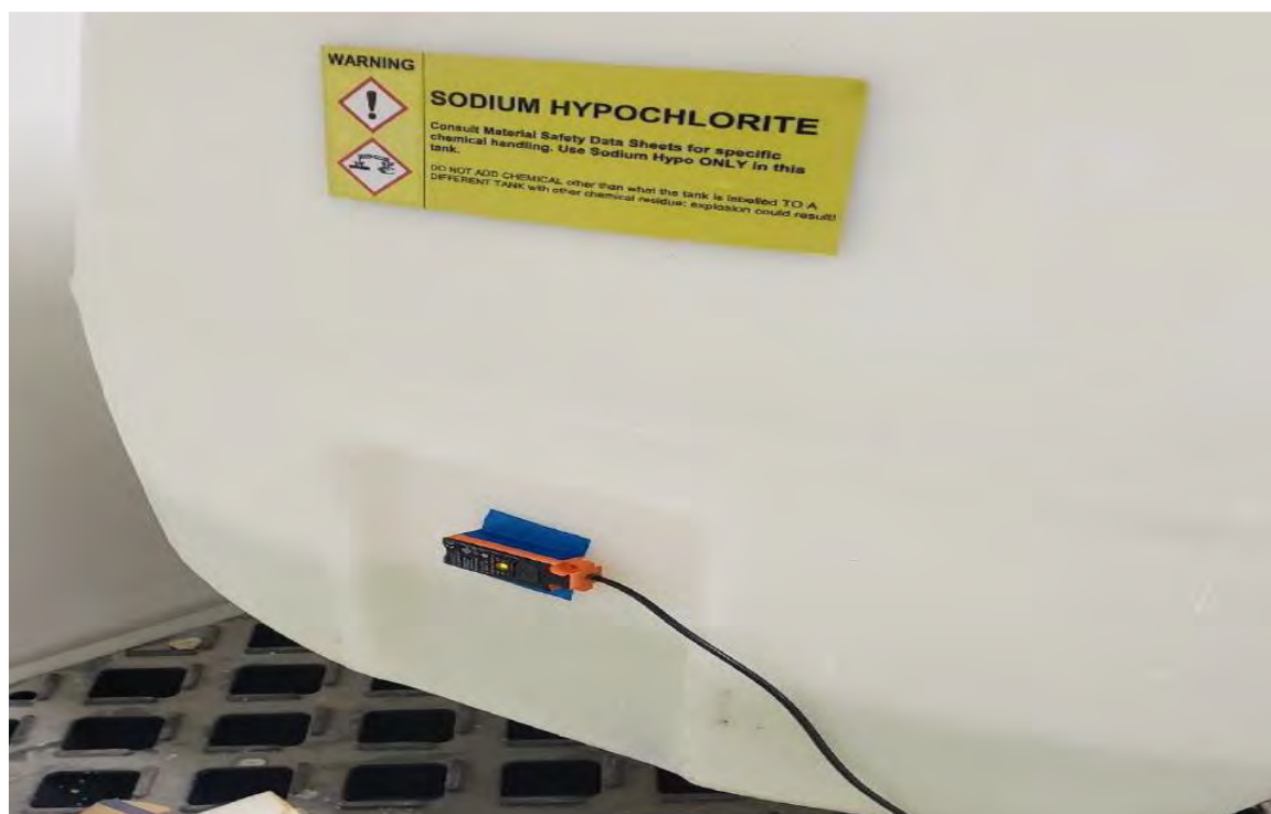
Sensor for Cl 2 level in the mixing tank
