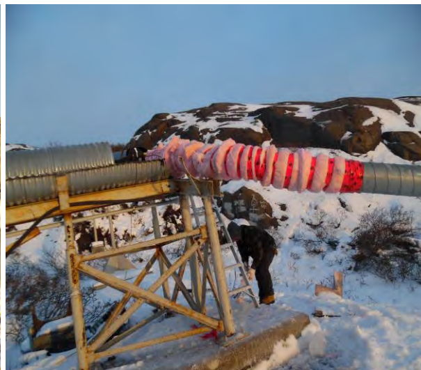
Insulation reinstates at the heat trace burnt section of the old IPH
