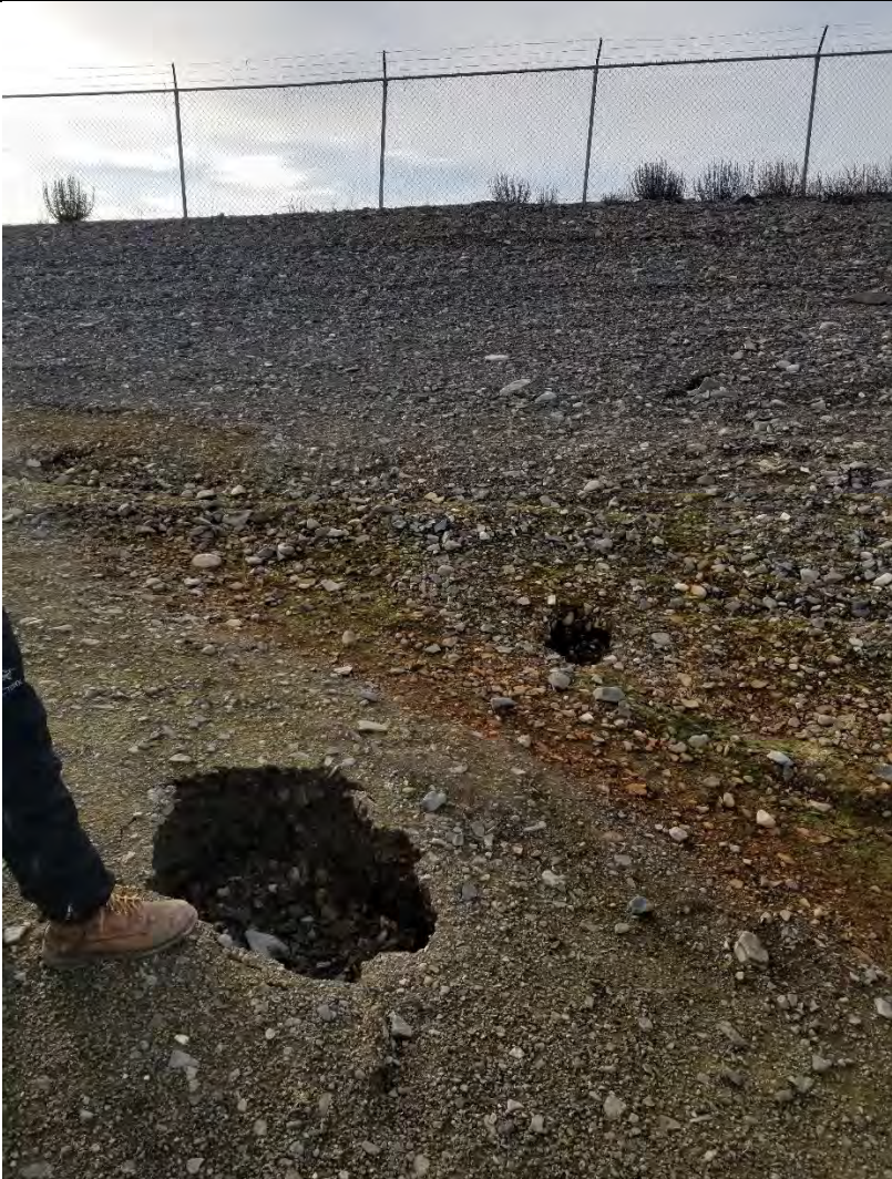
Description: Holes appearing in Buttress due to Leakage Flow underneath from Sewage Lagoon, View 1 as seen on 2020 September 25
