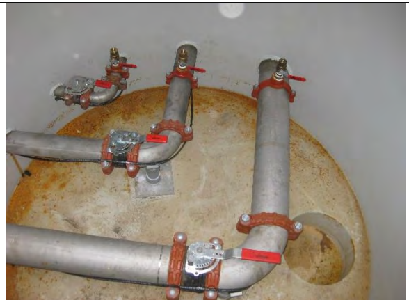
Photo 16: Vault 5 contains elbows and shut-off valves. Note heat trace.
