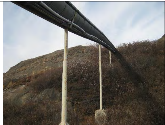
Photo 4: Frost action has caused supports to become uneven.
