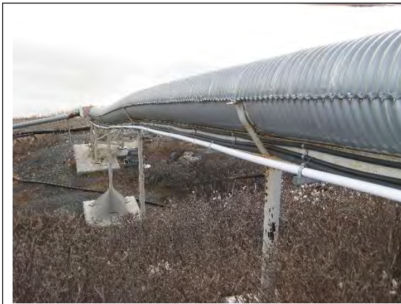
Photo 3: Elevated pipeline is supported on columns and concrete pads.
