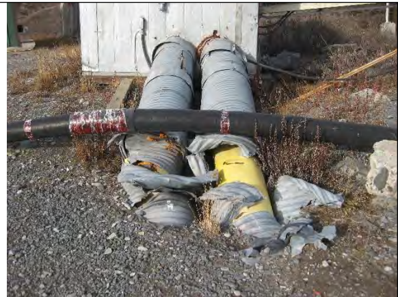
Photo 6: Steel casing and jackets damaged at the road crossing.
