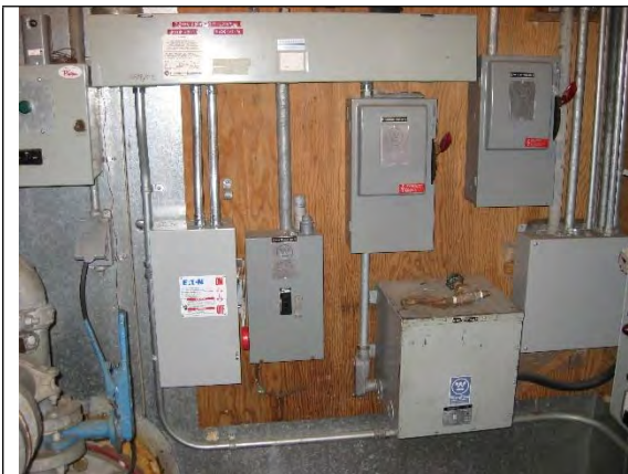
Photo 13: 600V equipment for raw water pumps.
