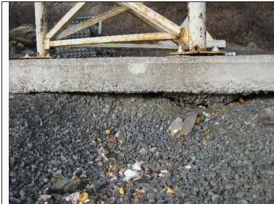
Photo 5: Concrete pads are losing granular support.
