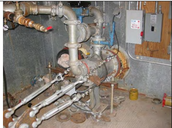
Photo 12: Mechanical equipment in the Old Pumphouse is in fair condition. One of the pumps has been removed.
