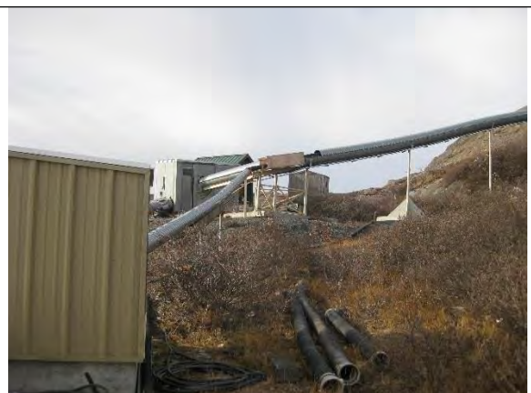
Photo 2: Tee removed, original pipeline now terminates only at the Old Access Vault 1.
