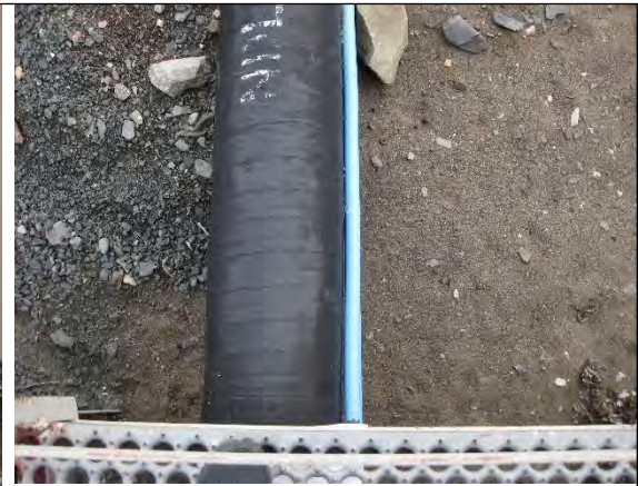
Photo 8: Pipeline downhill of the New Pumphouse. Compressed air line with light blue jacket.
