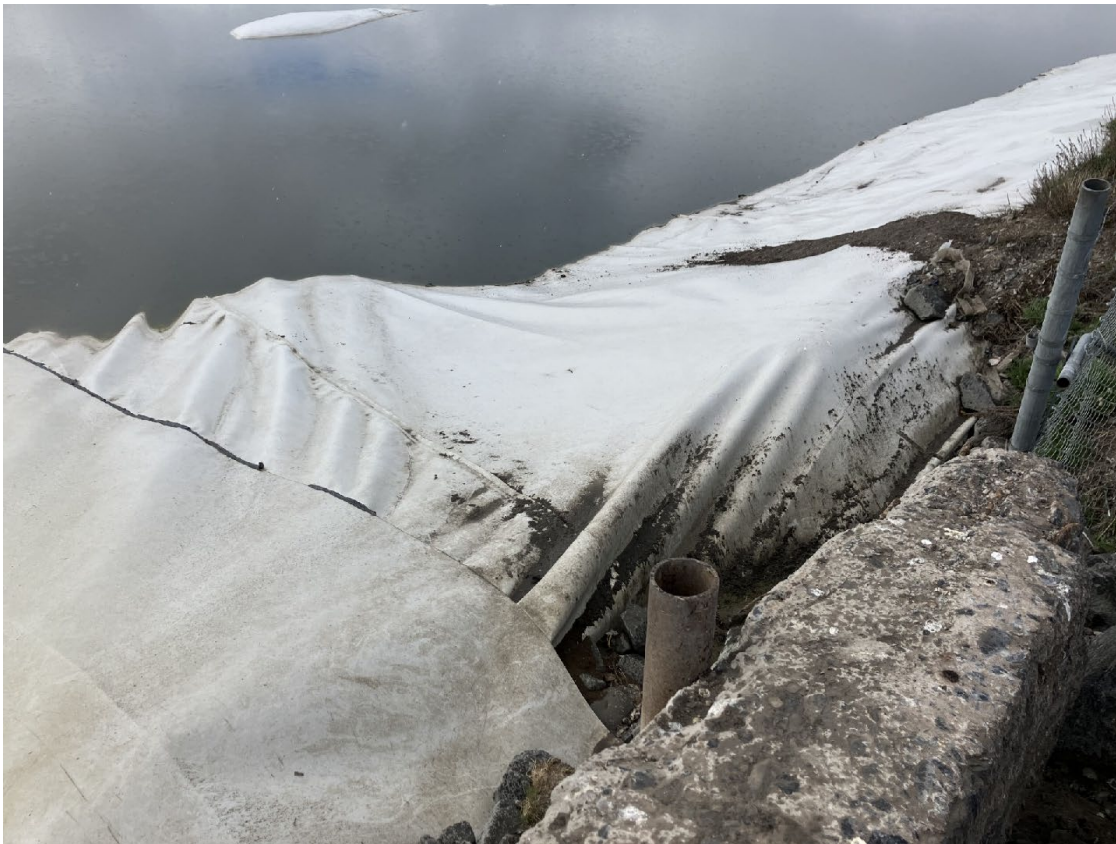
Figure 2: View of the truck fill erosion from above July 17, 2024.
