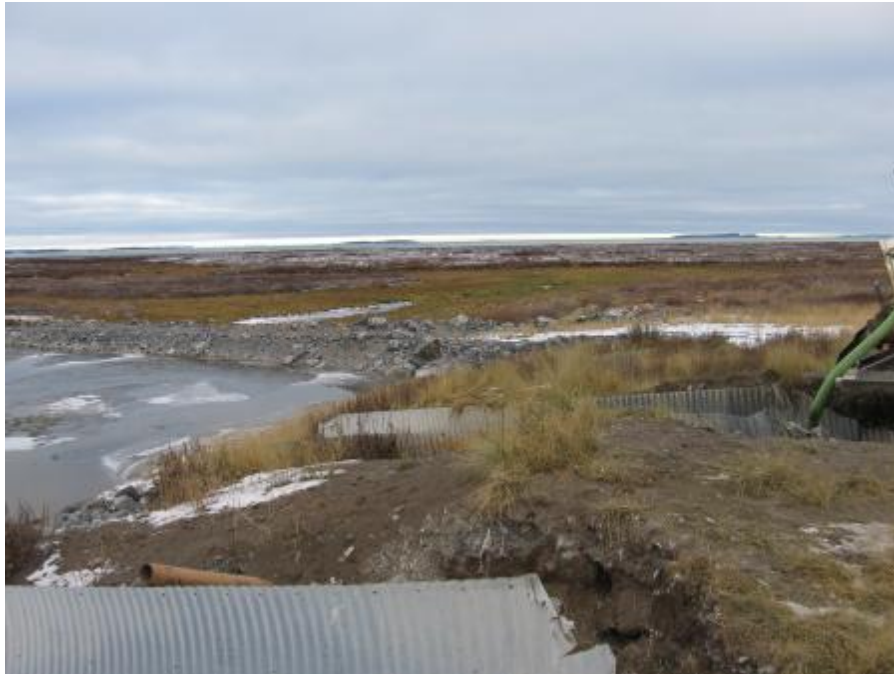
Photo 3 Culverts used as a spillway for truck discharge into the Sewage Lagoon.
