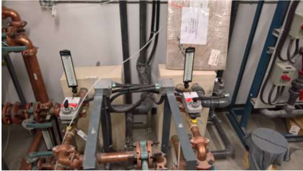
Fig. 9: Heat exchangers
