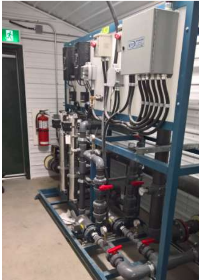
Fig. 8: Pump Skid 405, UV lamps and recirc pumps
