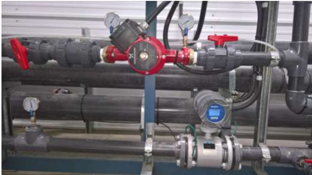
Fig. 10: One of the recirculating pumps and flowmeter FT-03 showing the recycle flow.
