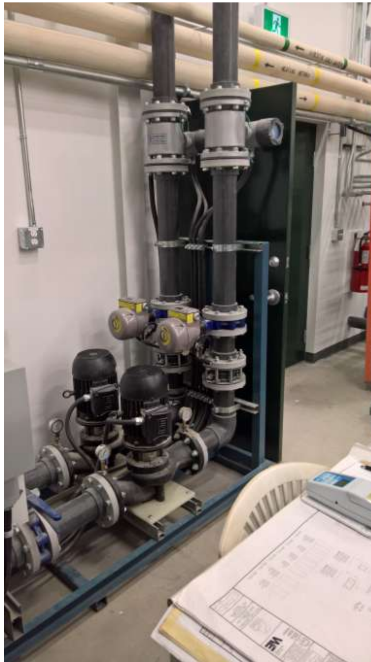
Fig. 14: Skid 406 showing Truck-fill pumps P14A and P14B
