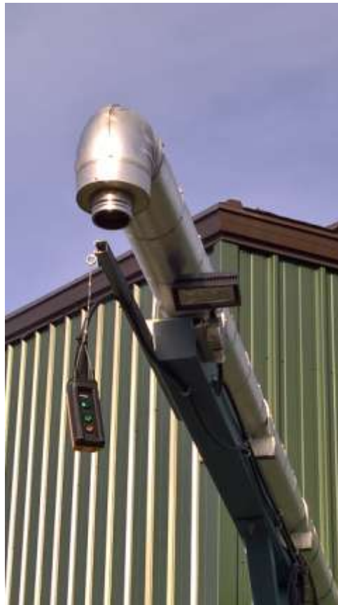
Fig. 13: Truck-fill arm prior to attachment of hose and sleeve.
