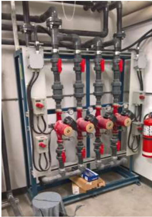
Fig. 11: Pump Skid 408 showing the Heat exchange pumps P-07A/B and P-08A/B.
