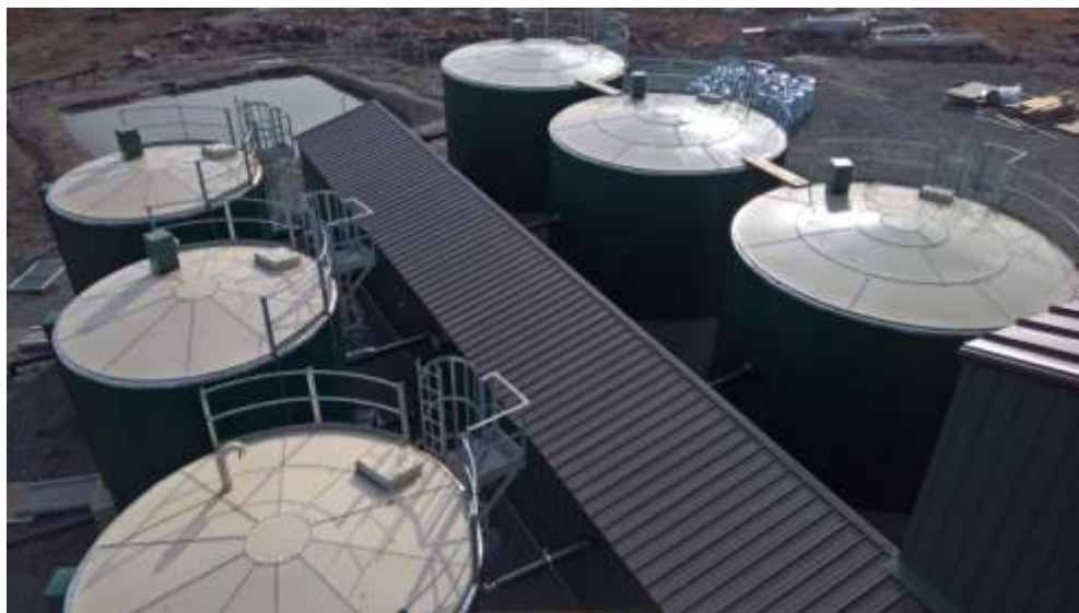
Fig. 17: Various slow sand filters and water storage tanks
