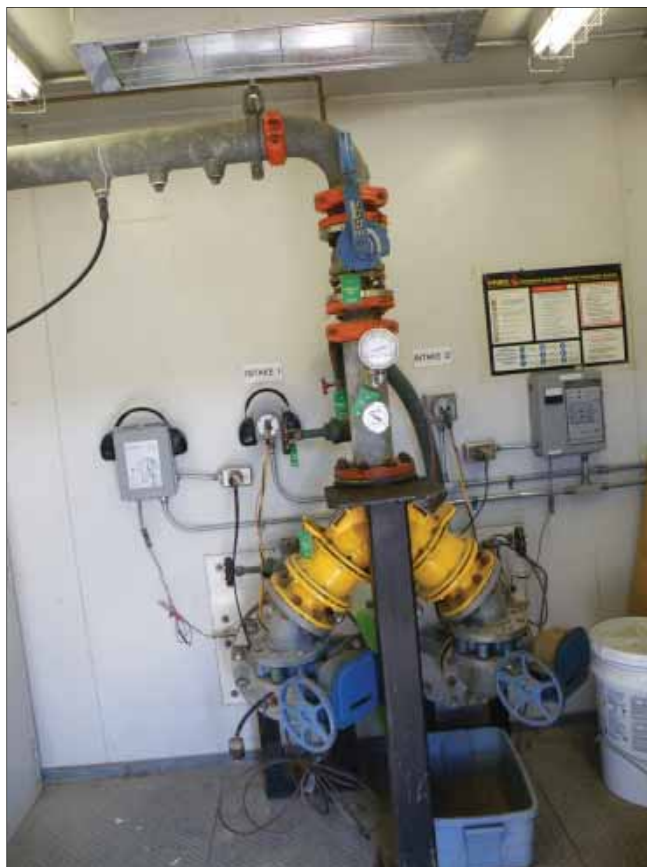
Photo 5: General Arrangement Intake
