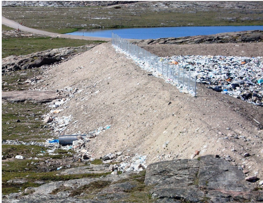
Photograph 2: Waste Disposal Area Earth Berm and Fence
