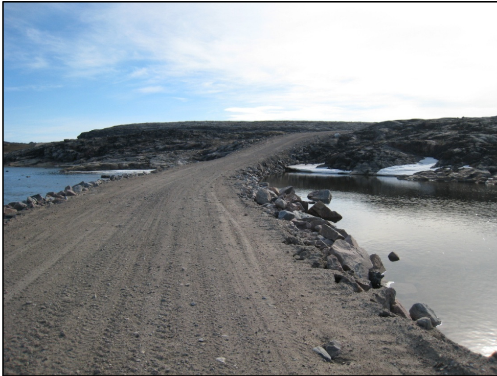
Photo 1 West aspect of constructed CRS-1 crossing at Km 0 of the North Pole River access road, marine Tariuraq Inlet on the left side of photo and the freshwater lake on the right side; no culverts installed.
