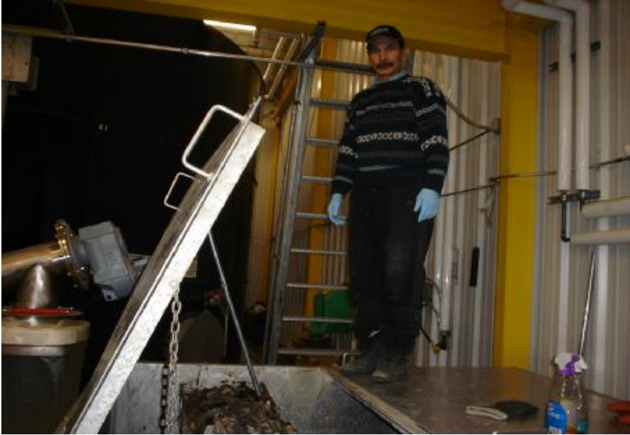
Photo 3. Billy is removing solid waste from bar rack influent chamber.
