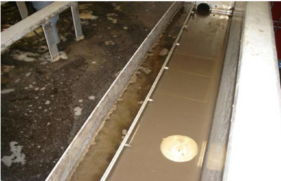
Photo 7. Clarifier – overflow suspended solid to effluent.
