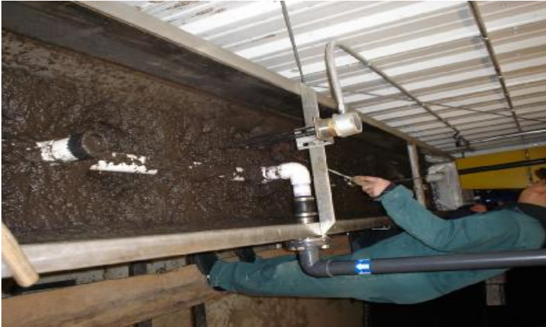
Photo 5. Checking sludge flow and distributing to bags
