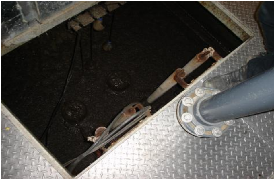
Photo 7. Screened Sewage Tank
