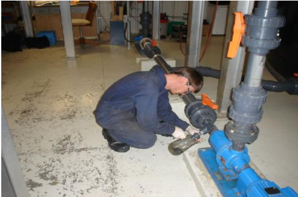
Photo 1. Biological Process Feed Pumps, (Taking sample from EQ Tank)
