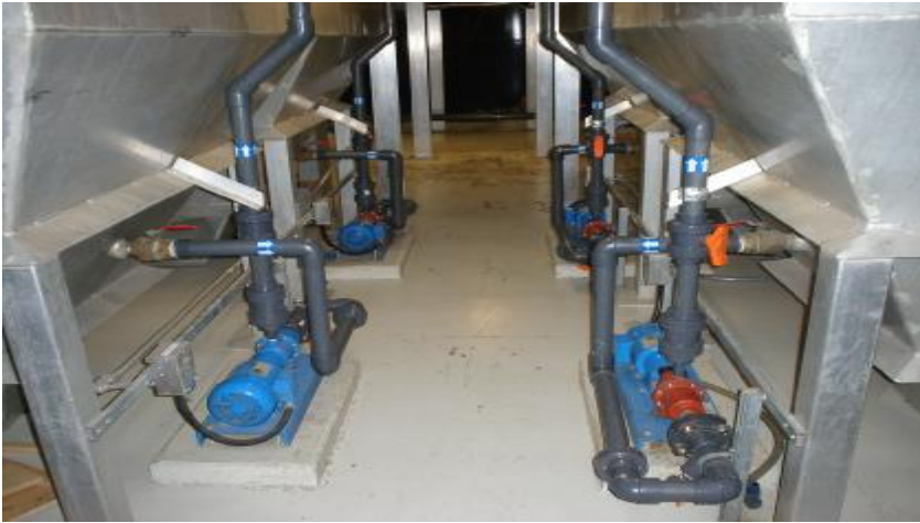
Photo 2. Sludge Digester with decant piping
