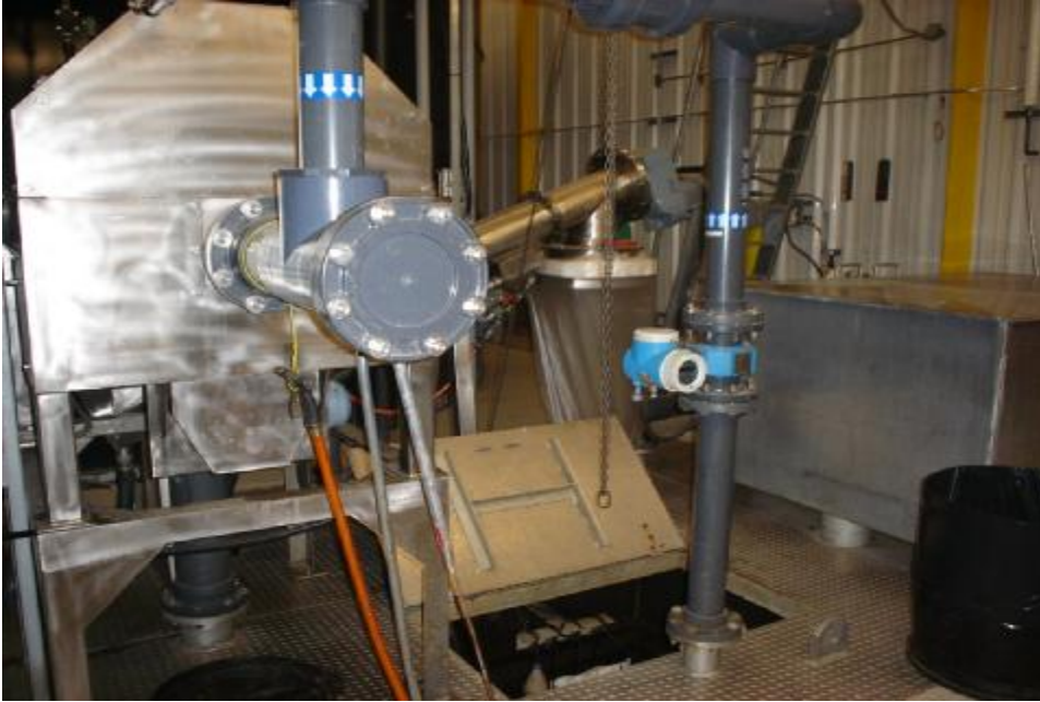
Photo 5. Rotary screen, compactor/conveyor and screenings bagger.
