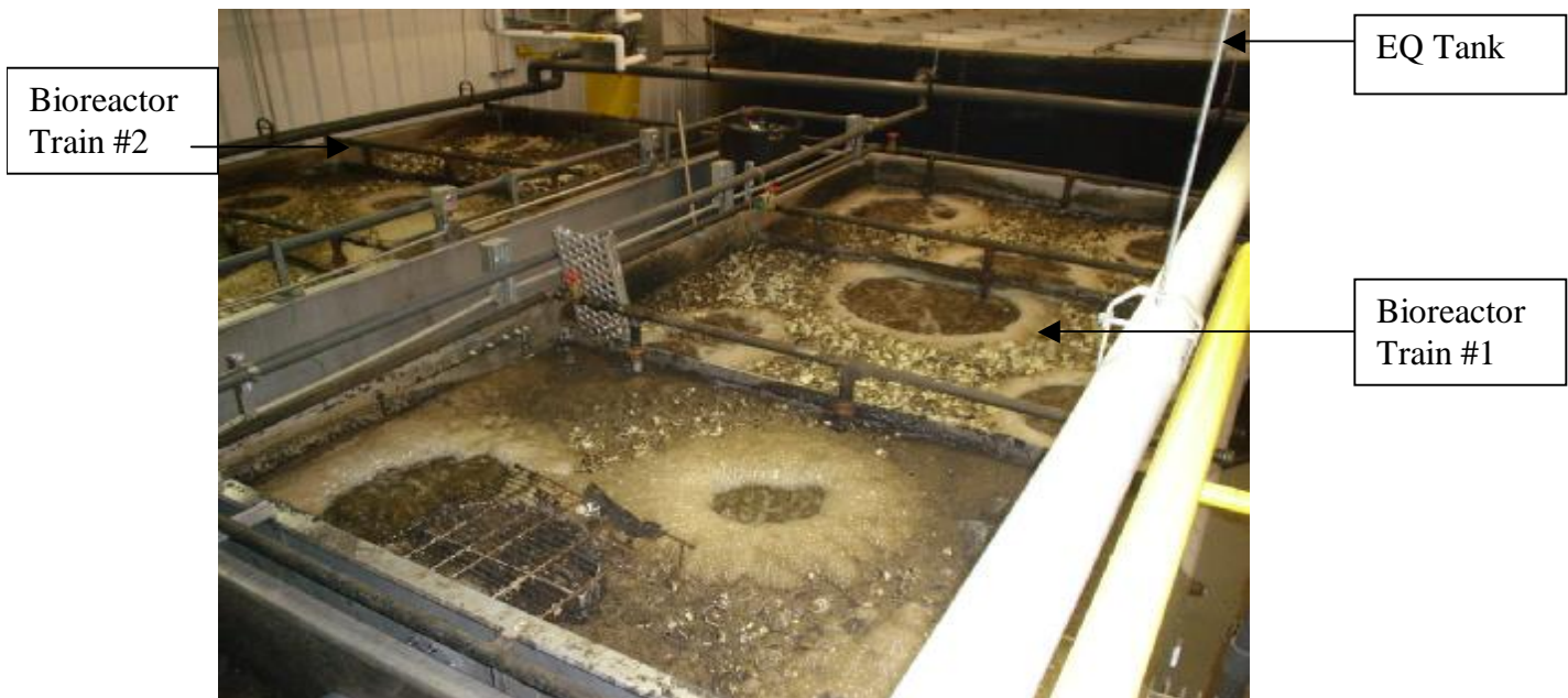
Photo 2. Activated Sludge Reactors. (Jan. 2007)
