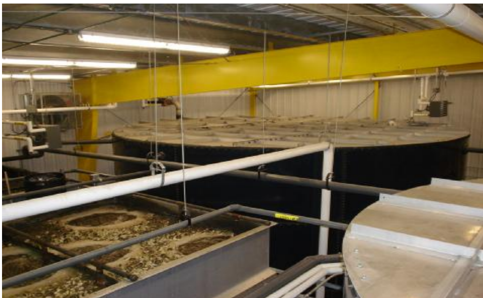
Photo 8. Equalization Tank
