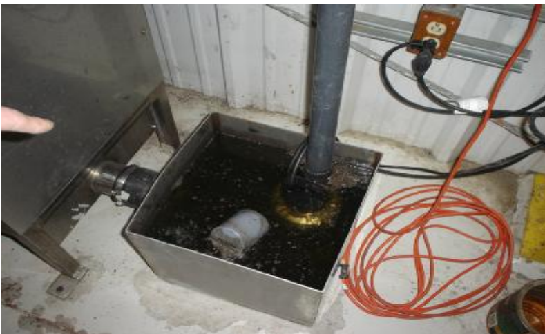
Photo 6. Filtrate return pump
