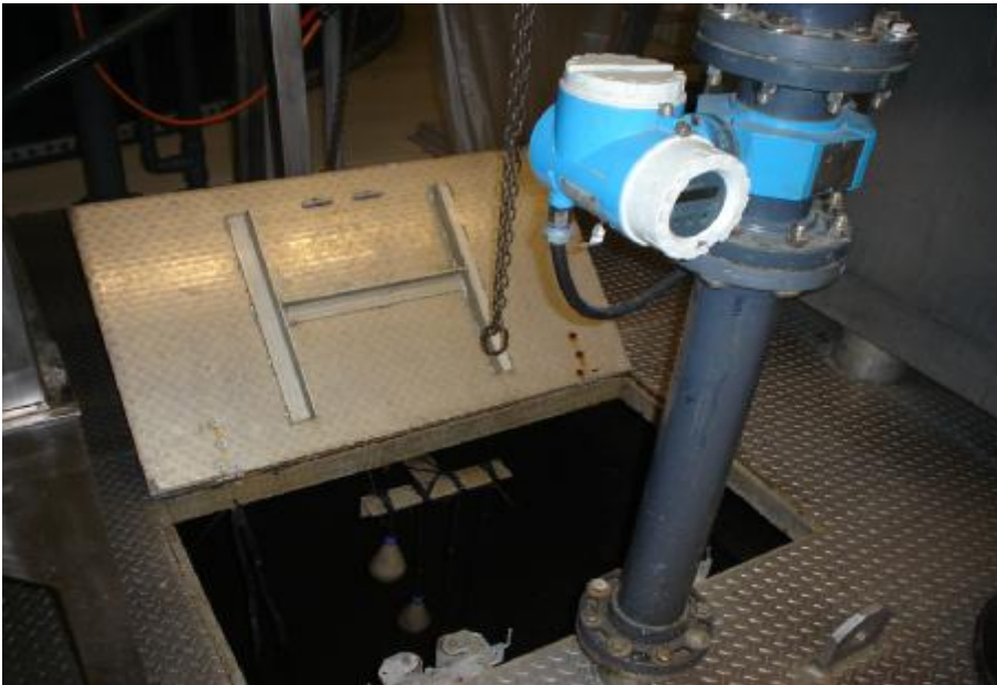
Photo 4. Receiving tank and influent flow meter.
