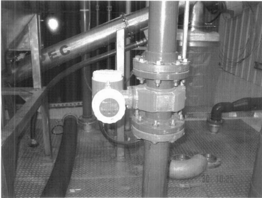
Photo 11. Flow metre on Sewage System out flow.
