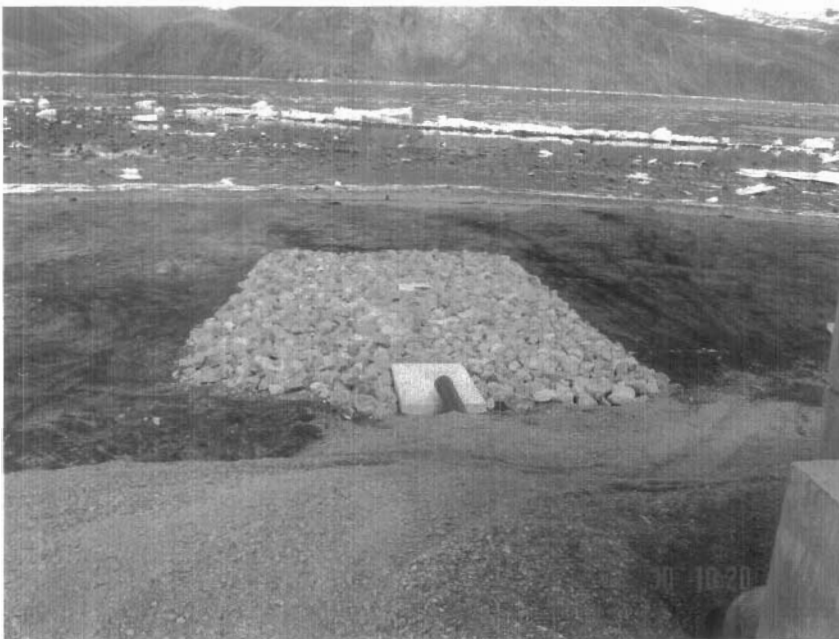
Photo 12. Sewage Facility discharge structure.
