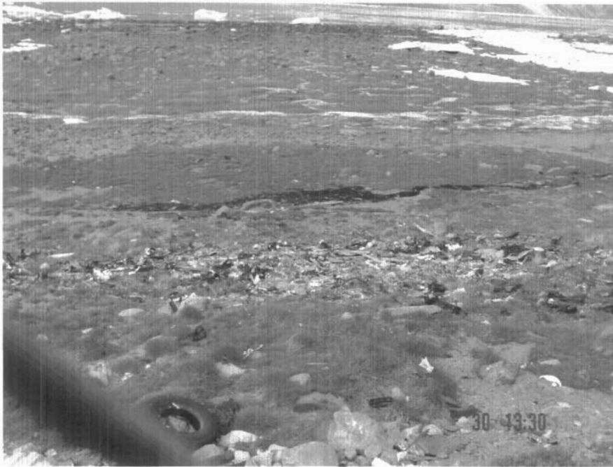
Photo 21. Solid Waste Disposal Facility seepage path and refuge at back of dump.
