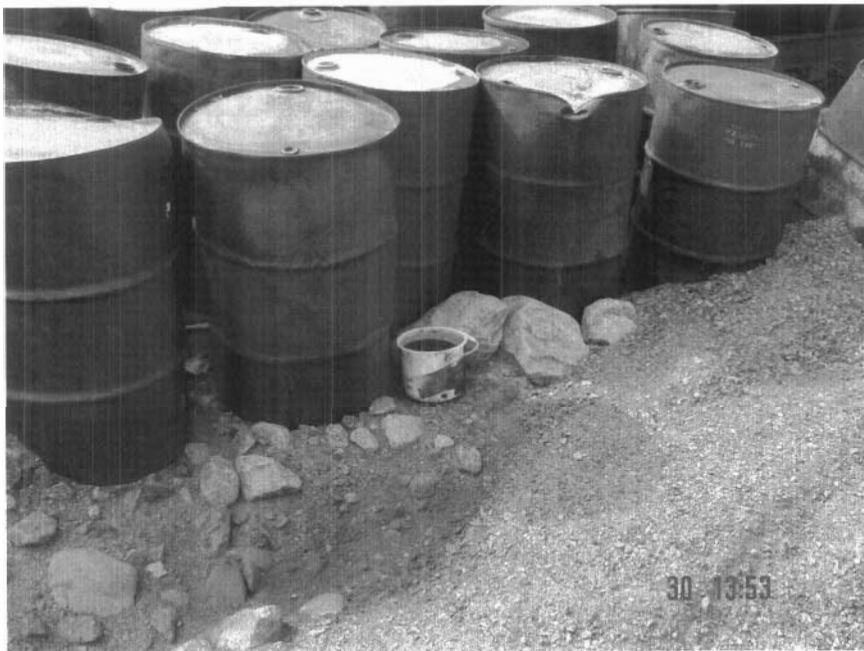
Photo 24. Waste oil storage in improper containers.
