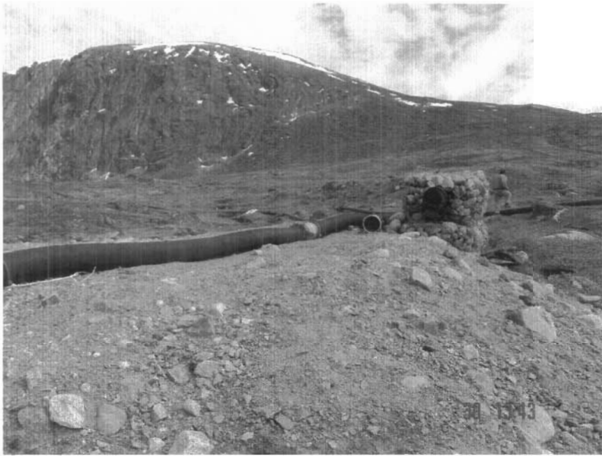
Photo 3. Water Reservoir recharge line.
