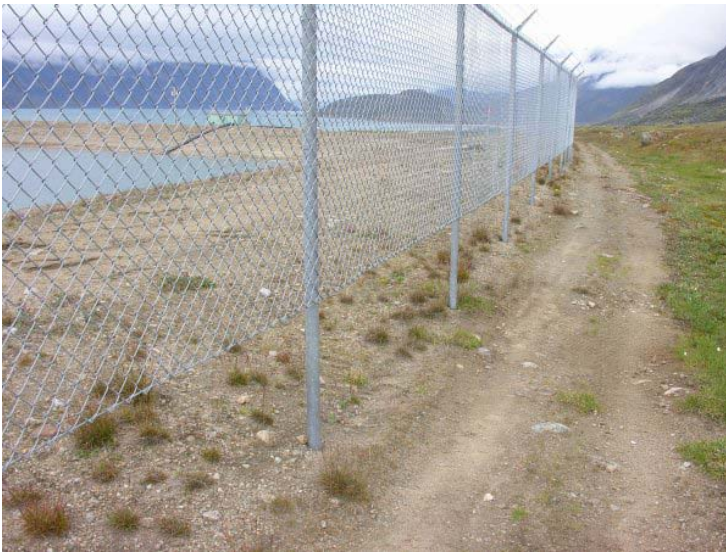
View of fence around reservoir, not extending to ground level.
