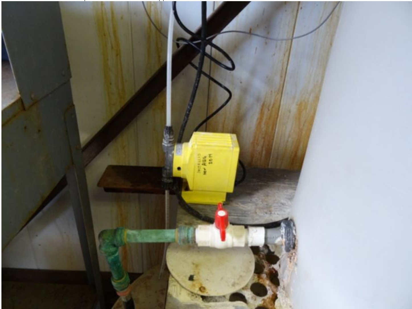
Figure 6 Chlorination pump
