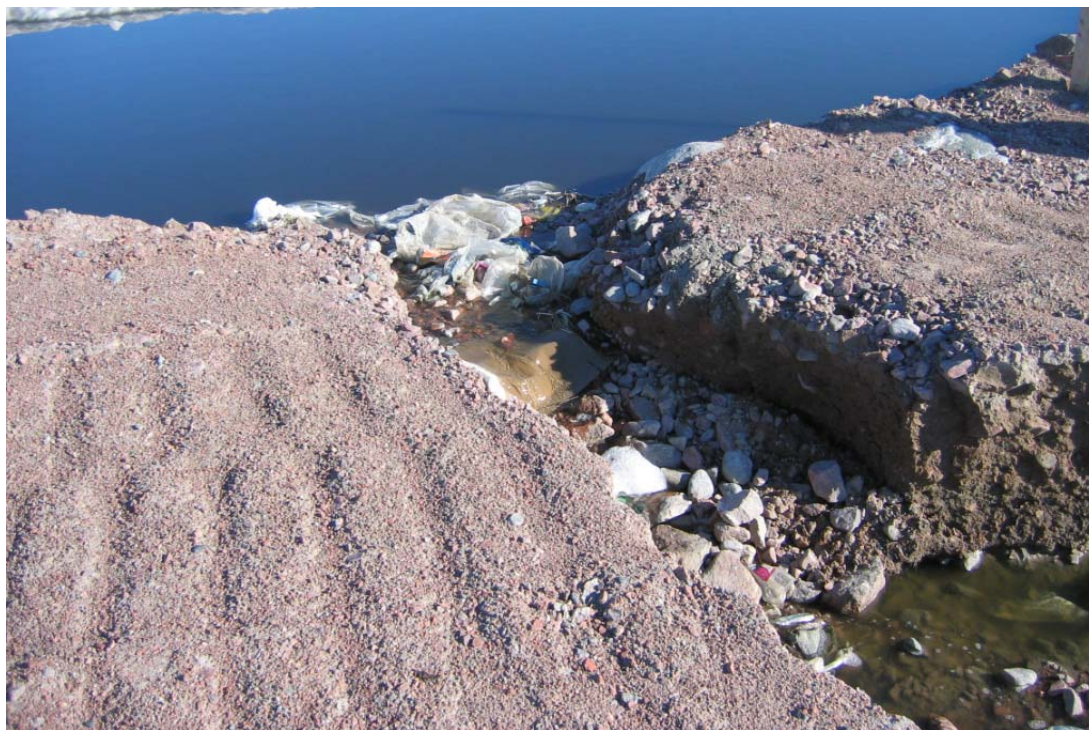
Plate 2: View looking west at existing downstream lagoon. Note breach in dyke
