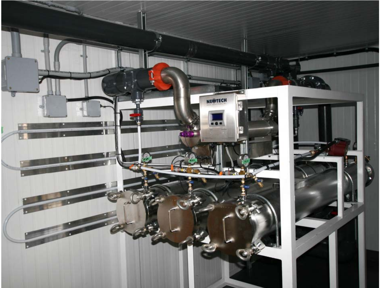
Fig. 1 - Cartridge filter housings and UV module.
