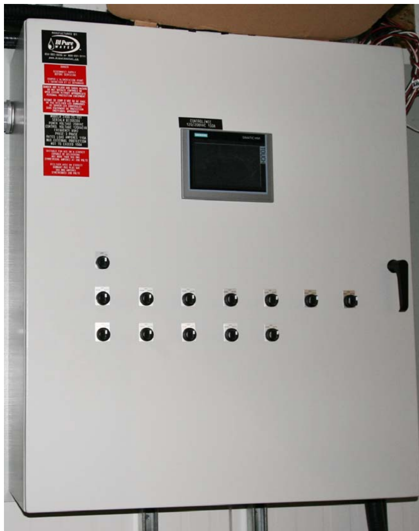
Fig. 3 – Control panel with HMI and switches
