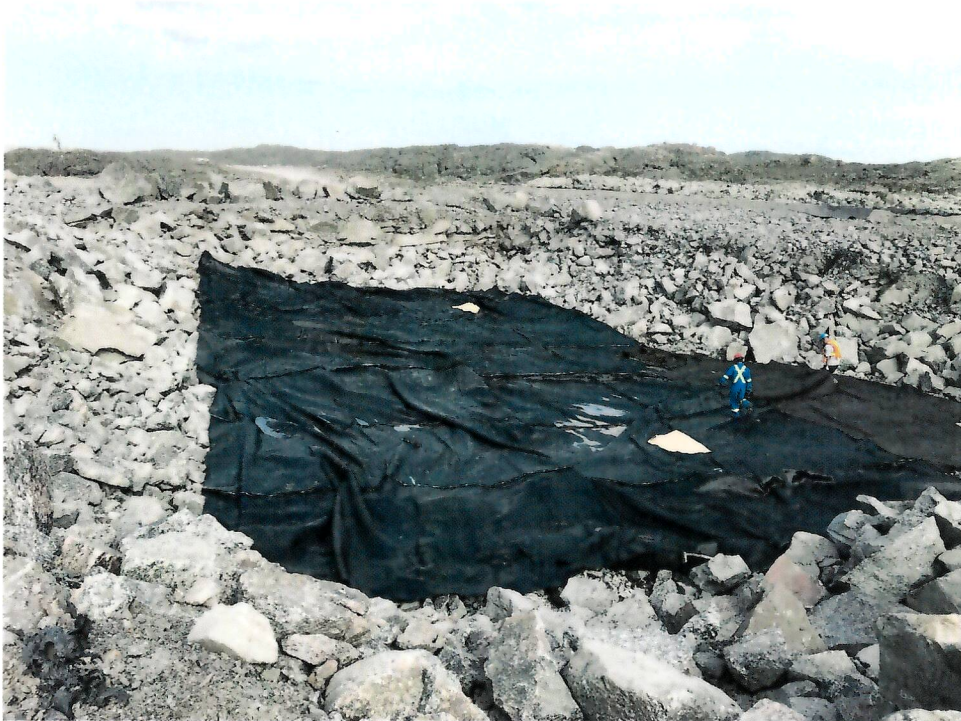
FIGURE 3: GEOTEXTILE IN BALSTED HOLE
