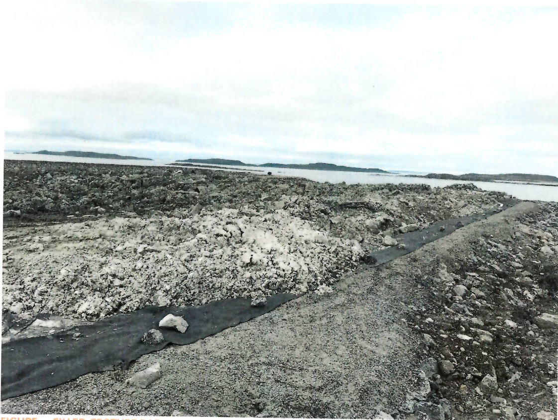
FIGURE FILLED GEOTUBE PAD
