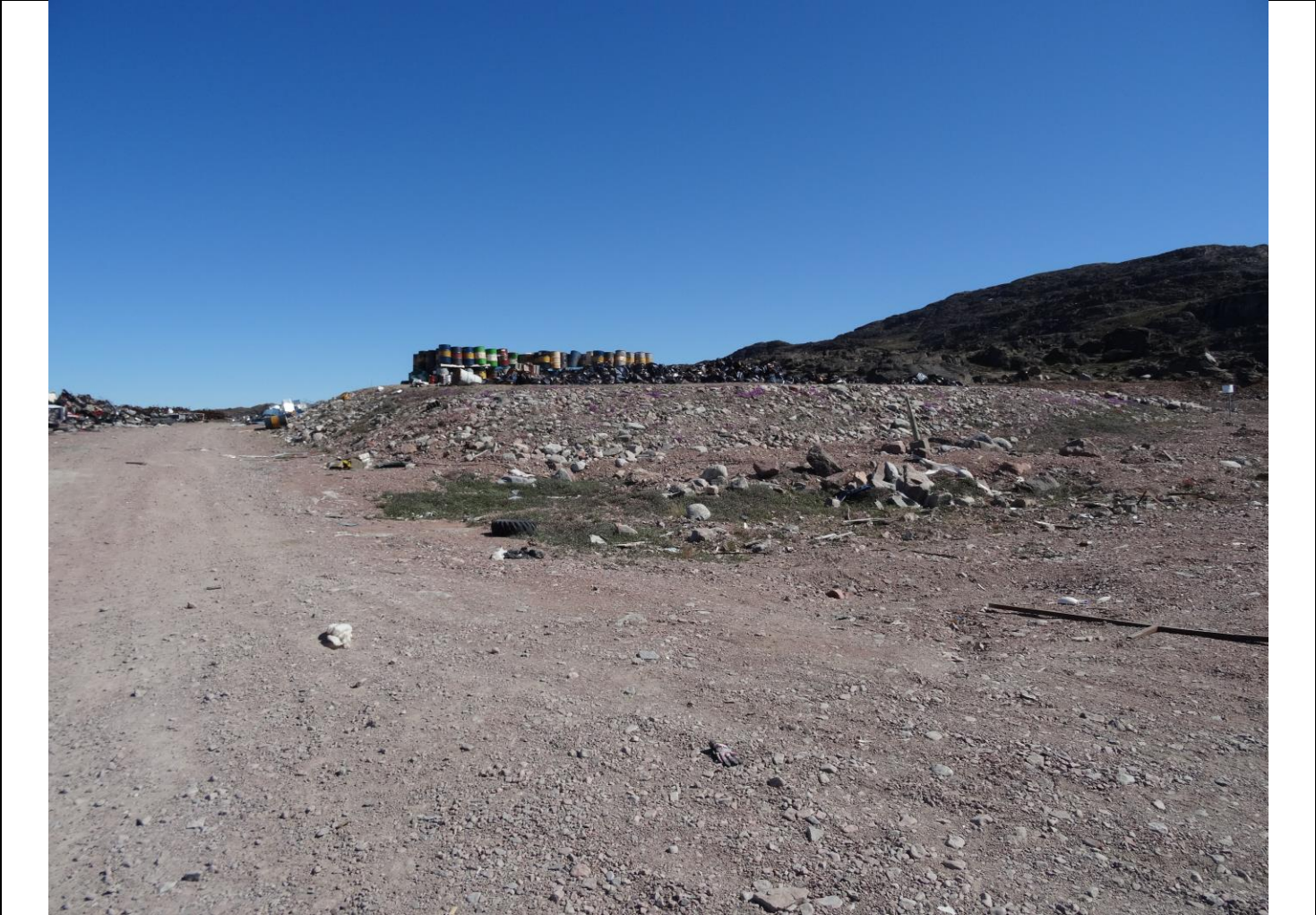
Description: 3 Bermed Cells in the Metal Dump containing Used Oil Drums in 1 Cell and Washed Crushed Drums in the other 2 Cells
