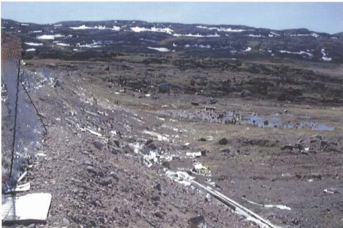
figure 5. Leachate runoff from the solid waste disposal facility; 2001/07/06.
