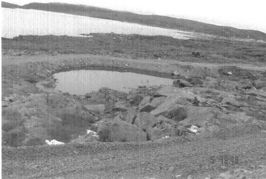
Photo 15. New berm and road at back of sewage lagoon.
