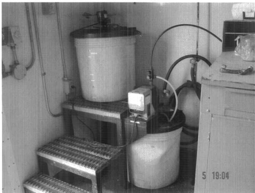
Photo 4. Chlorination system at Water Intake Facility.
