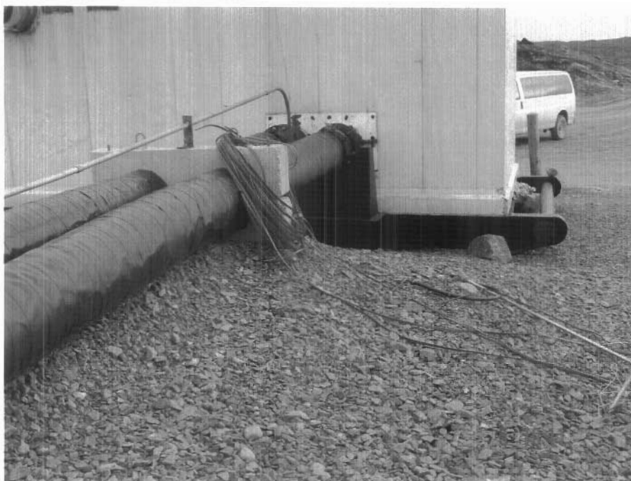
Photo 5. Old conveyance line heat trace.
