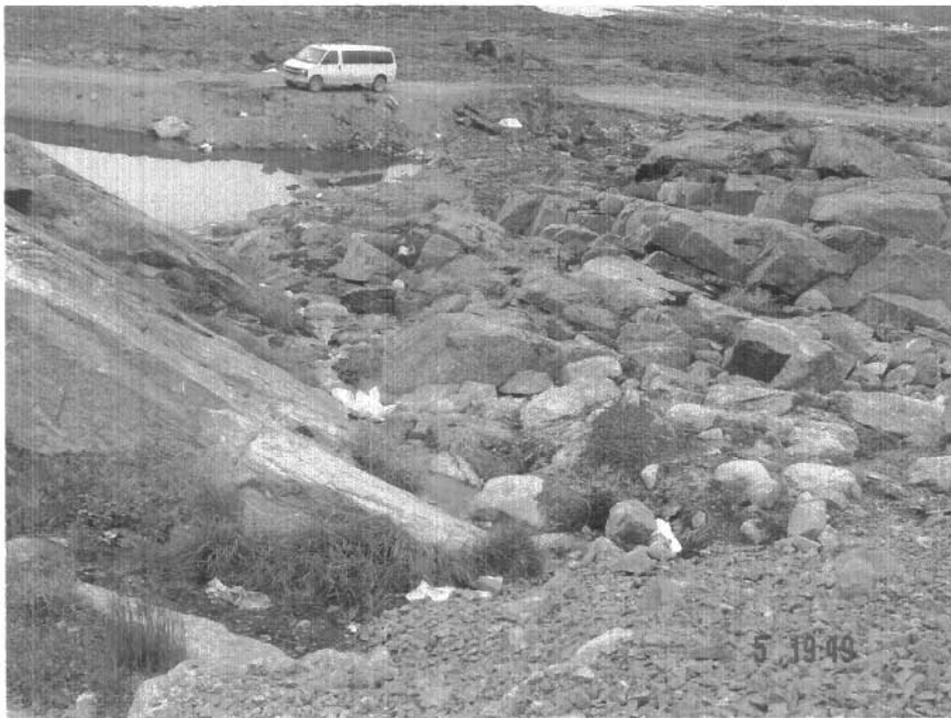
Photo 16. Seepage emitting from back of sewage lagoon.
