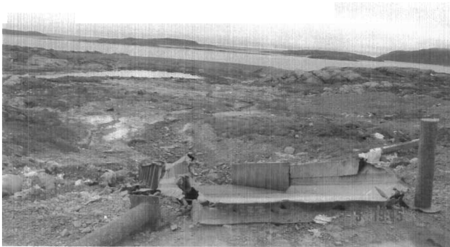
Photo 13. Sewage truck discharge structure at sewage lagoon.
