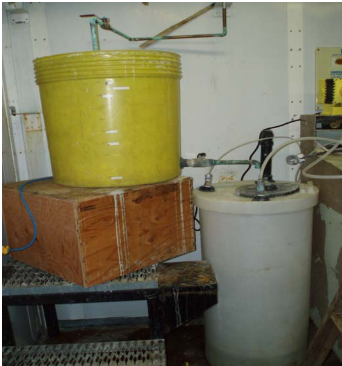
Picture 2. Chlorine being added to the tanks before it gets distributed to the community.
