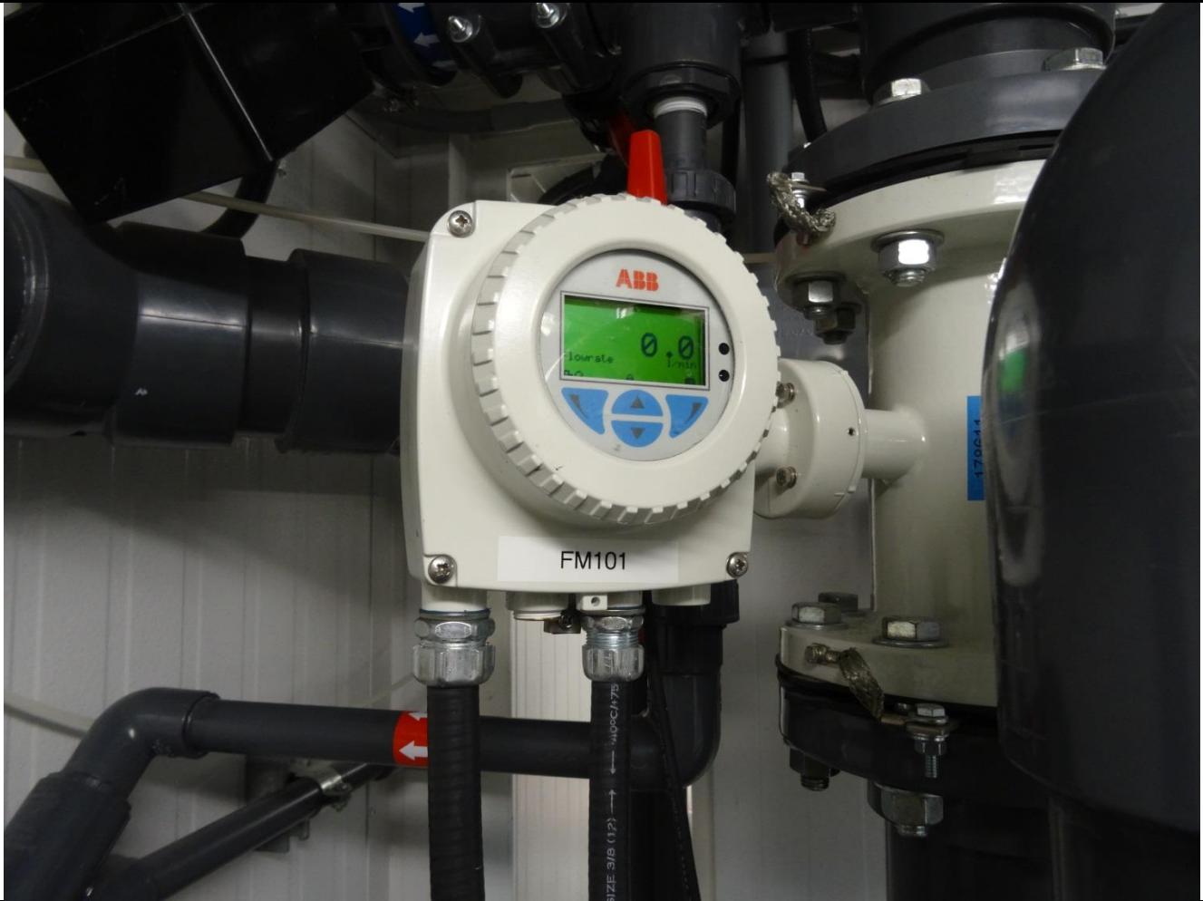
Description: Flow Meter on Raw Water Intake
