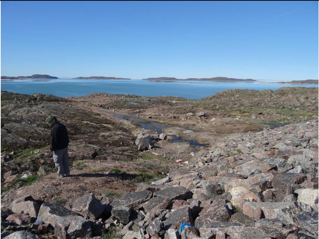
Description: Sewage Lagoon – Leak #1 in Berm flowing toward ocean
