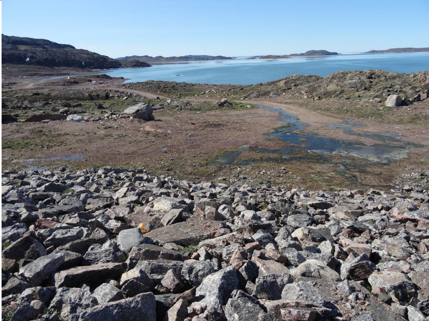
Description: Sewage Lagoon – Leak #2 in Berm flowing toward ocean
