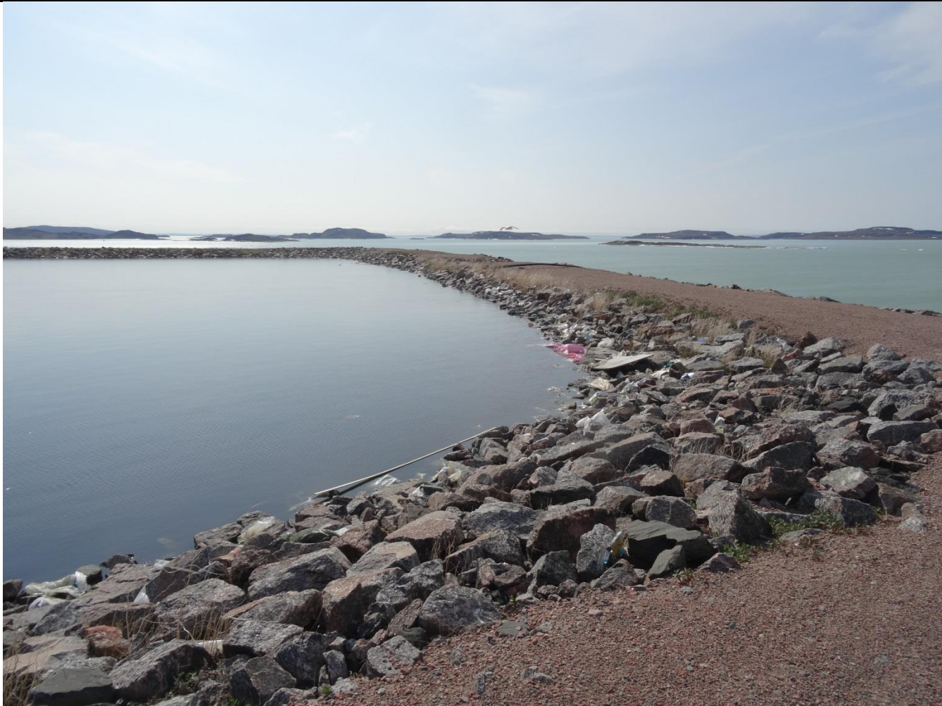
Description: Sewage Lagoon showing High Levels requiring Decanting
