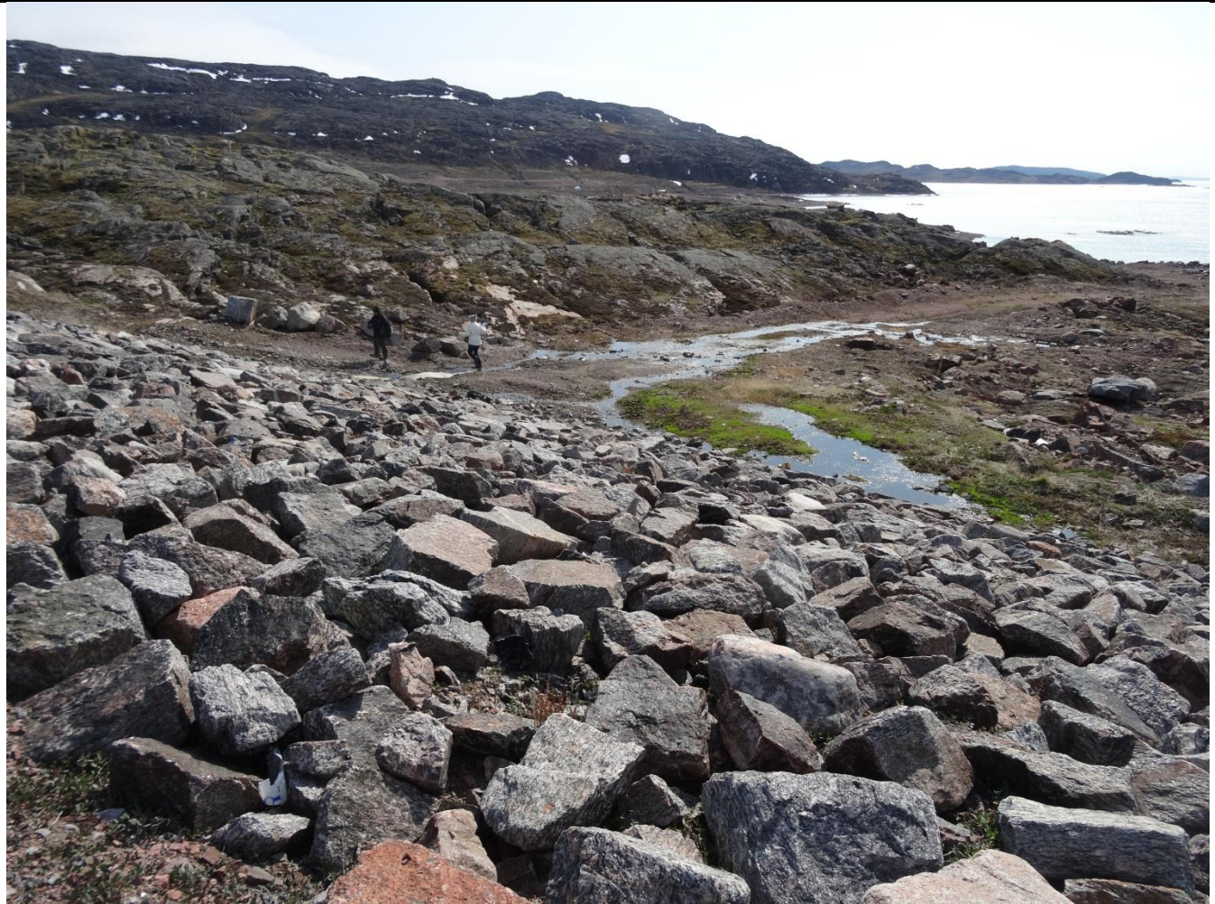
Description: View of Sewage Lagoon Leak #1 from top of Berm
