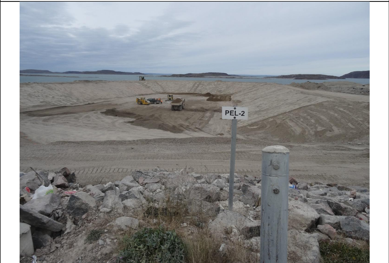
Description: Contractor Rebuilding the Sewage Lagoon which is expected to be in use before freeze-up this season
