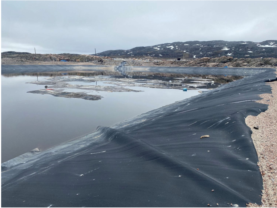
2023 Liner Bubbles - West Side
