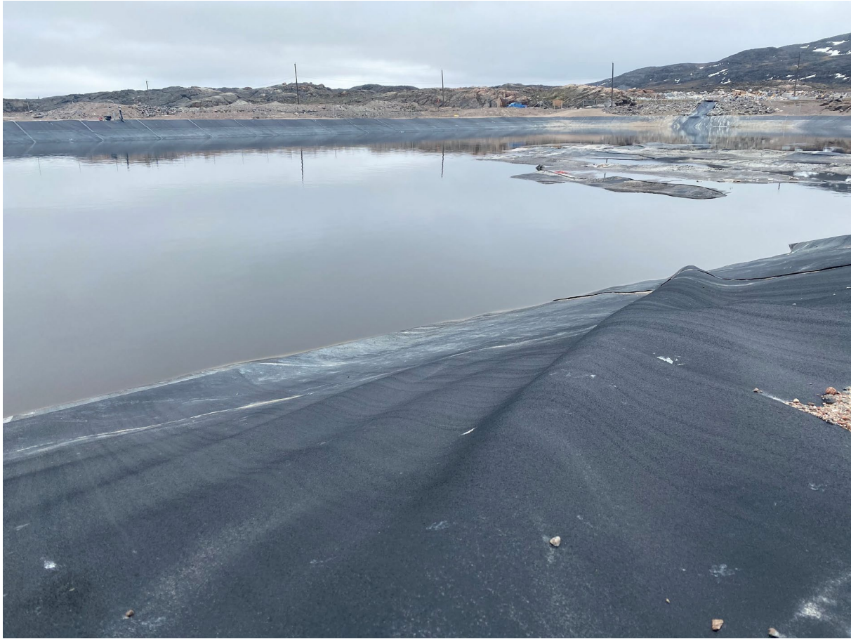
2023 Liner bubbles- west side of the lagoon
