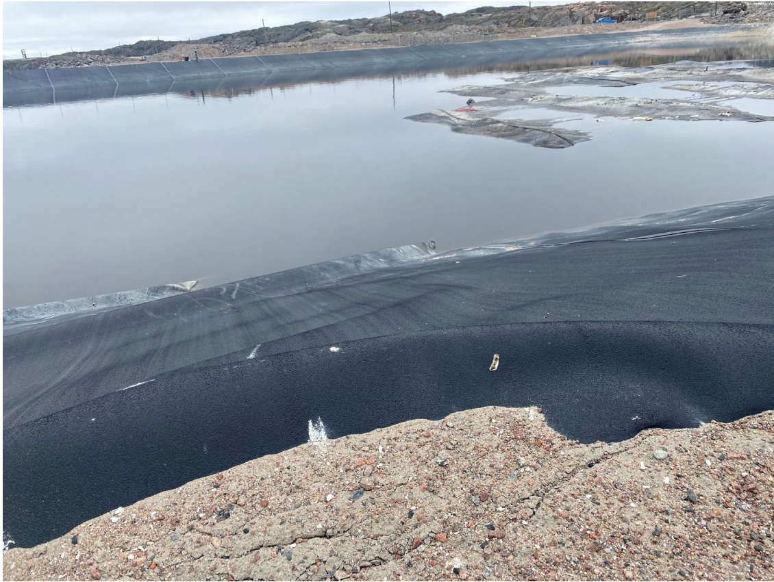
2023 Liner Bubbles - West Side
