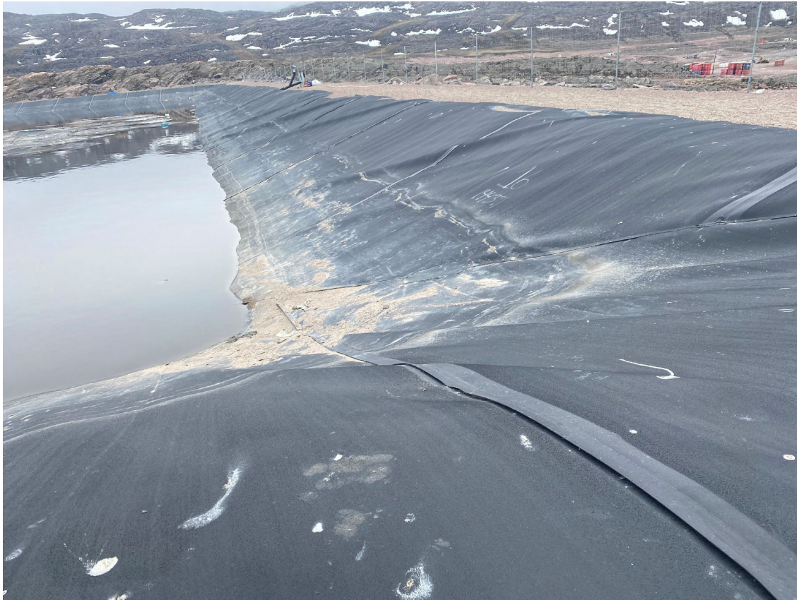
2023 Liner Bubbles - West Side
