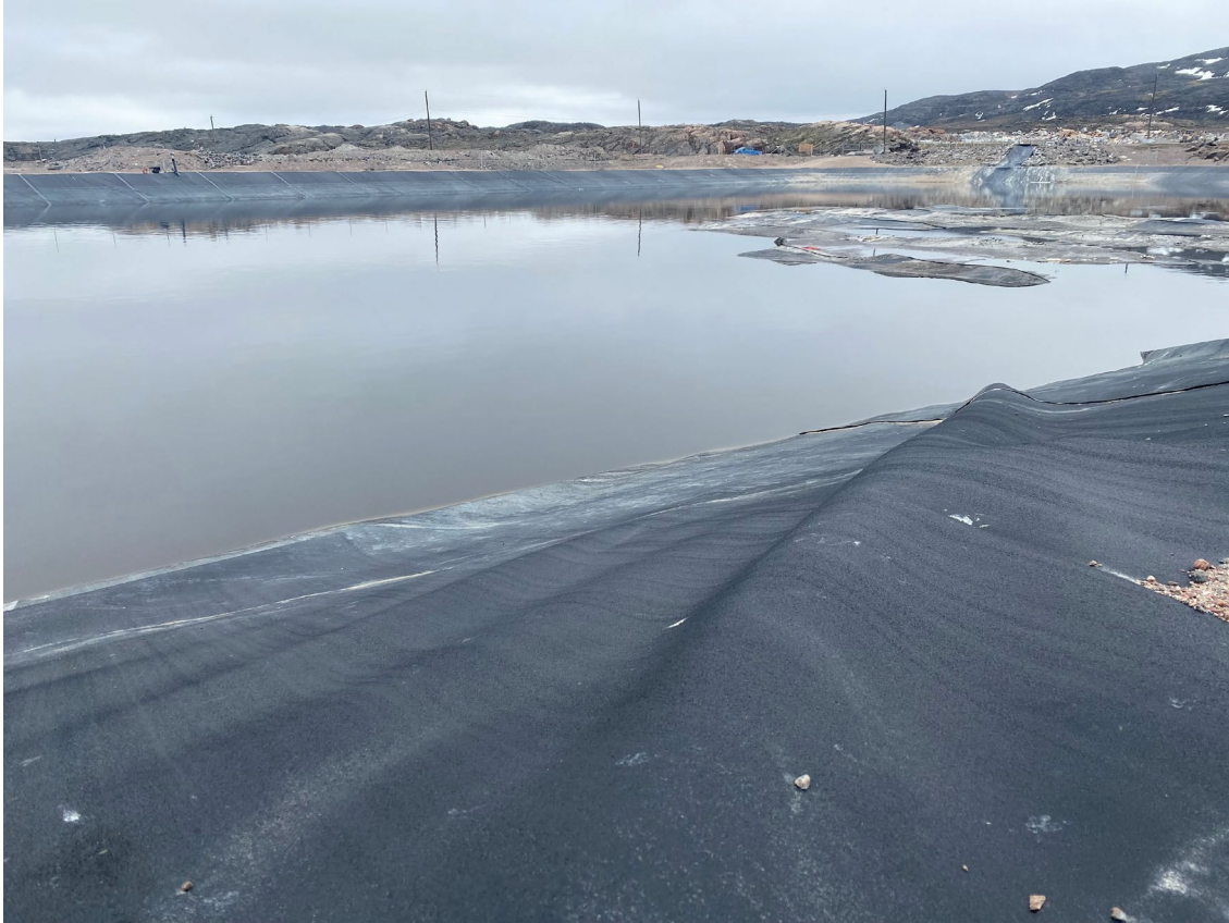
2023 Liner Bubbles - West Side
