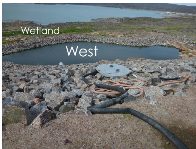
Discharge control manhole on west side flowing onto flow dispersion berm structure
