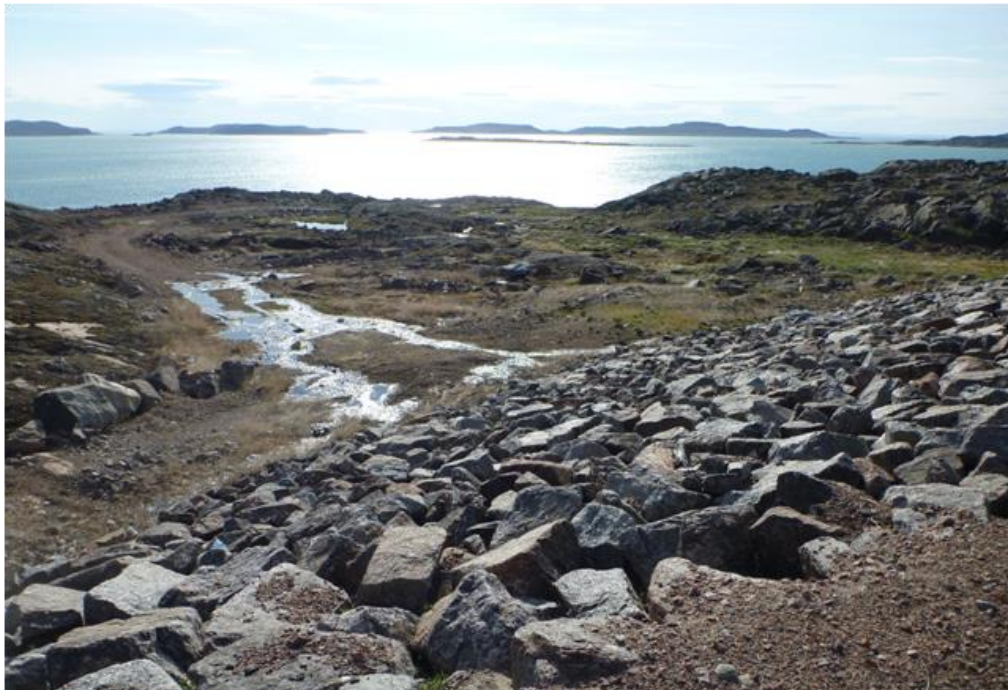
Figure 3: Seepage from south perimeter berm, Kugaaruk waste water lagoon
