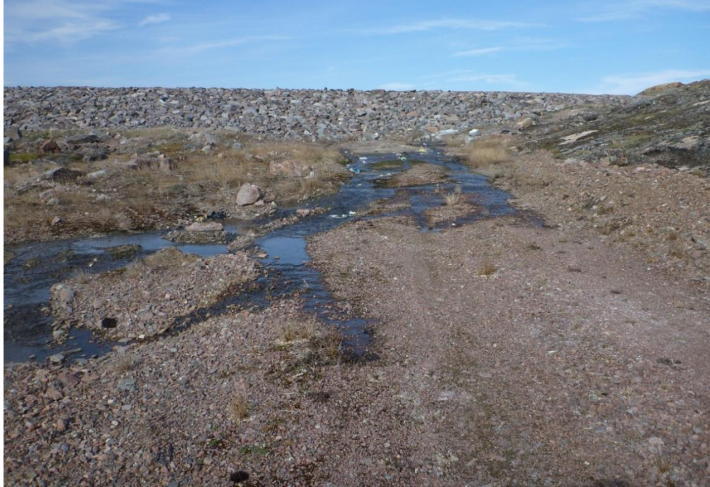
Figure 2: Seepage from south perimeter berm, Kugaaruk waste water lagoon
